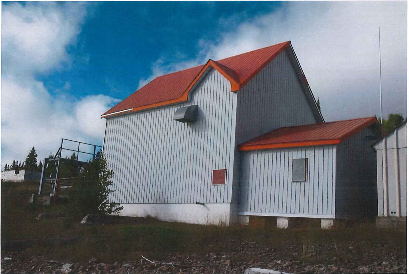
Generator Building & Annex. Metal cladding in good condition, several fascia pieces missing.
