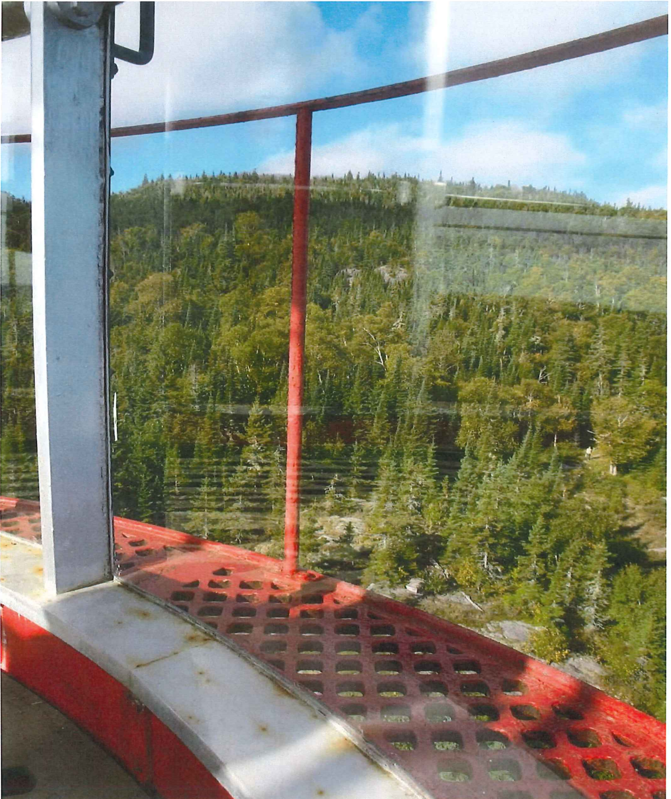
Exterior platform: Open-grate cast-iron with steel pipe railing. Local corrosion.
