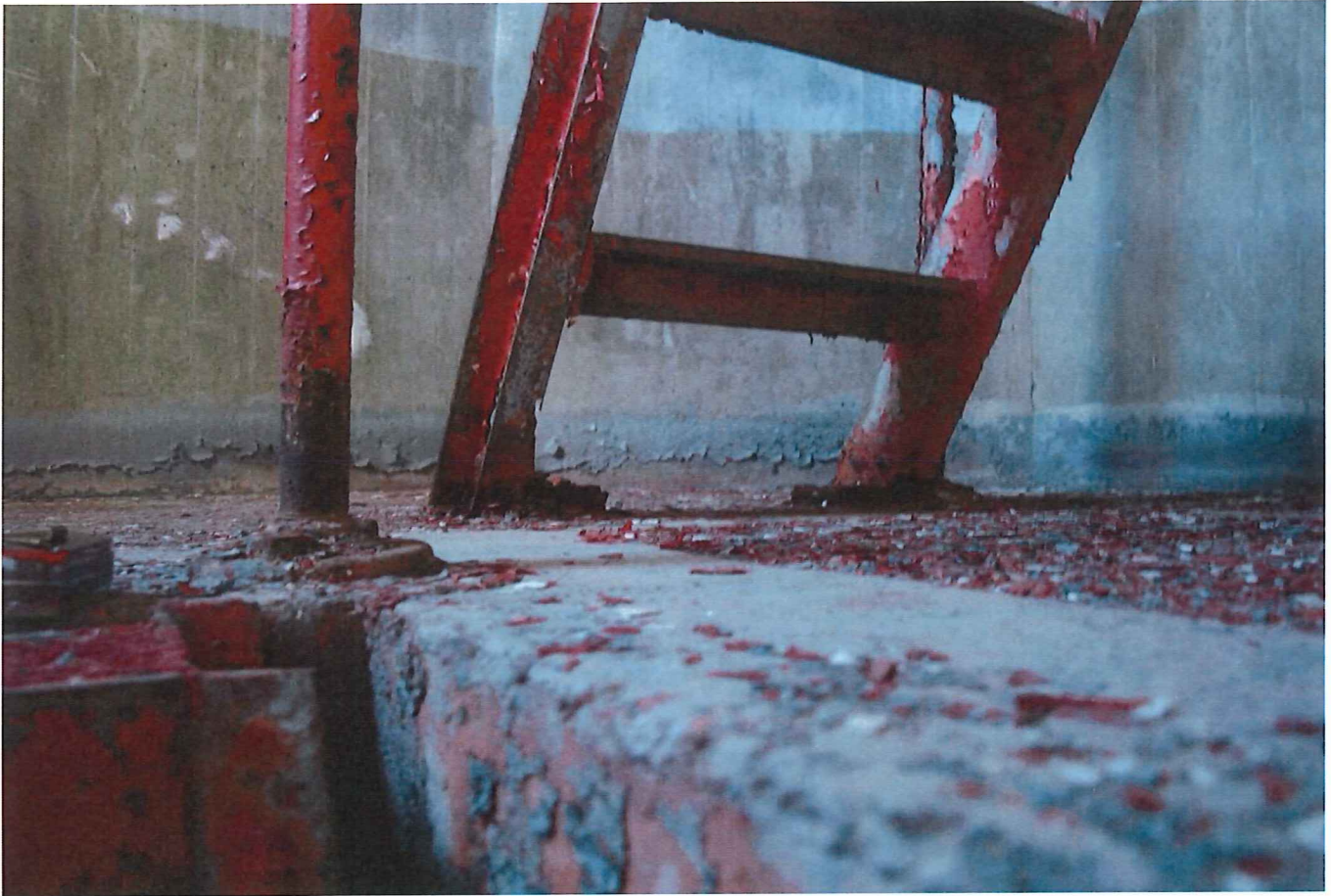
Typical condition of ladders and railings at supports. Peeling paint, local corrosion.
