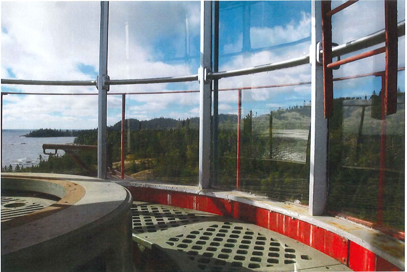
Lantern room: Metal-plate wall, open-grate cast iron upper floor. Condition generally satisfactory.
