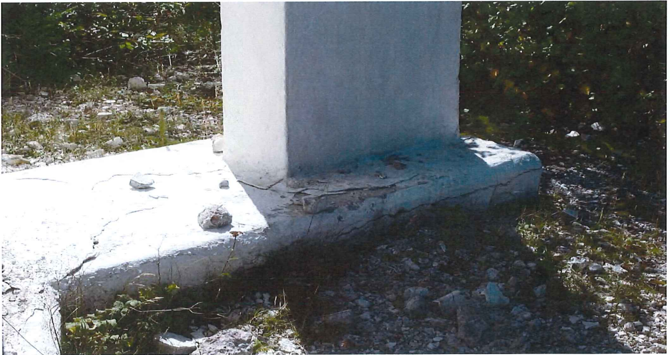
Concrete cracking and spalling at base of buttress.
