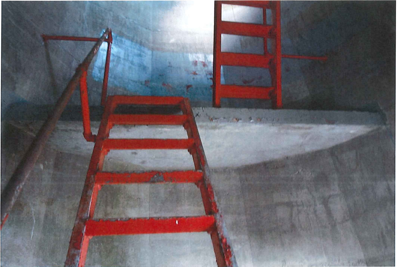
Typical ladders, pipe railings, concrete landing. Note walls generally in good condition.
