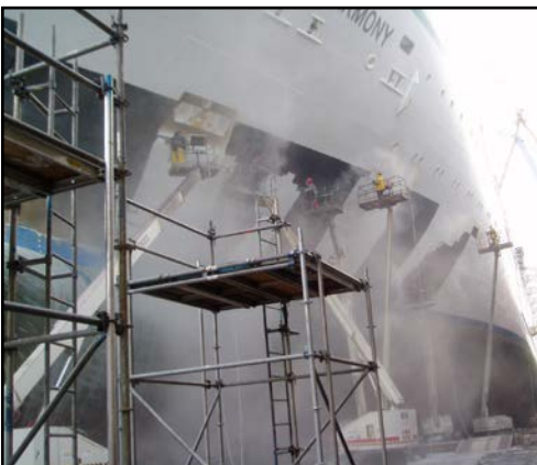
The hull of a cruise ship being ultra high pressure washed.
