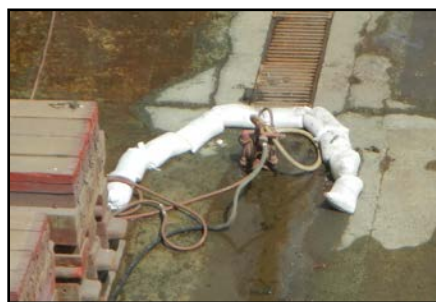
Sand bags used on dock bottom to divert and filter excess water.
