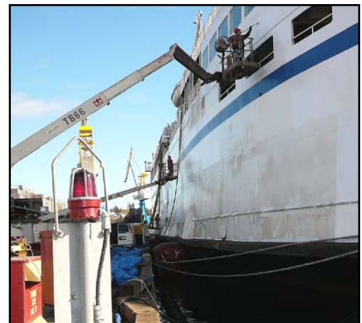
While painting vessels docked alongside the wharves or jetties, do not spray paint. Take sufficient measures to prevent paint from entering the marine environment.
