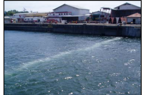
Bubble curtain employed during vessel transfer.
