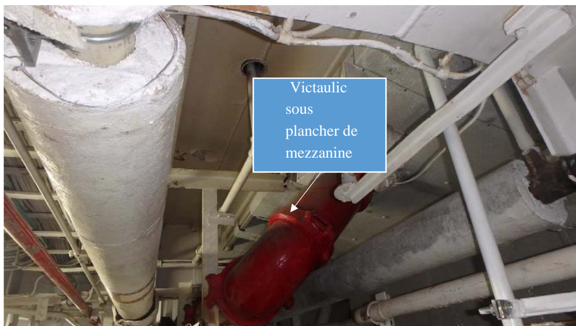
Photo no. 26; tuyau 200mm sous plancher mezzanine
