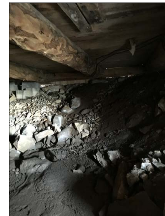
PHOTO 1: POUTRES EXISTANTES, DIMENSIONS VARIANT DE 230@305mm (9"@12")
