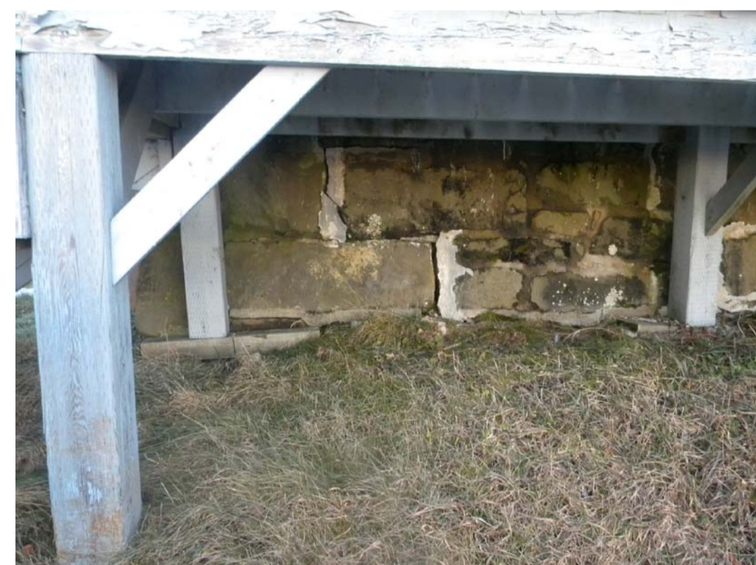
PHOTO 7 - PIERRES DE COIN EXISTANTES
