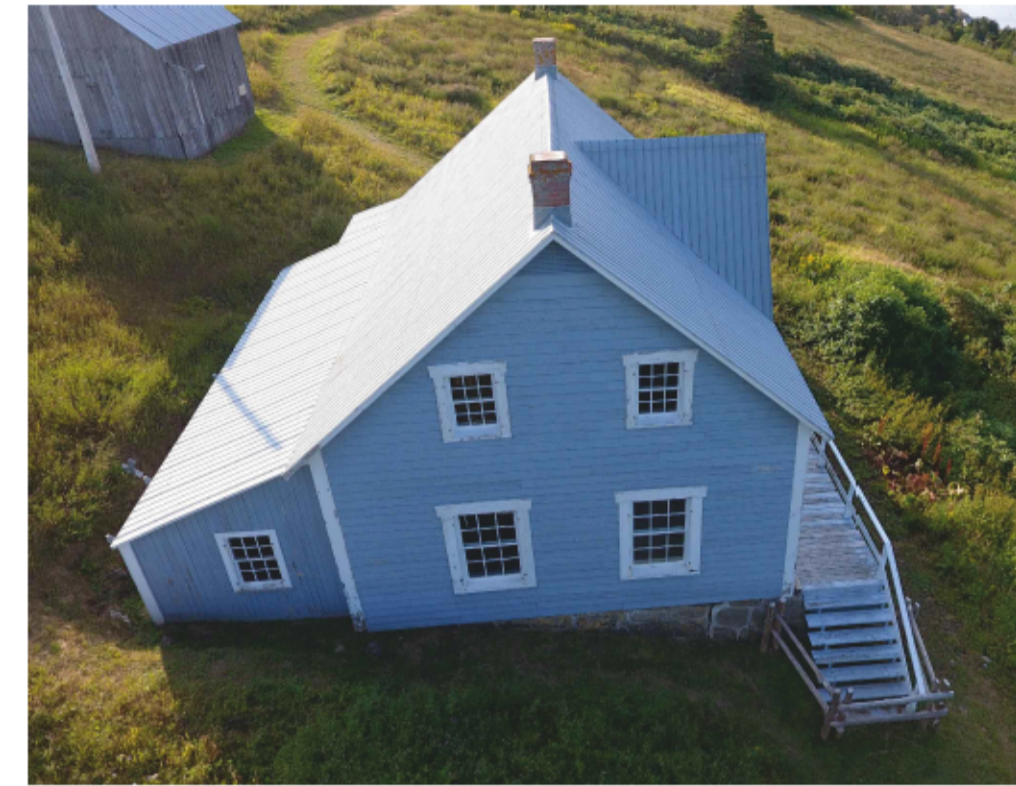
EXISTING LEFT ELEVATION - PHOTO
