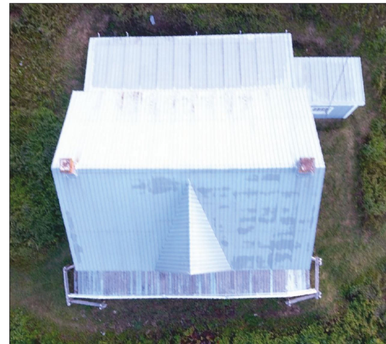
PICTURE 1 - EXISTING ROOF VIEW
