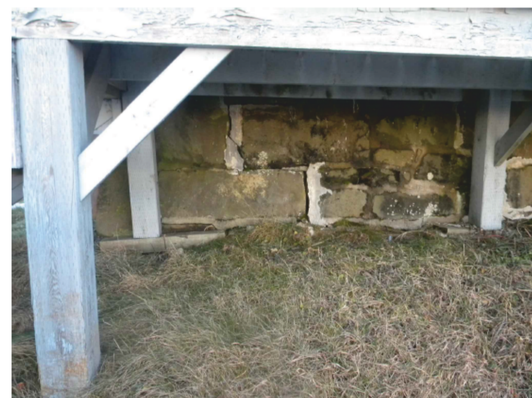
PHOTO 7 - EXISTING CORNER STONES
