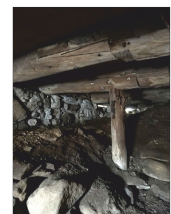
PICTURE 2: SUPPORT OF EXISTING BEAM
