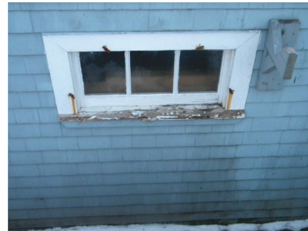
PHOTO 4 - EXISTING WINDOW SILL
