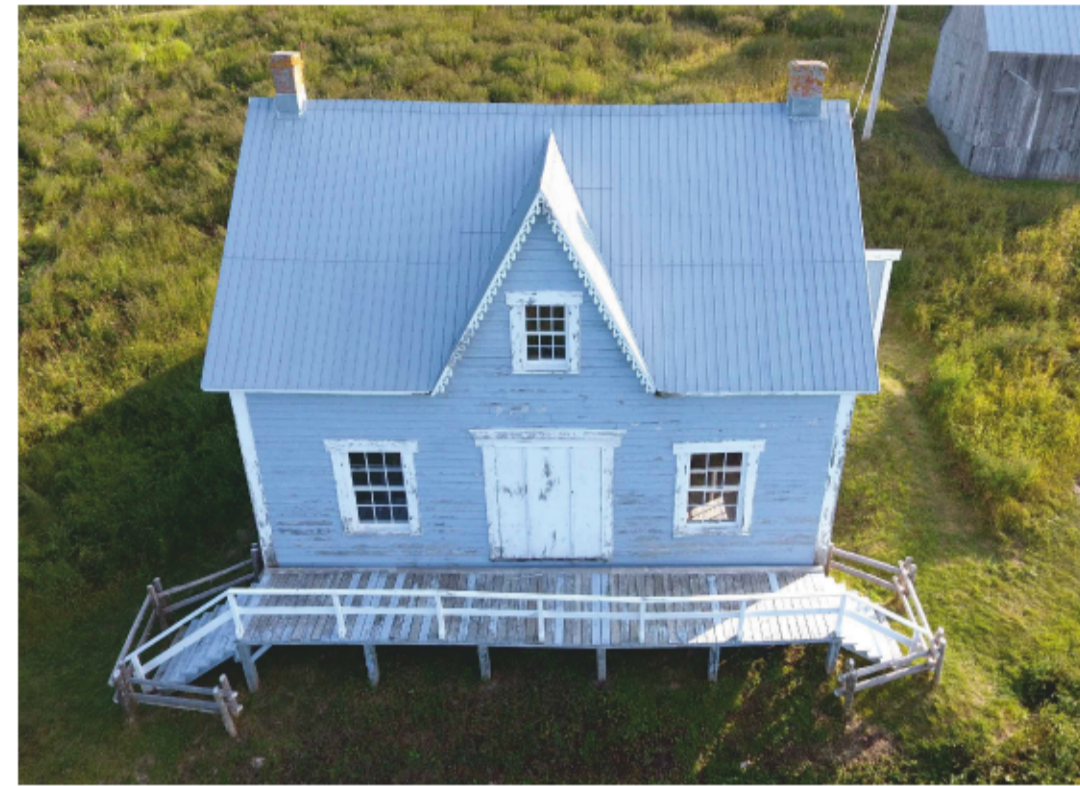
EXISTING FRONT ELEVATION - PHOTO
