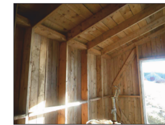
WALLS AND CEILING OF THE ANNEX EXISTING
