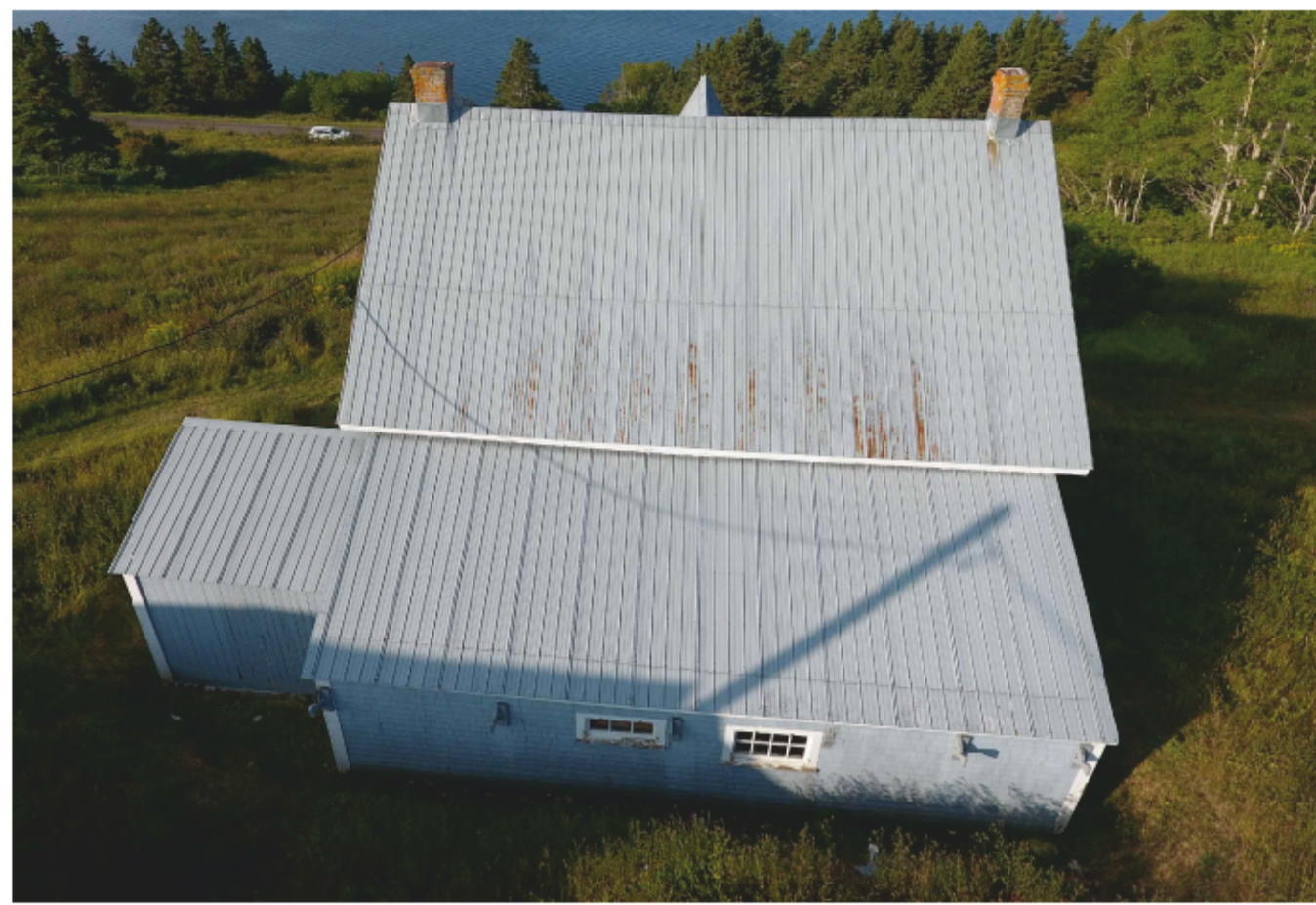
EXISTING BACK ELEVATION - PHOTO
