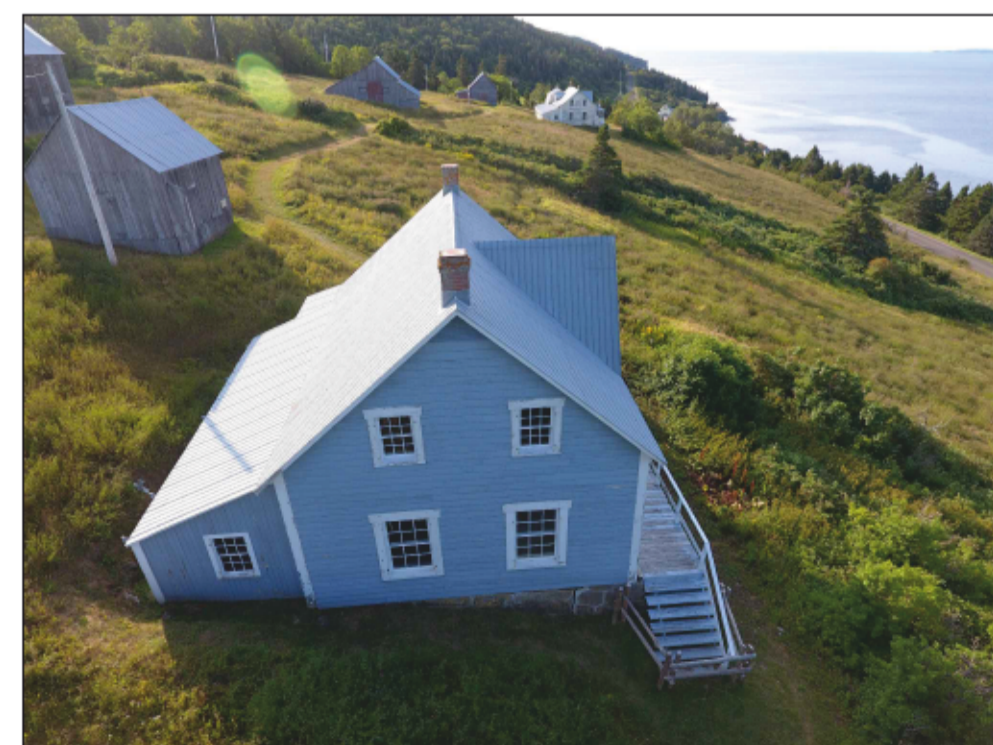
PICTURE 6 - EXISTING GROUND SLOPE VIEW
