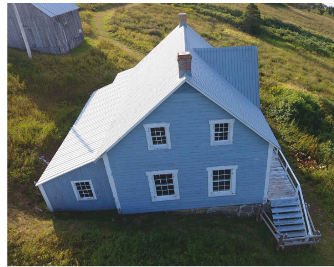
EXISTING LEFT ELEVATION - PHOTO
