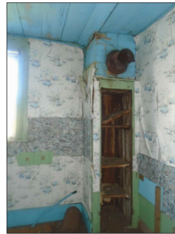
EXISTING CHIMNEY FIRST FLOOR
