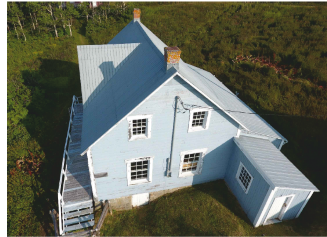
EXISTING RIGHT ELEVATION - PHOTO
