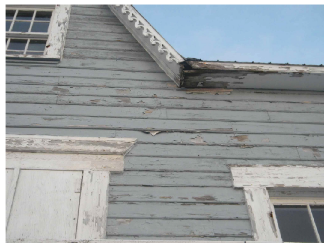
PHOTO 5 - EXISTING FRONT FASCIA AND SOFFIT
