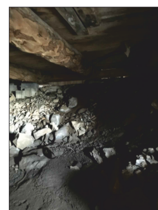
PICTURE 1: EXISTING BEAMS, DIMENSIONS FROM 230 @ 305mm (9" @ 12")
