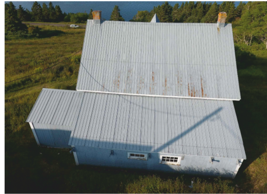
EXISTING BACK ELEVATION - PHOTO
