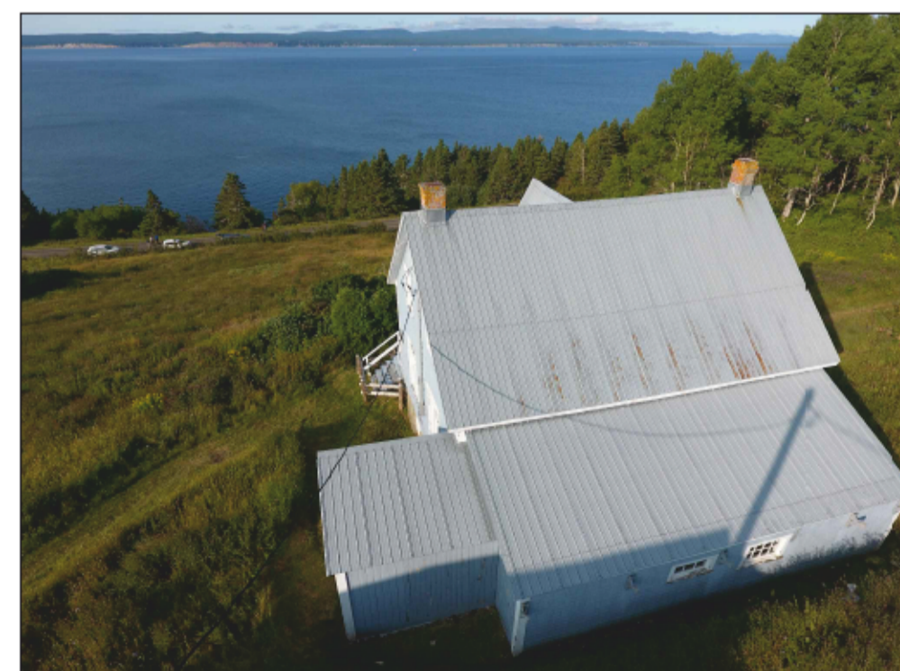
PICTURE 5 - EXISTING GROUND SLOPE VIEW
