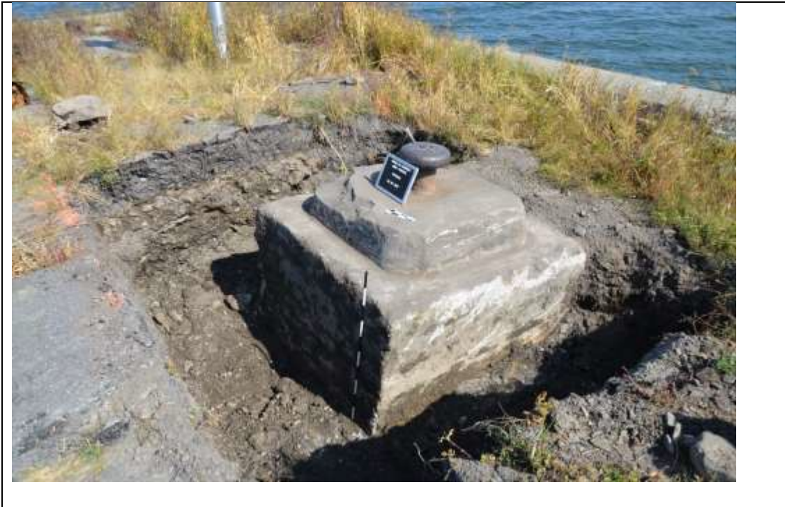
Figure 7 – Bollard and its concrete base two layers deep (510G13A101) located at the northeast end of the Federal Wharf (Photo Matthieu Paradis, Parks Canada).
