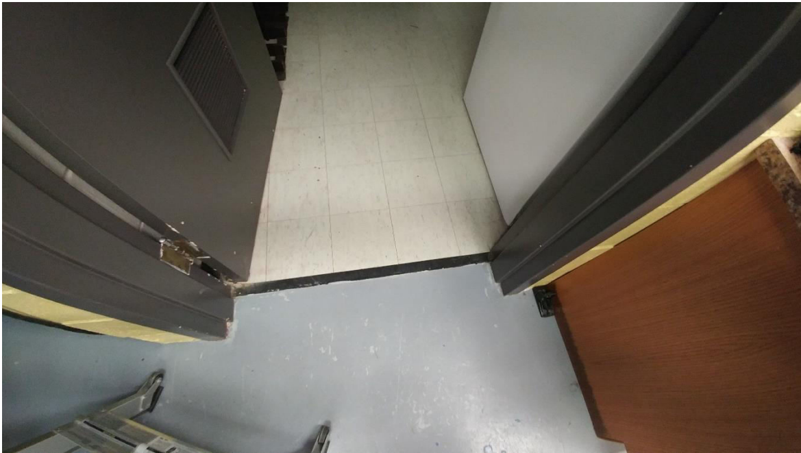
Photo 3: Previously confirmed 9" vinyl floor tile. This material was generally in good condition.
