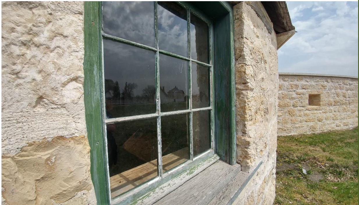
Photo 1: Lead containing green trim on the bakehouse
