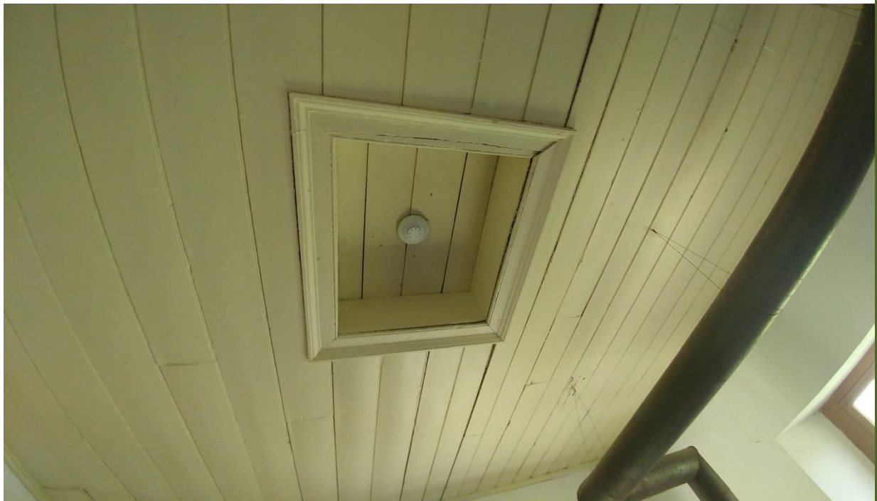
Photo 2: Heat sensor fixed to the attic hatch in the Ross Cottage. Attic area was not examined as a result.
