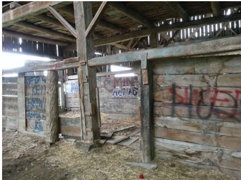
Photo 12: Interior view of large barn.
