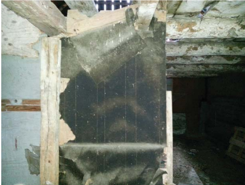
Photo 7: View of representative tar paper located in Building 3.
