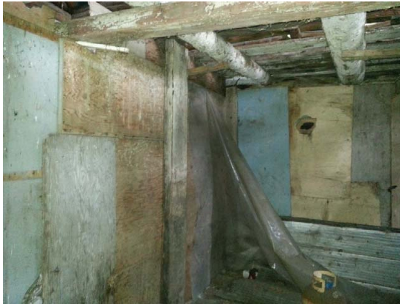
Photo 9: View of lead containing grey wall paint located in Building 3.
