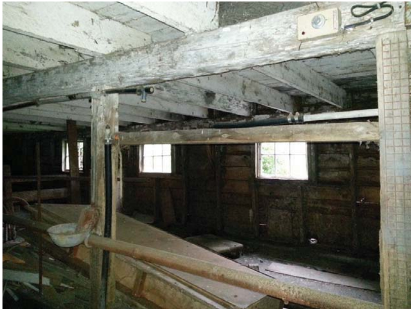
Photo 13: Interior view of stable.
