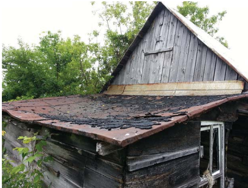
Photo 2: View of representative asphalt shingles collected from Building 1.
