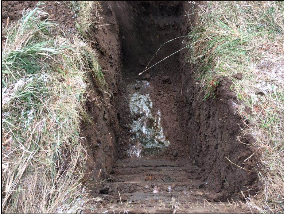
Photo 1: Test hole TP 1, showing bedrock surface at approximately 1.9 m depth.
