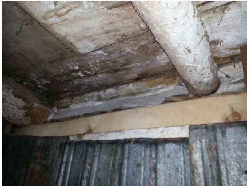
Photo 8: View of representative mortar located in Building 3.
