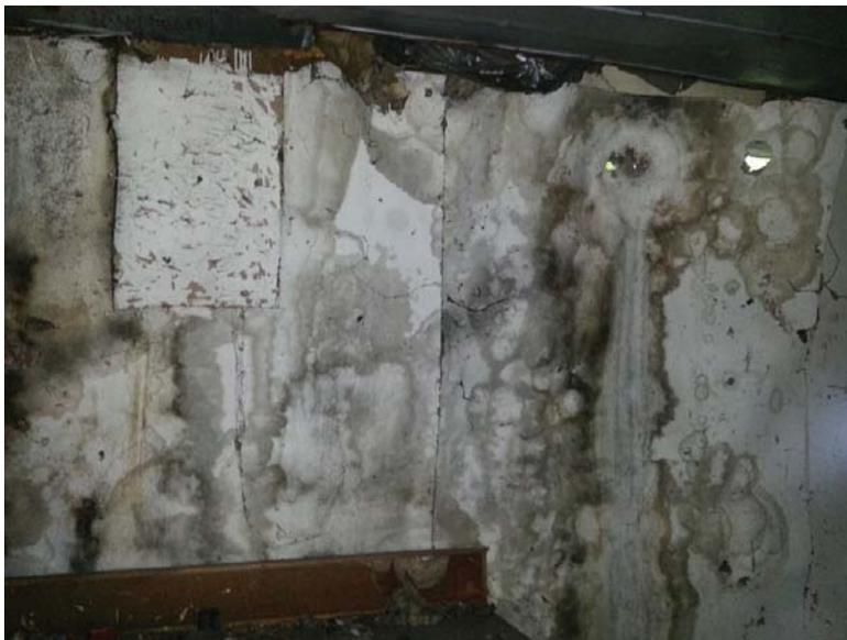
**Photo 3:** View of water damage and suspected mould growth in Building 1.
