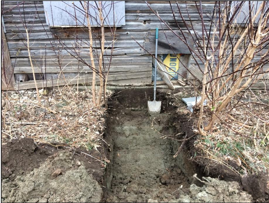
Photo 4: Exterior of Building 'C', showing dry stacked rock wedge foundation.
