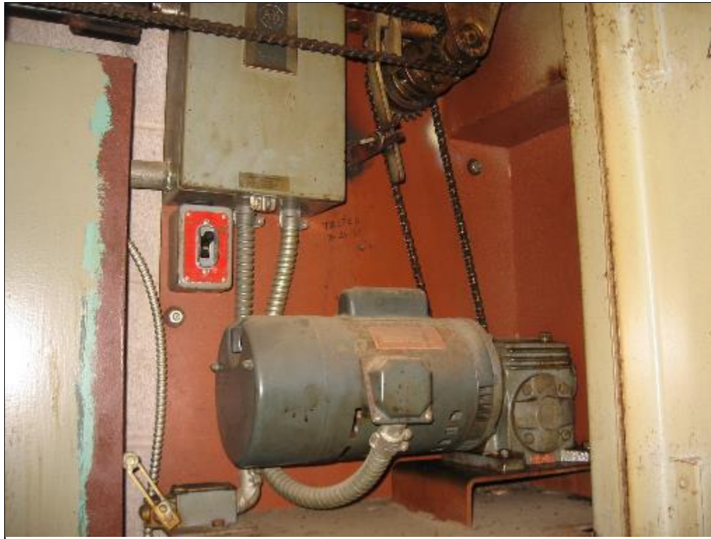
Photo 21: Electric motor in wall cavity off laundry room of each wing containing <1 litre of gear oil for chain-driven riot doors. (8 Sept. 2016)
