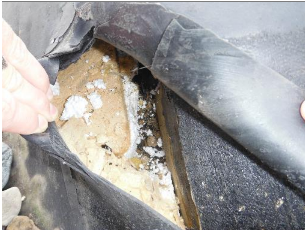
Photo 8: Roof layers. Including rigid foam insulation (all layers non-ACM) (8 Sept. 2016)
