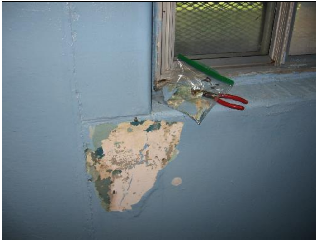
Photo 13: Interior light blue/green/beige flaking paint on wall in Room C8. Sample No. P-1. (7 Sept. 2016)
