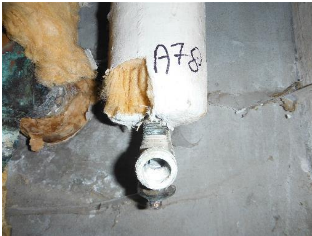
Photo 4: Insulating pipe cement (Sample No. A-78: 30 % Chrysotile asbestos) over fibreglass at end of 12 mm dia. pipe in Lower Mechanical Room. (8 Sept. 2016)
