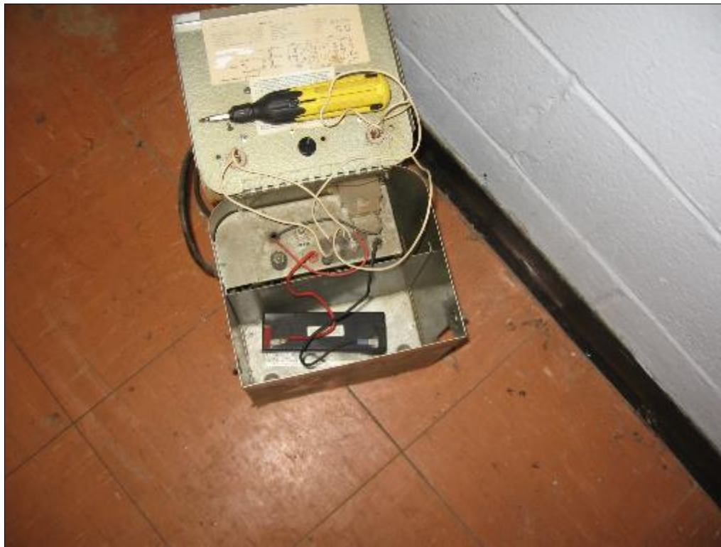
Photo 24: Emergency lighting unit on floor in hallway of main entrance, near Room 104, containing a lead- acid battery. (8 Sept. 2016)
