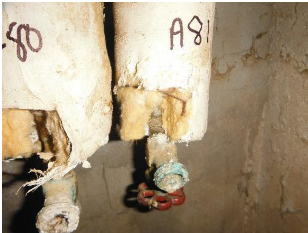
Photo 6: Insulating pipe cement (Sample No. A-81: 20 % Chrysotile asbestos) over fiberglass at end of 12 mm dia. pipe in Lower Mechanical Room. (8 Sept. 2016)
