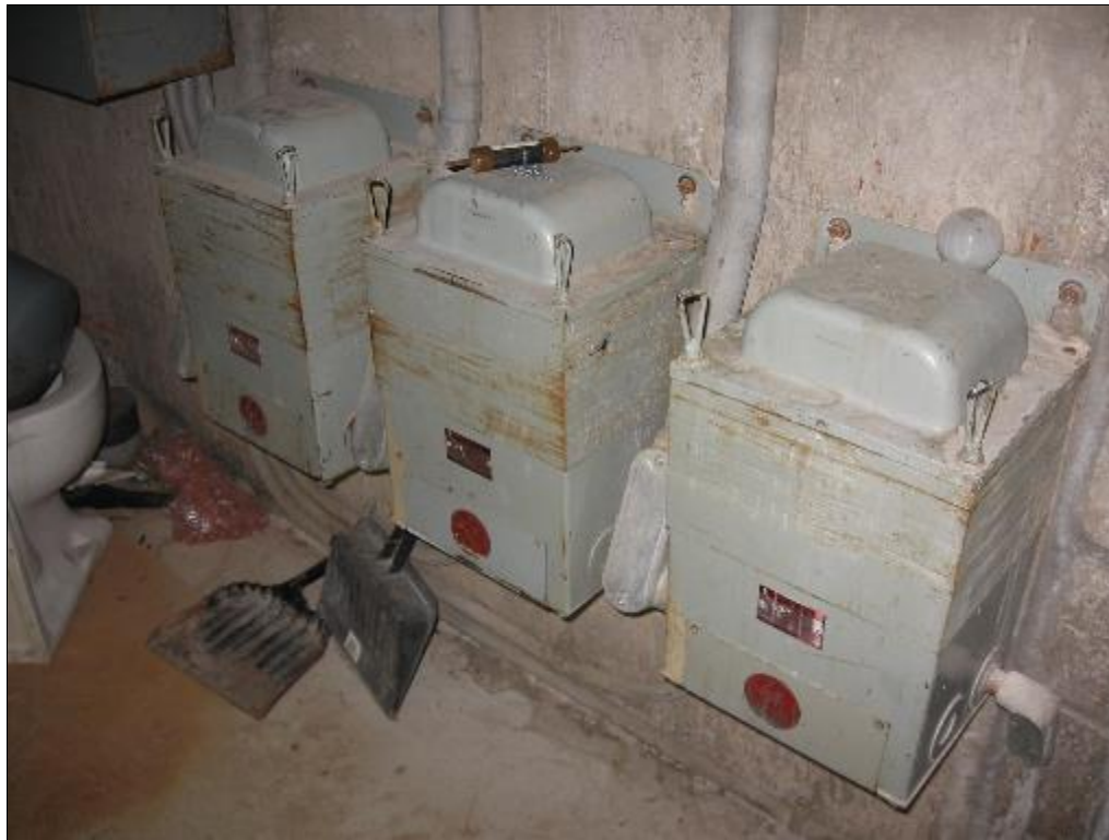
Photo 22: Transformers in Lower Mechanical Room reported to be dry-type (no PCBs). (8 Sept. 2016)
