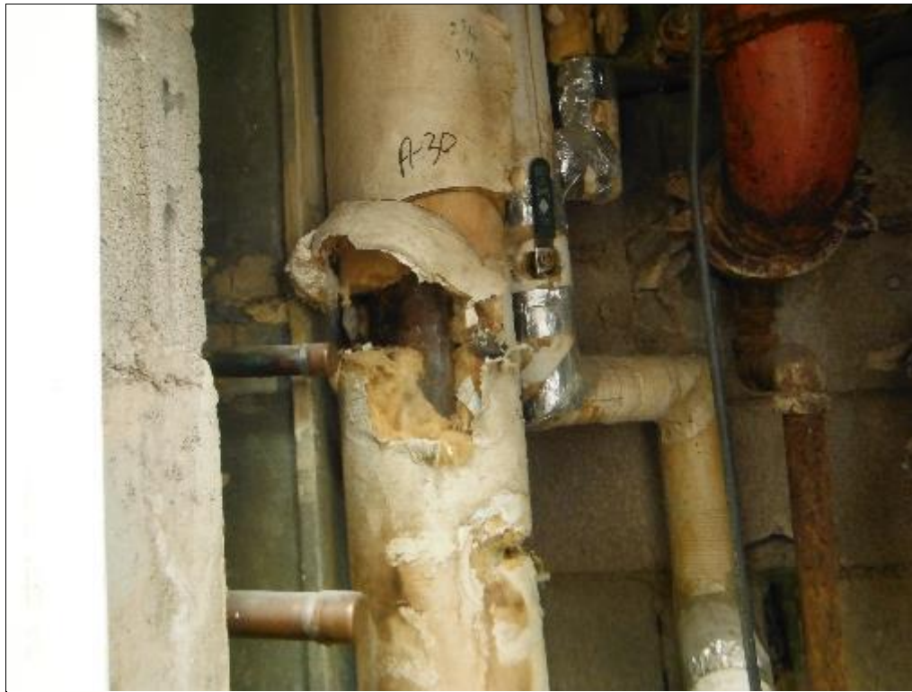
Photo 3: Insulating pipe cement (Sample No. A-30: 15 % Chrysotile asbestos) over fibreglass on 25 mm dia. pipe joint in utility corridor off Rm. 109/111. (8 Sept. 2016)
