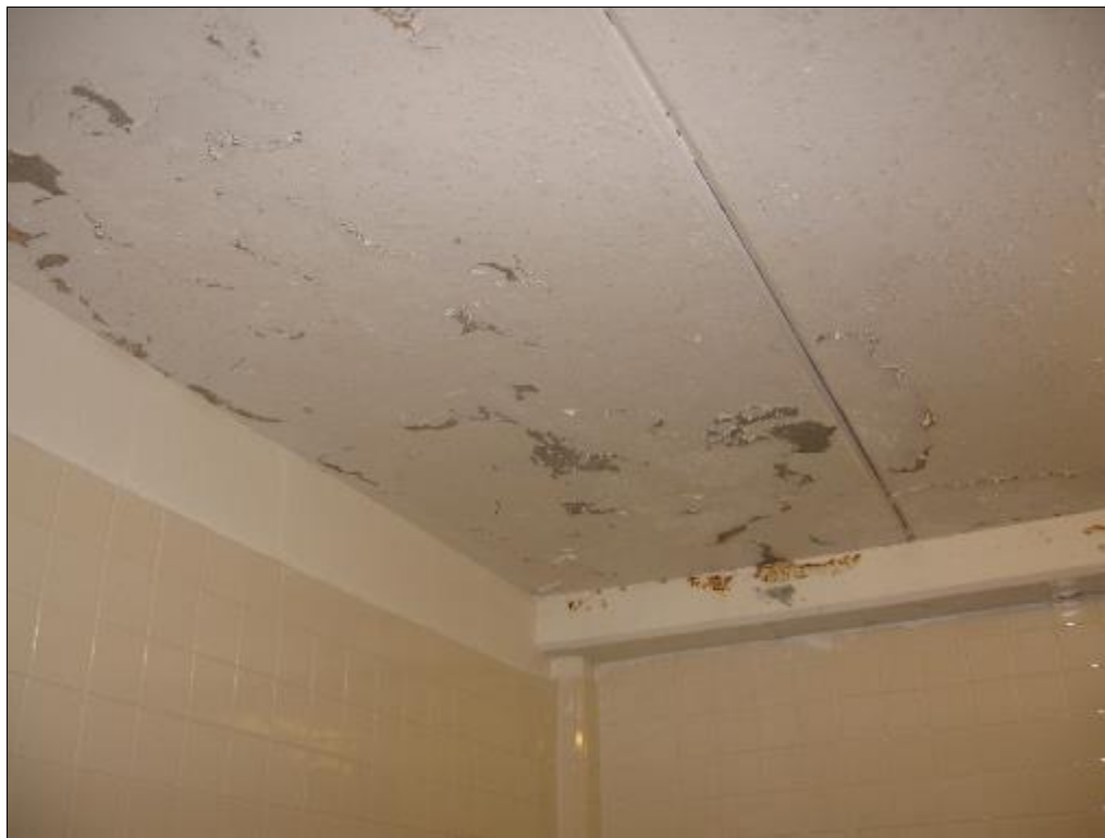
Photo 14: Interior white flaking paint on ceiling in Room A19 (shower). Sample No. P-2. (7 Sept. 2016)
