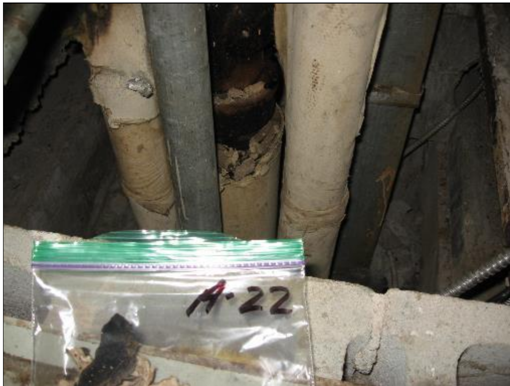
Photo 10: Typical interior of utility corridor via steel door access. Insulating pipe lagging was found to be non-ACM, however traces of insulating cement (parging) suspected on some joints and elbows. (8 Sept. 2016)
