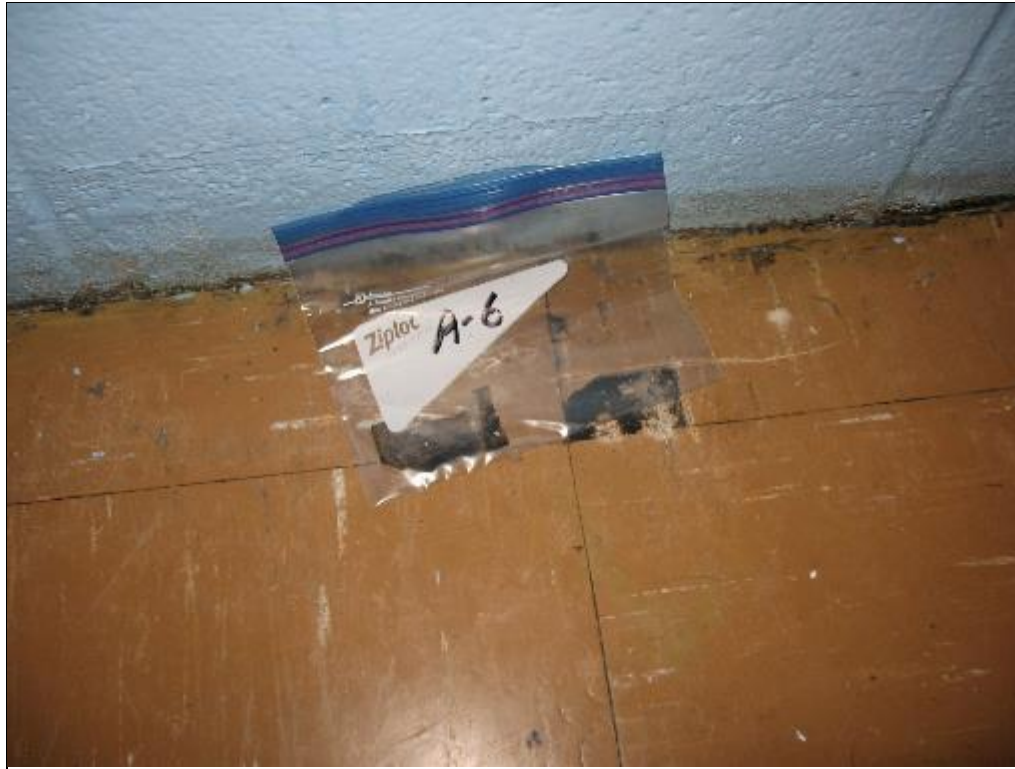
Photo 11: Asbestos-containing (Sample No. A-6: 2% Chrysotile) vinyl floor tile (300 mm x 300 mm, brown with white streaks) in Room A11. (7 Sept. 2016) Same tile observed in nine other cells.
