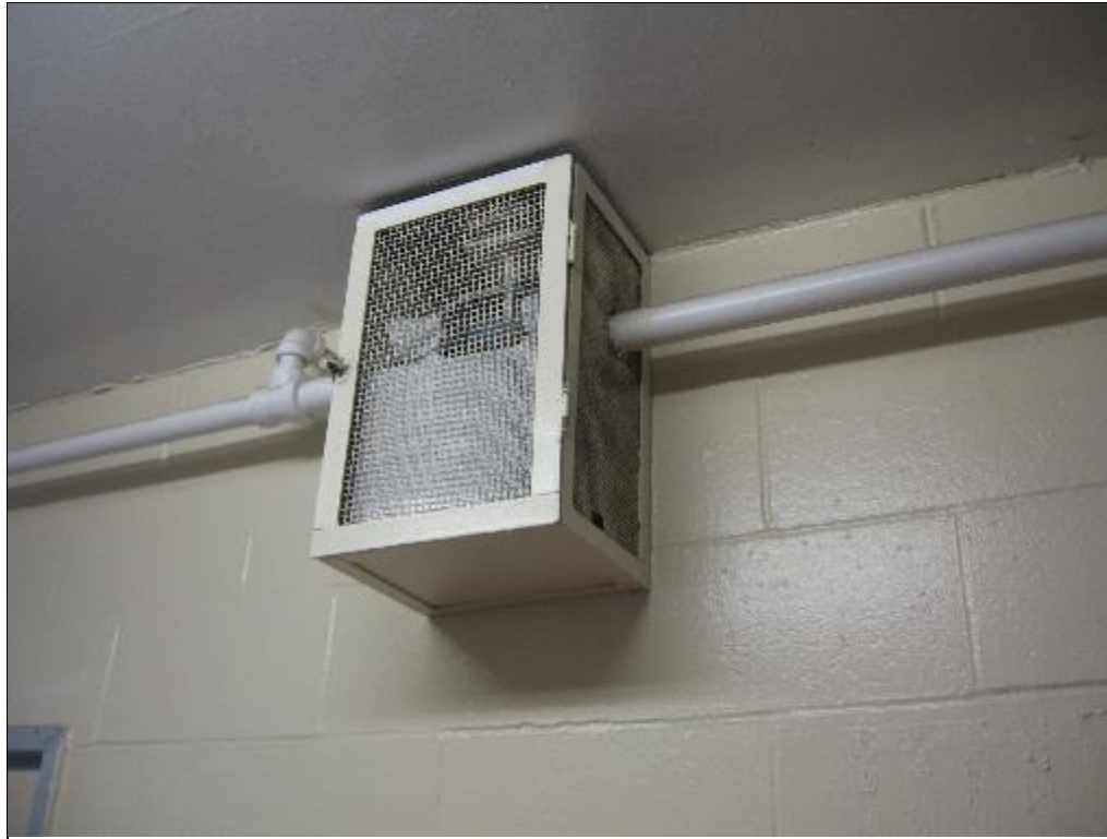
Photo 23: Emergency lighting unit in hallway of main entrance, near Room 104, suspected of containing a lead- acid battery (8 Sept. 2016)
