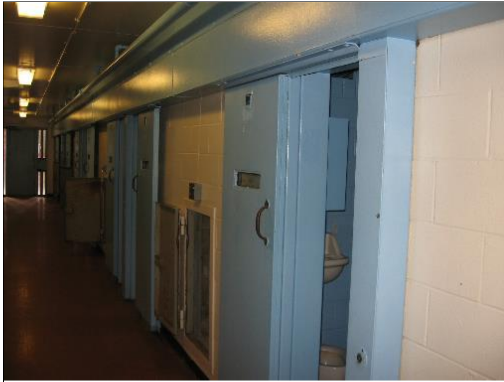
Photo 9: Typical inmate cell wing. Note steel access doors (open) to utility corridors (8 Sept. 2016)
