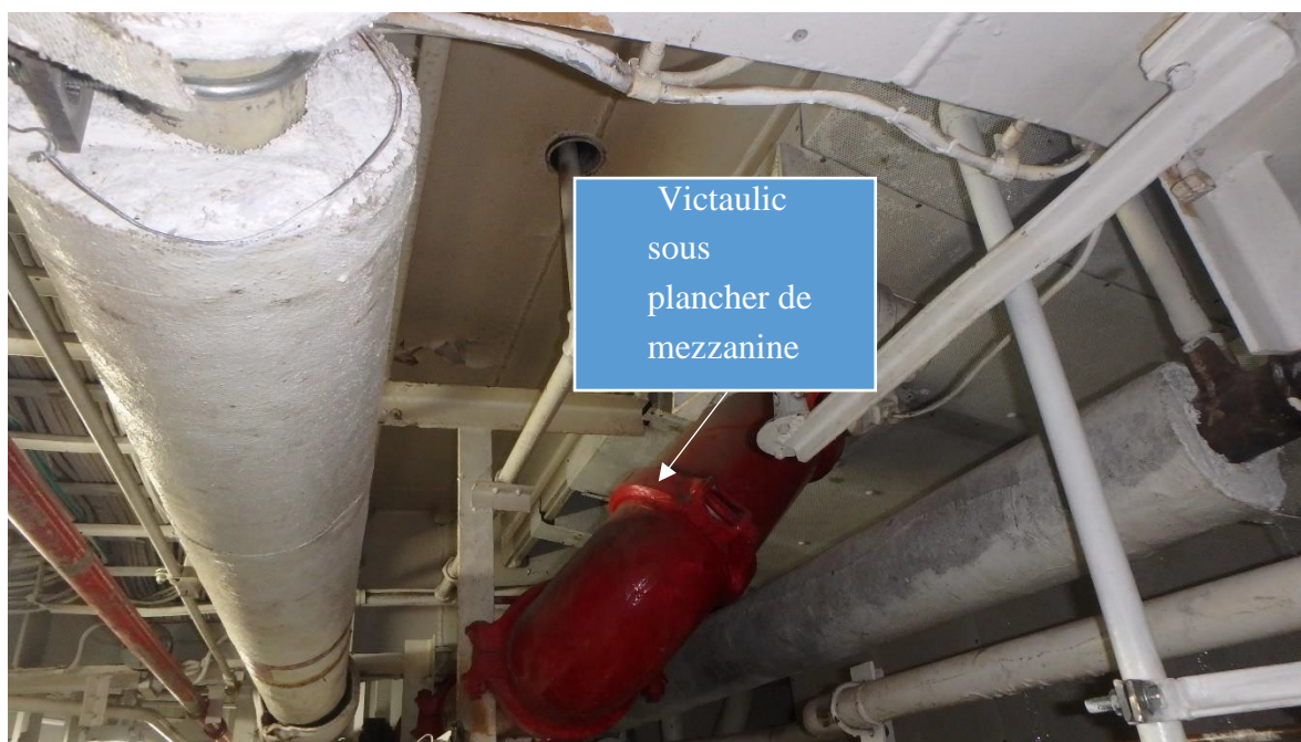
Photo no. 26; tuyau 200mm sous plancher mezzanine
