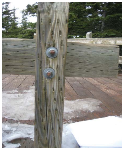
P15: SPLIT DIAPHRAGM ABOVE STRINGER (LOWER LEVEL)
