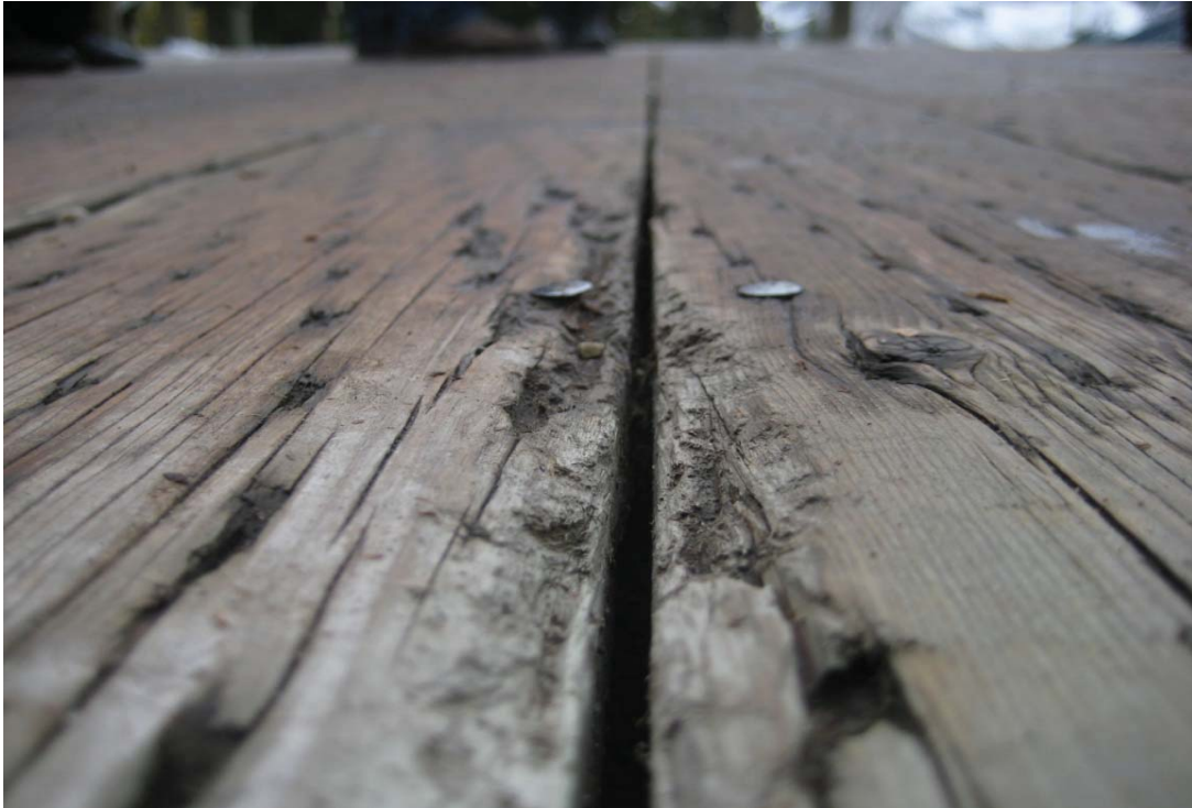
P13: WEAR AND ABRASION ON DECK BOARDS
