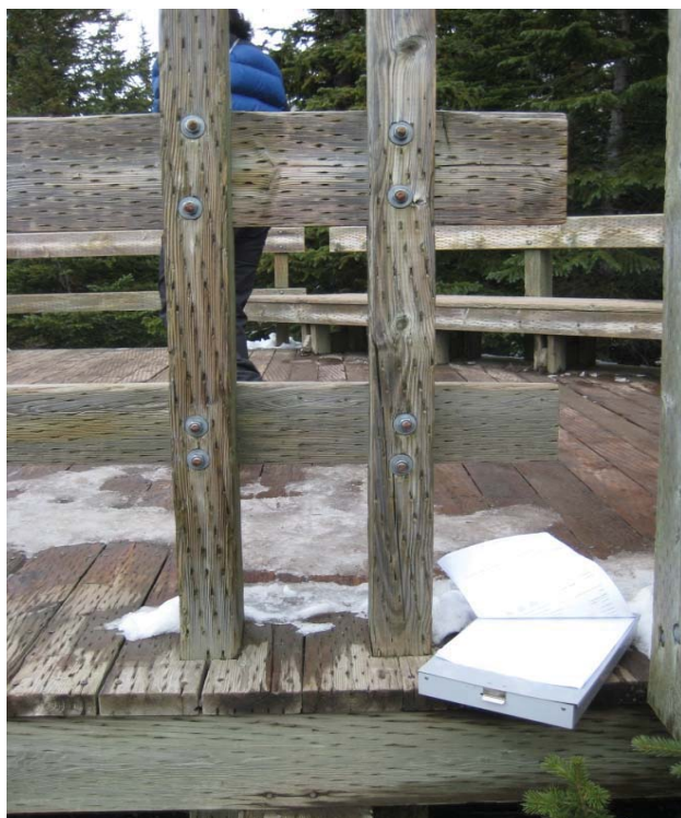
P15: SPLIT DIAPHRAGM ABOVE STRINGER (LOWER LEVEL)
