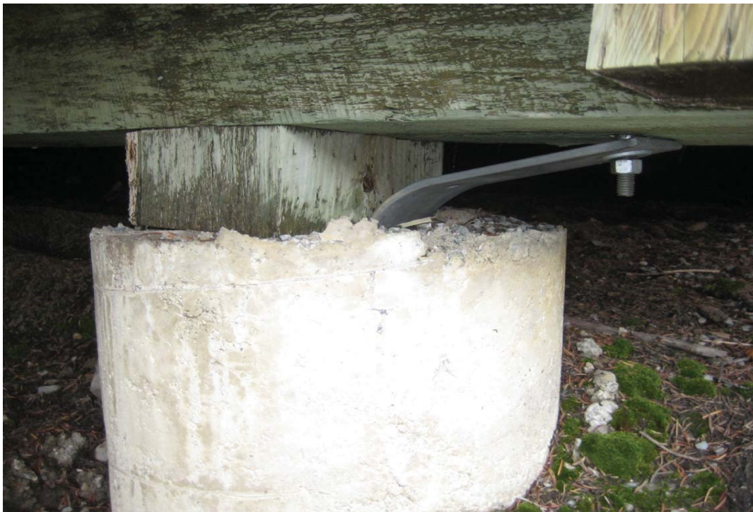
P12: BENT SPLICE PLATE
