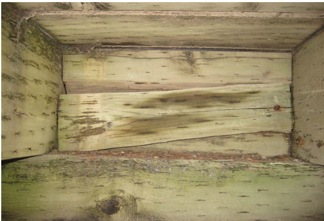
P15: SPLIT DIAPHRAGM ABOVE STRINGER (LOWER LEVEL)
