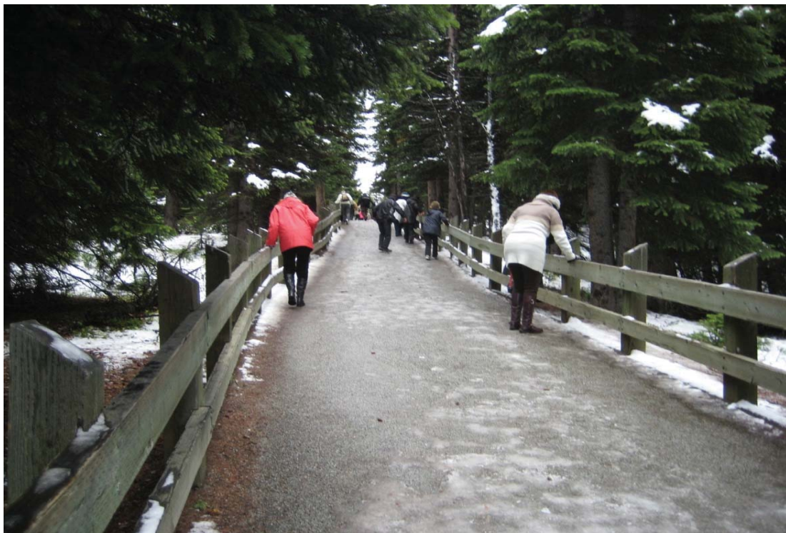
P06: EAST APPROACH LOOKING NORTH. NOTE LOW HEIGHT OF HANDRAILING
