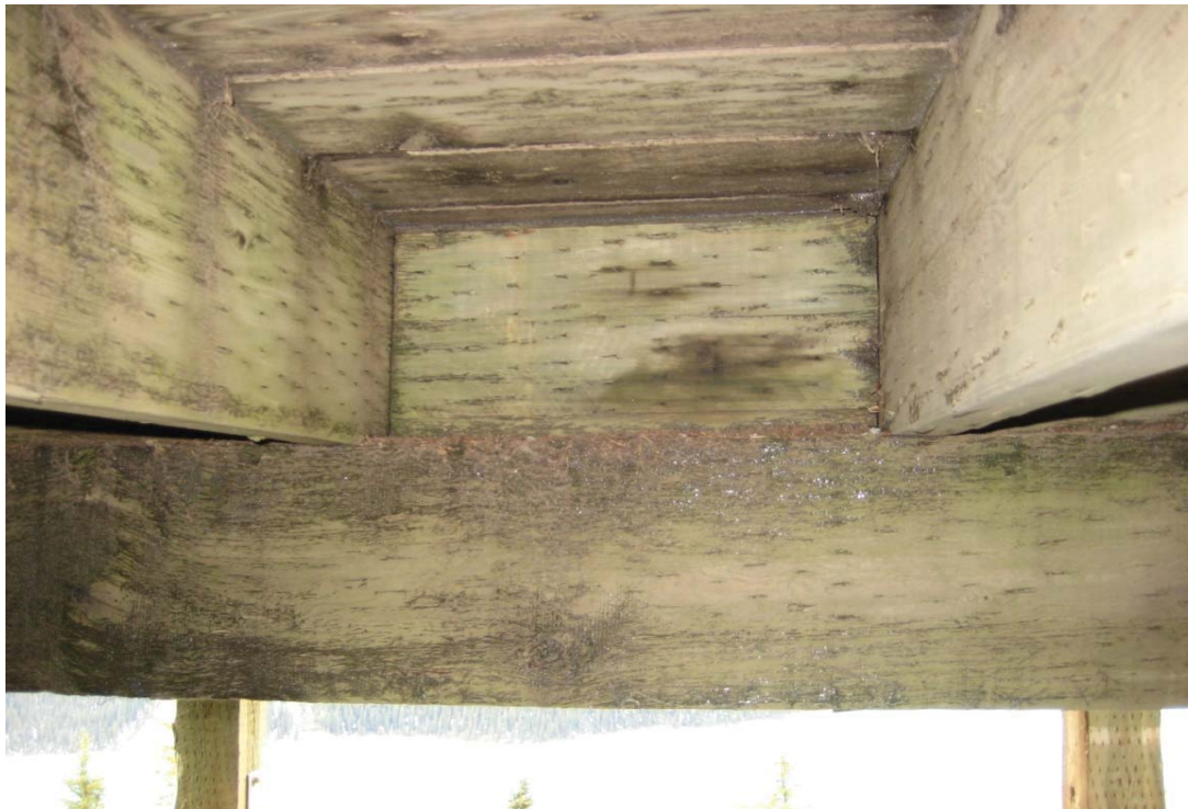
P11: DEBRIS ACCUMULATION ON STRINGERS
