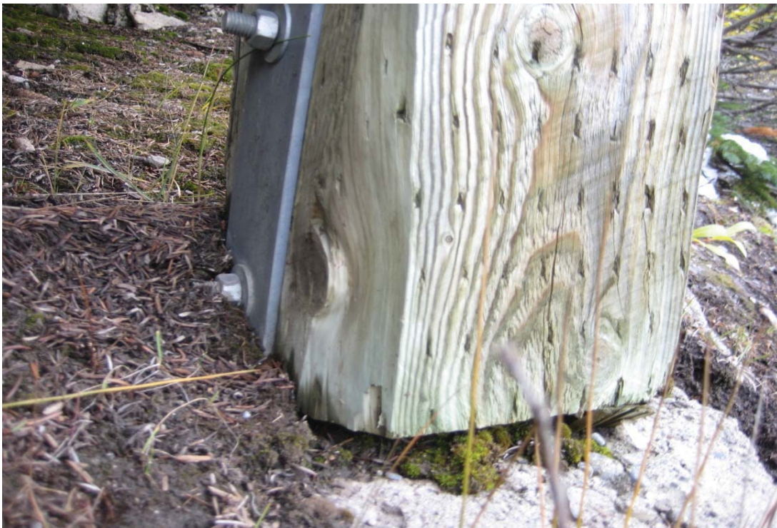
P10: DEBRIS ACCUMULATION AROUND COLUMN BASE
