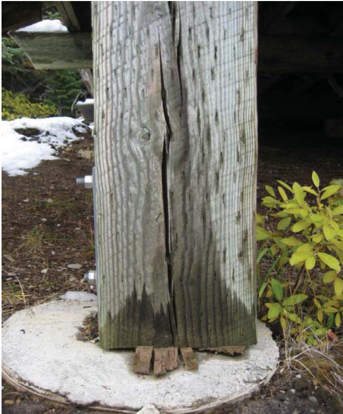
P09: SPLITS IN COLUMN AND POOR BEARING CONTACT WITH FOUNDATION
