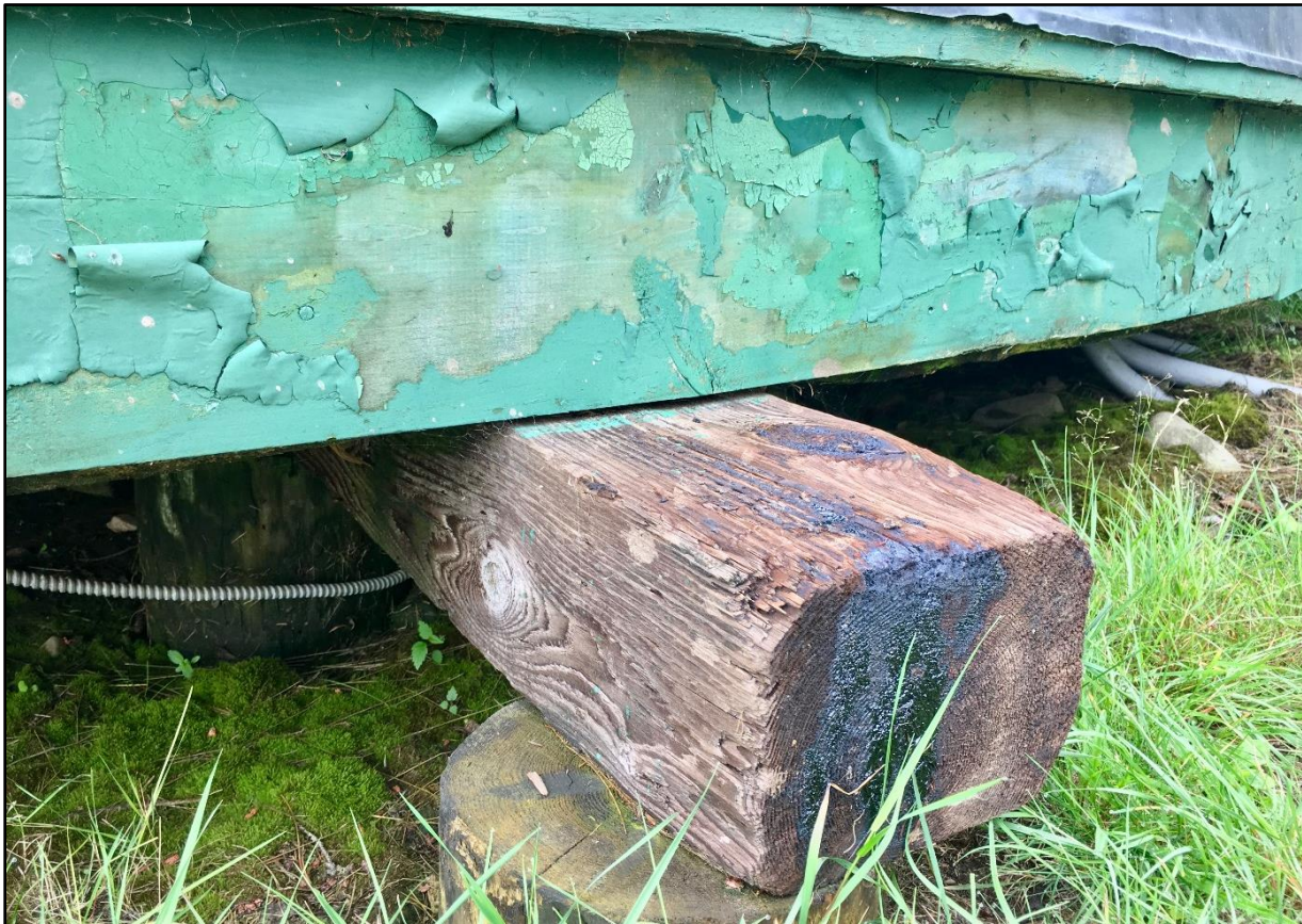
Figure 9. Amphitheatre floor exterior trim covered by lead paint (green) and creosote timber
