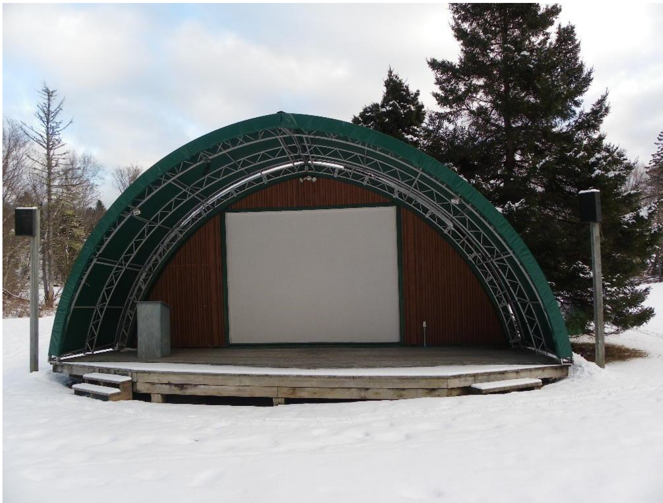
Figure 3. Current Amphitheatre to be demolished and replaced by a new one (PCA Digital Files).
