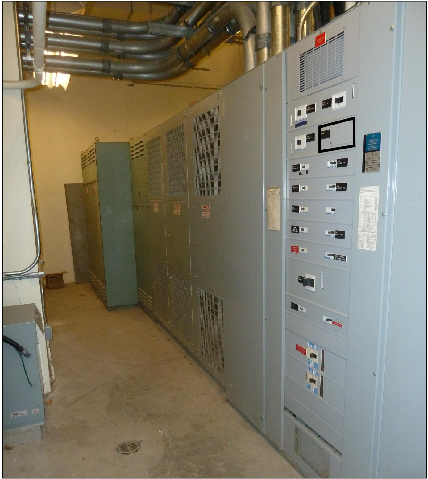
1 EXISTING EMERGENCY DISTRIBUTION PANEL IN BUILDING WA05 SCALE: N.T.S.
