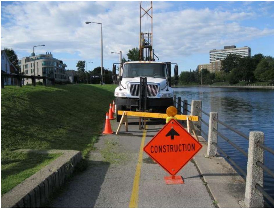
Drilling the borehole E-2
