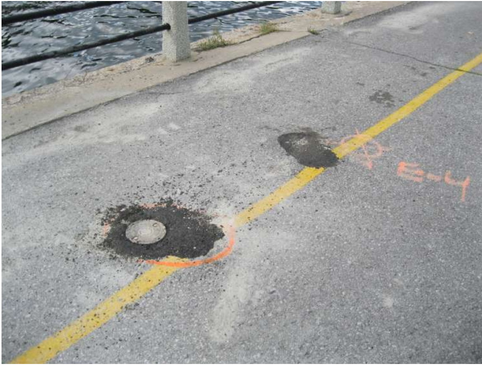
Piezometer cover, backfilling and asphaltting the hole after drilling (borehole E-4)
