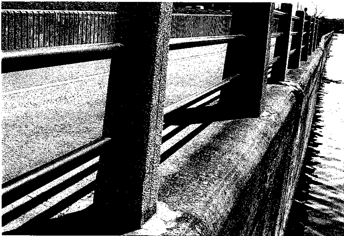
Typical deterioration at joint, looking South from B.H. 103
