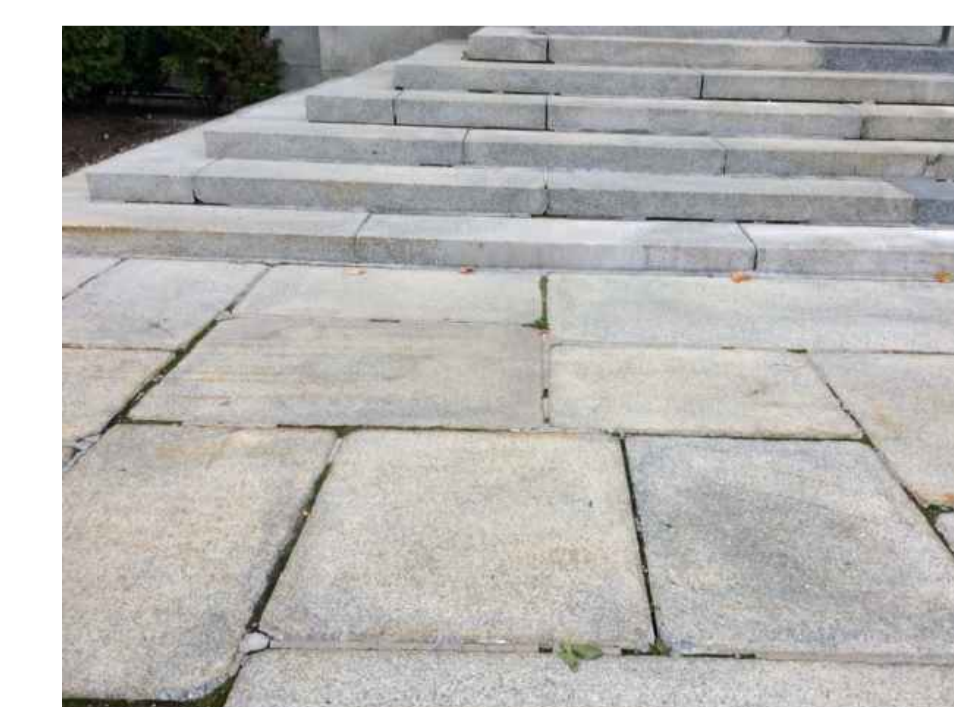
9 G01 EXISTING VIEW @ FRONT STEPS SCALE = N.T.S.
