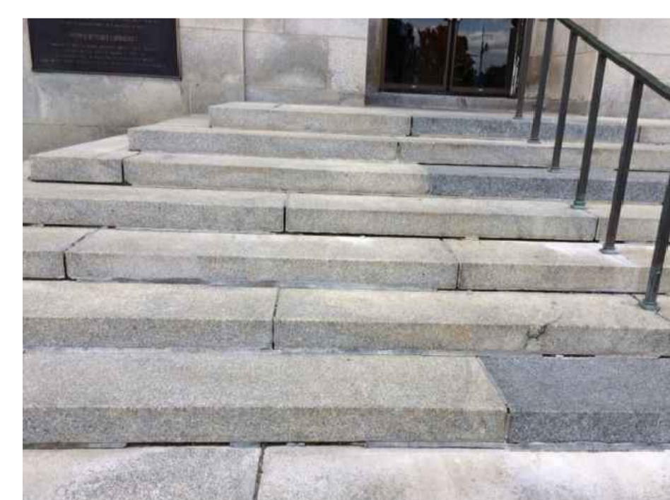
7 G01 EXISTING VIEW @ FRONT STEPS SCALE = N.T.S.
