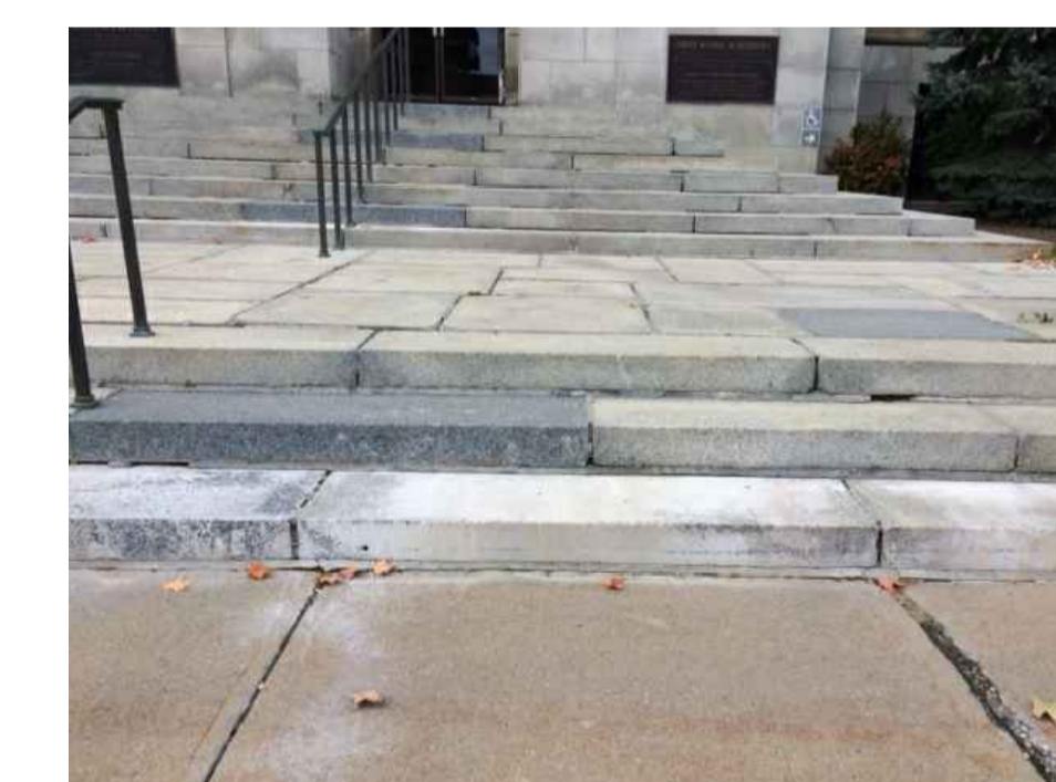
6 G01 EXISTING VIEW @ FRONT STEPS SCALE = N.T.S.
