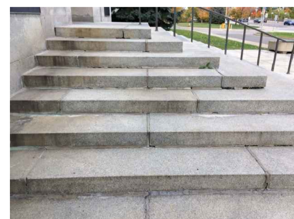
4 G01 EXISTING VIEW @ FRONT STEPS SCALE = N.T.S.
