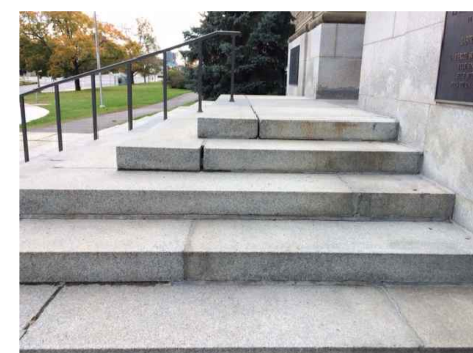
5 G01 EXISTING VIEW @ FRONT STEPS SCALE = N.T.S.
