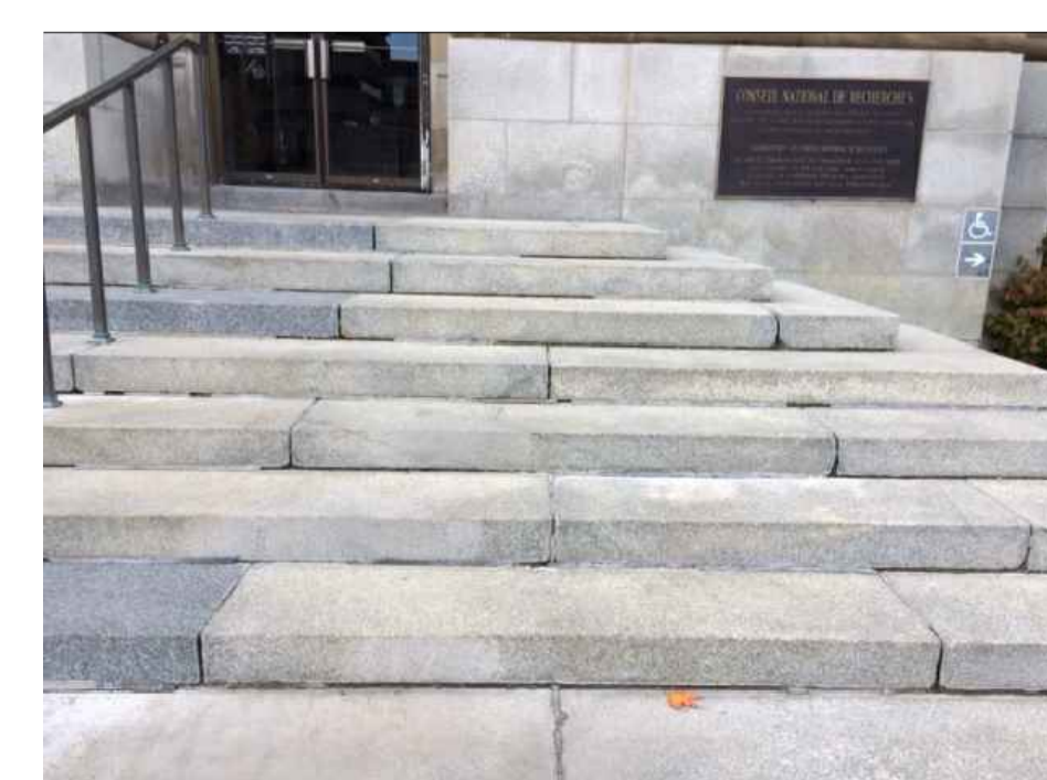
8 G01 EXISTING VIEW @ FRONT STEPS SCALE = N.T.S.
