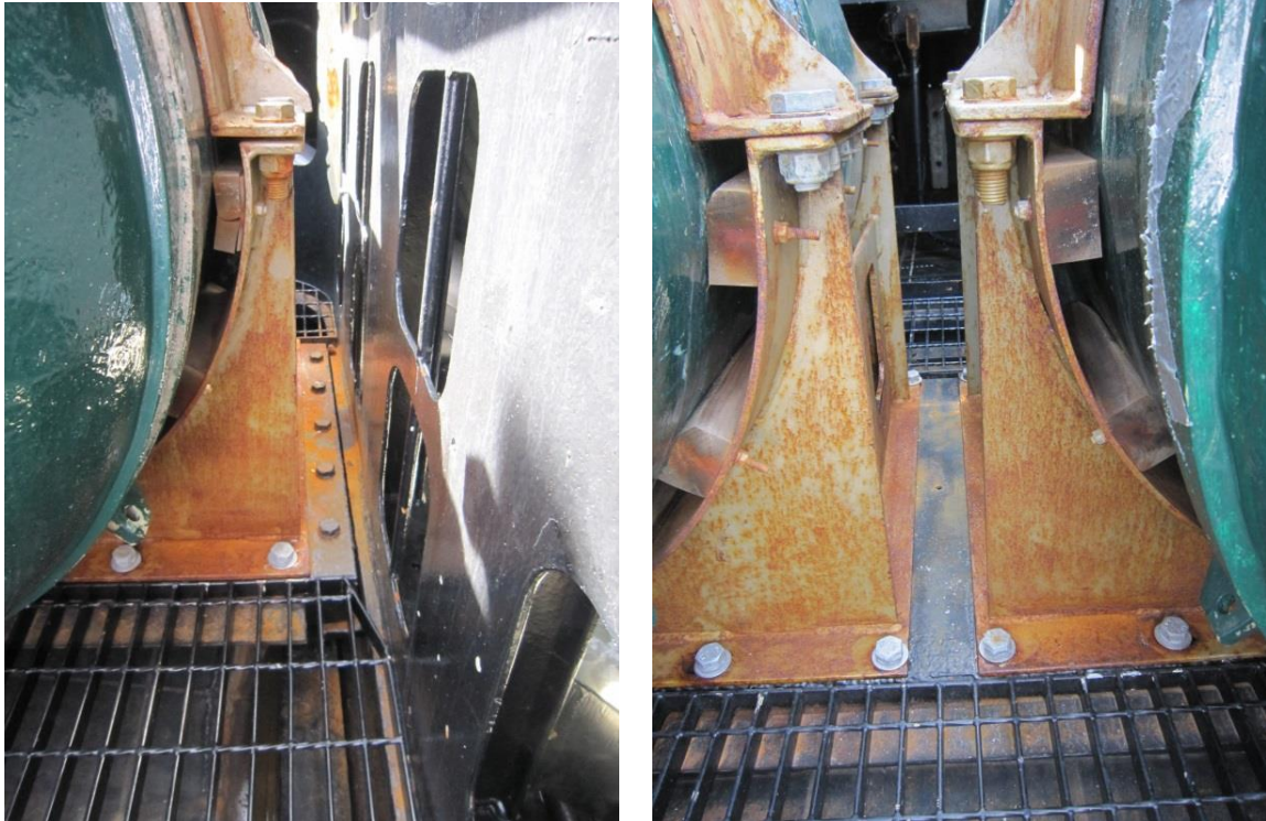
Figure 2: WTPV Cradle and Steel Plate Anchors
