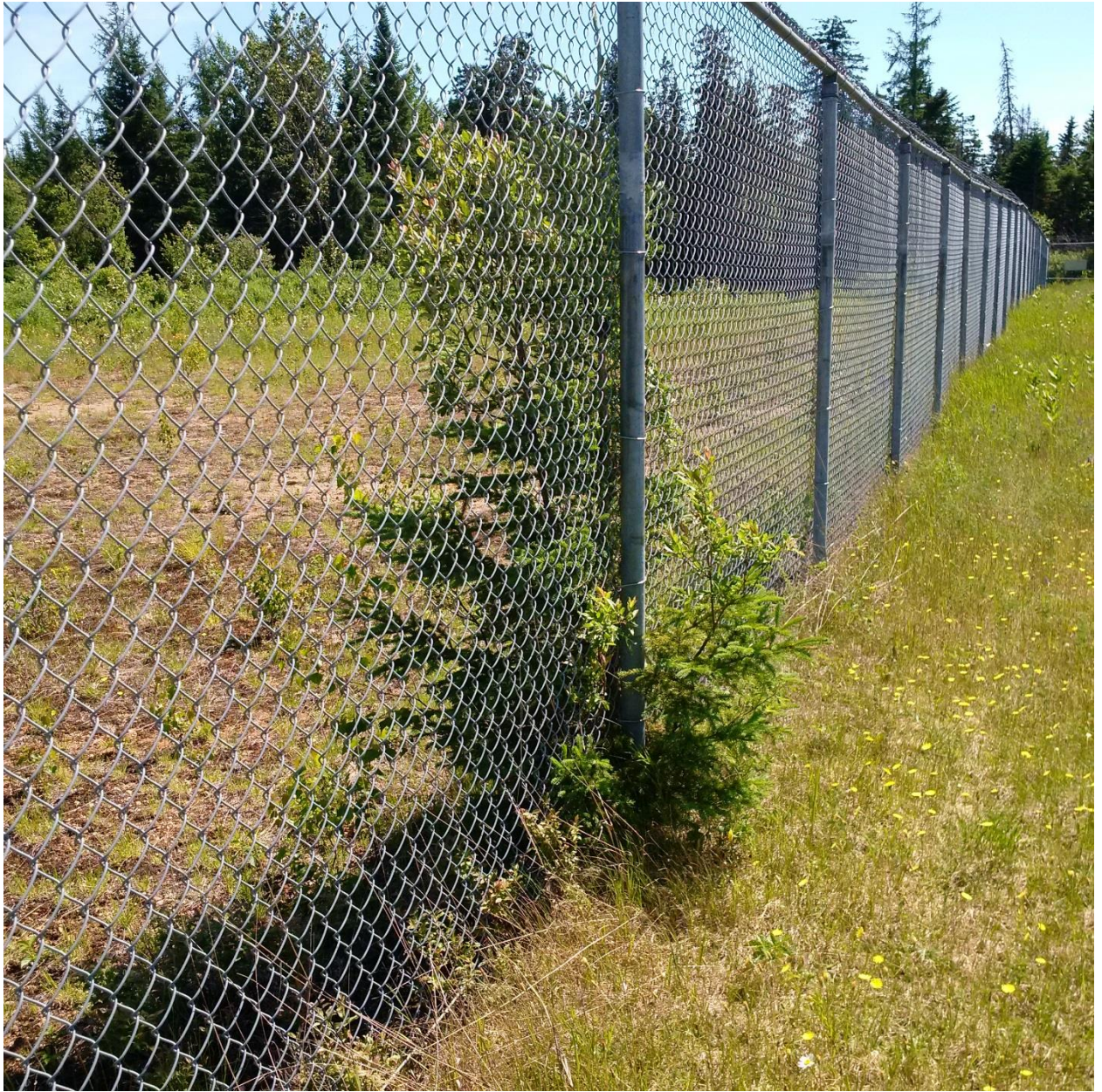
Project : Vegetation control in the Mags sector
