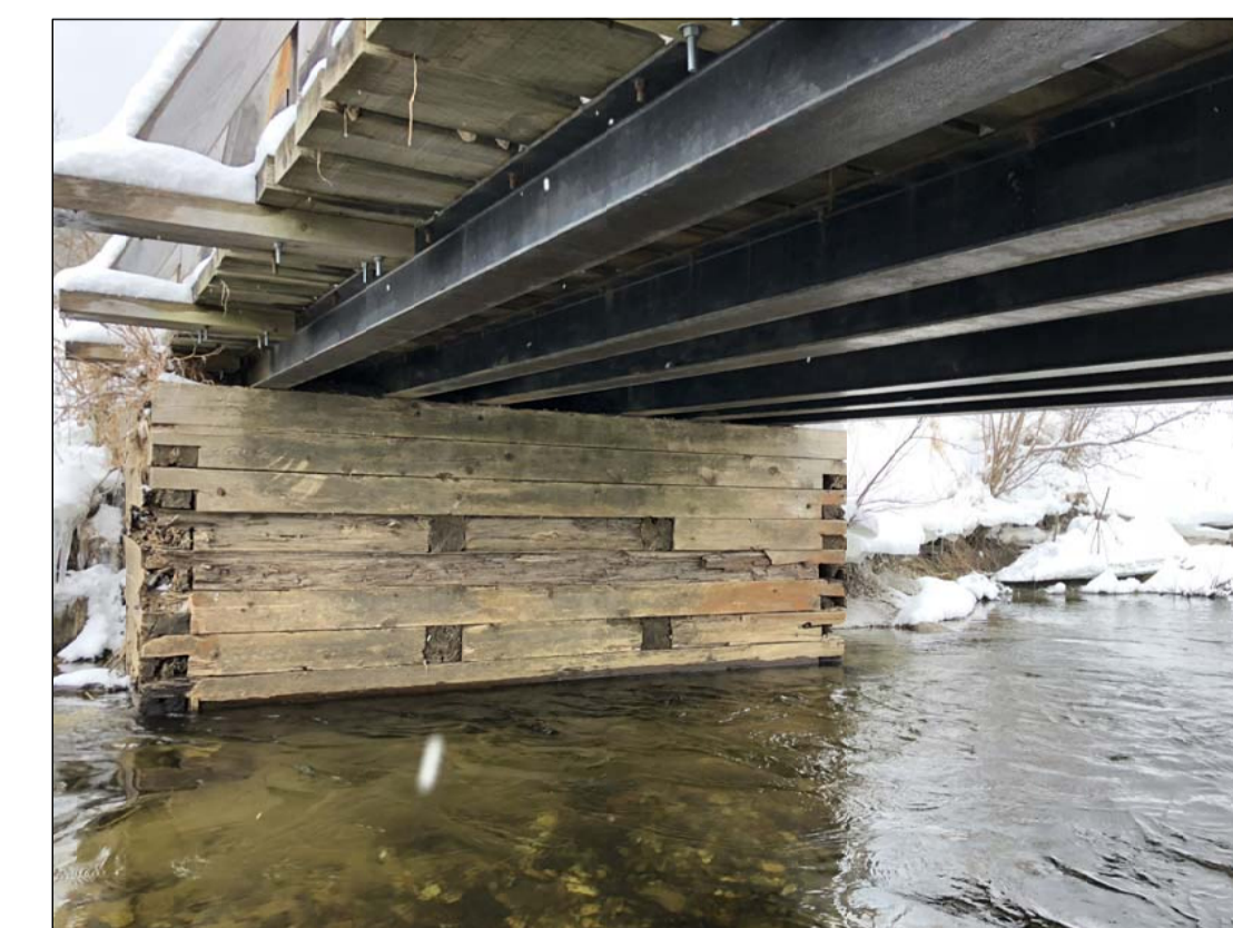
LE DESSOUS DE LA STRUCTURE EXISTANTE: NIVEAU D'EAU TYPIQUE HORS DE PRINTEMPS UNDERSIDE OF EXISTING STRUCTURE: TYPICAL WATER ELEVATION OUTSIDE OF SPRING FLOODING
