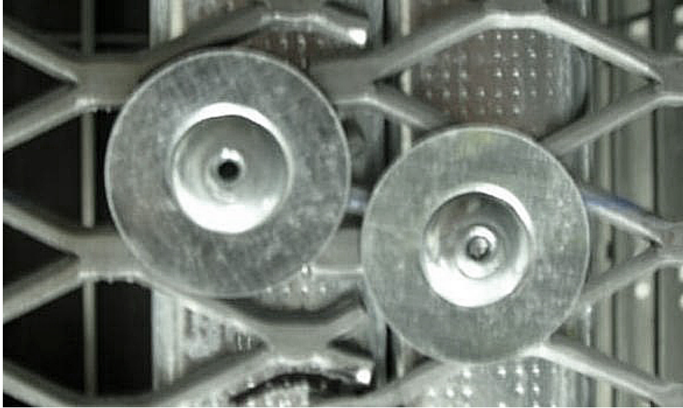
Figure 5: Example of Mesh Interlay Seam, Riveted
