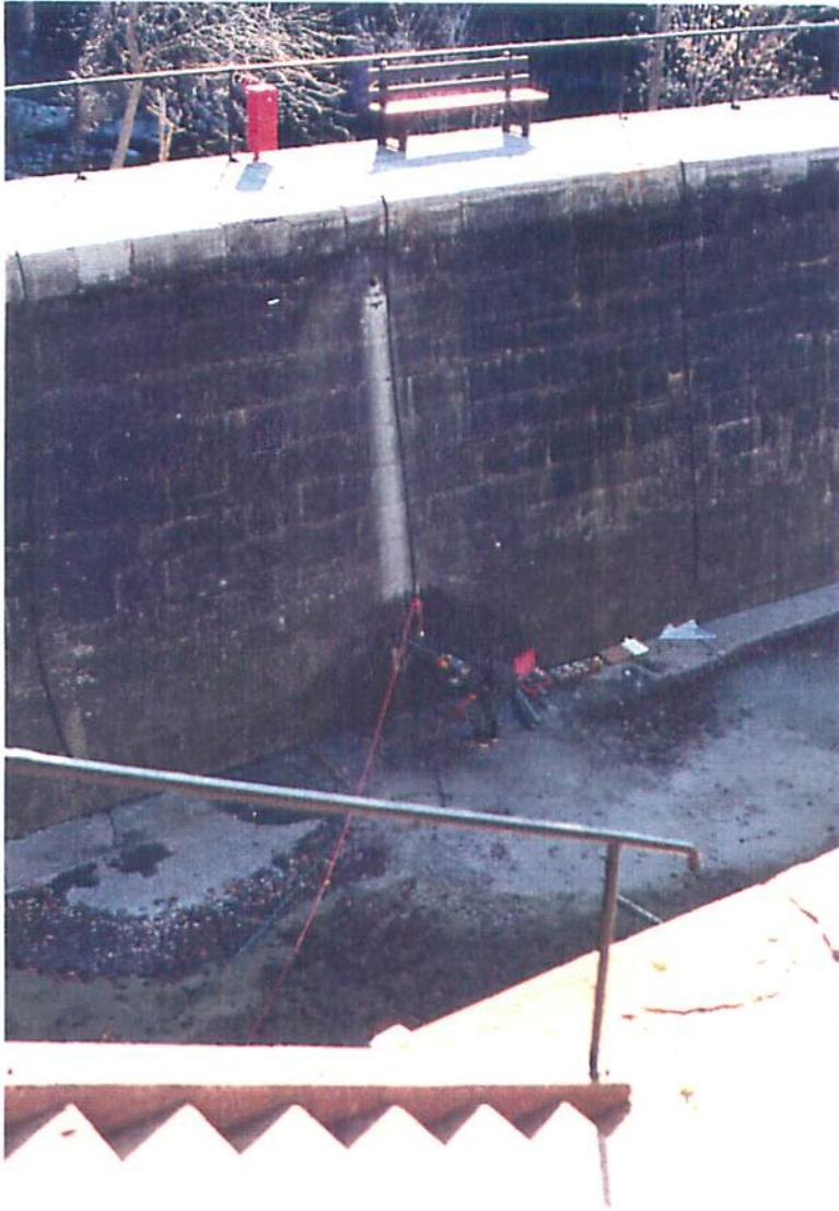
Photograph No. 11 Coring of Hole No. H17
