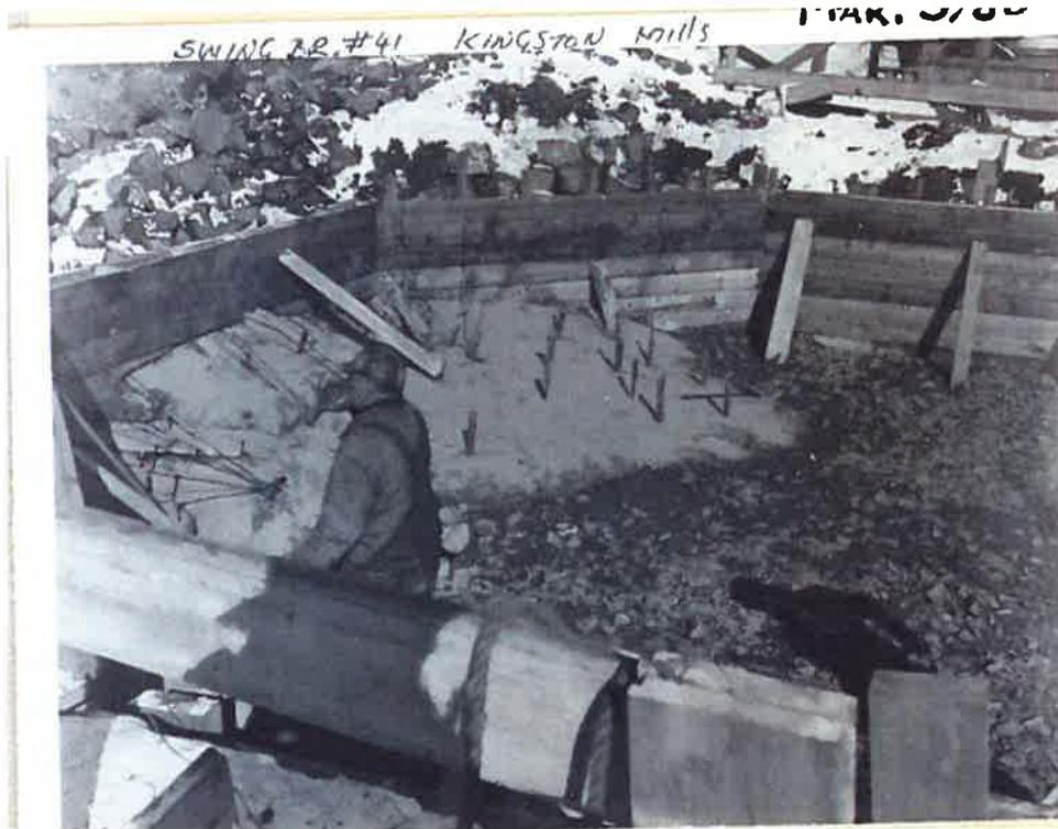
Photograph 2 – Showing the construction of original pier founded on the bedrock on the west side with dowels into the bedrock.
