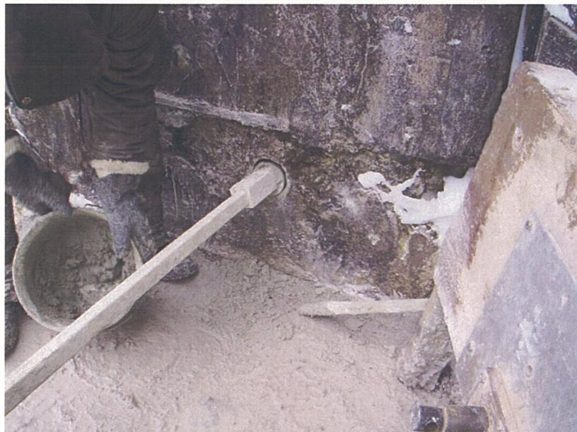
**Photo 4** – BH 05-2, Repair using drypack non-shrinkage grout
