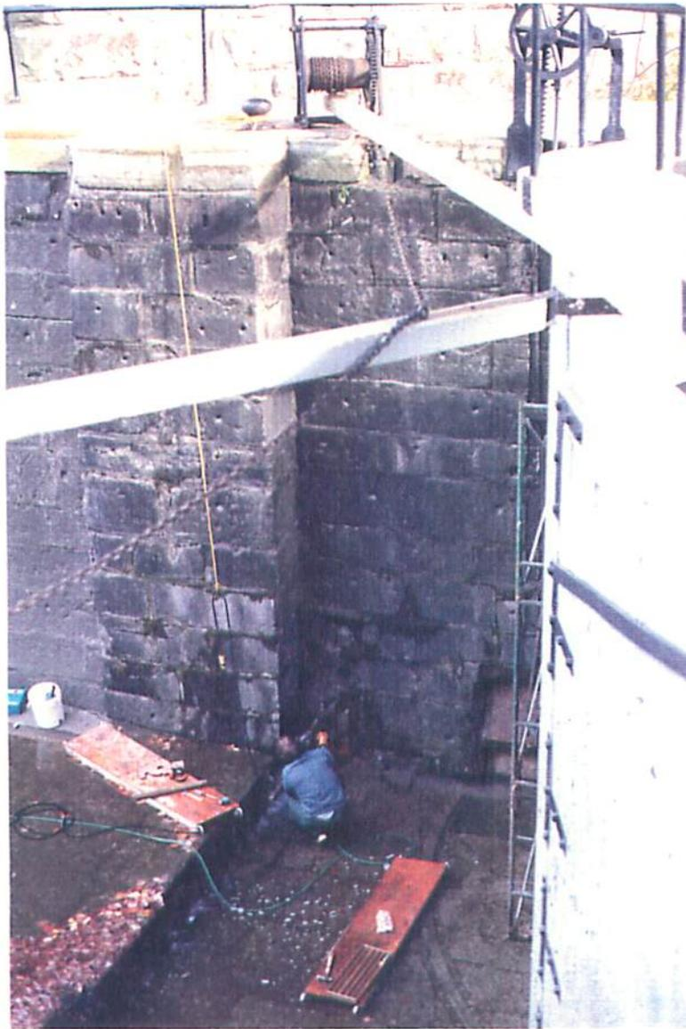
Photograph No. 10 Coring of Hole No. H15
