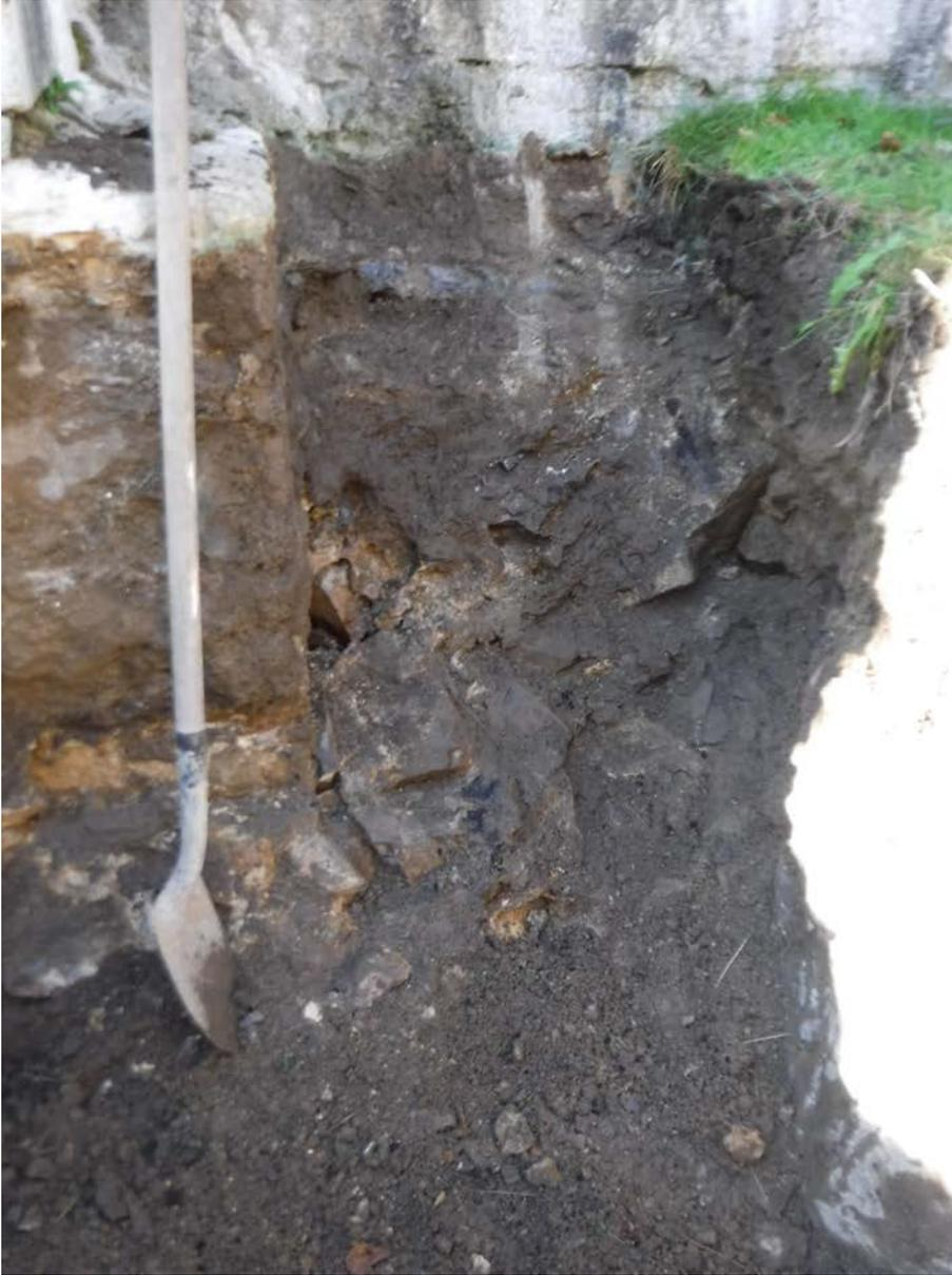
Test Pit #3 – Grouted rubble at base of chamber wall
