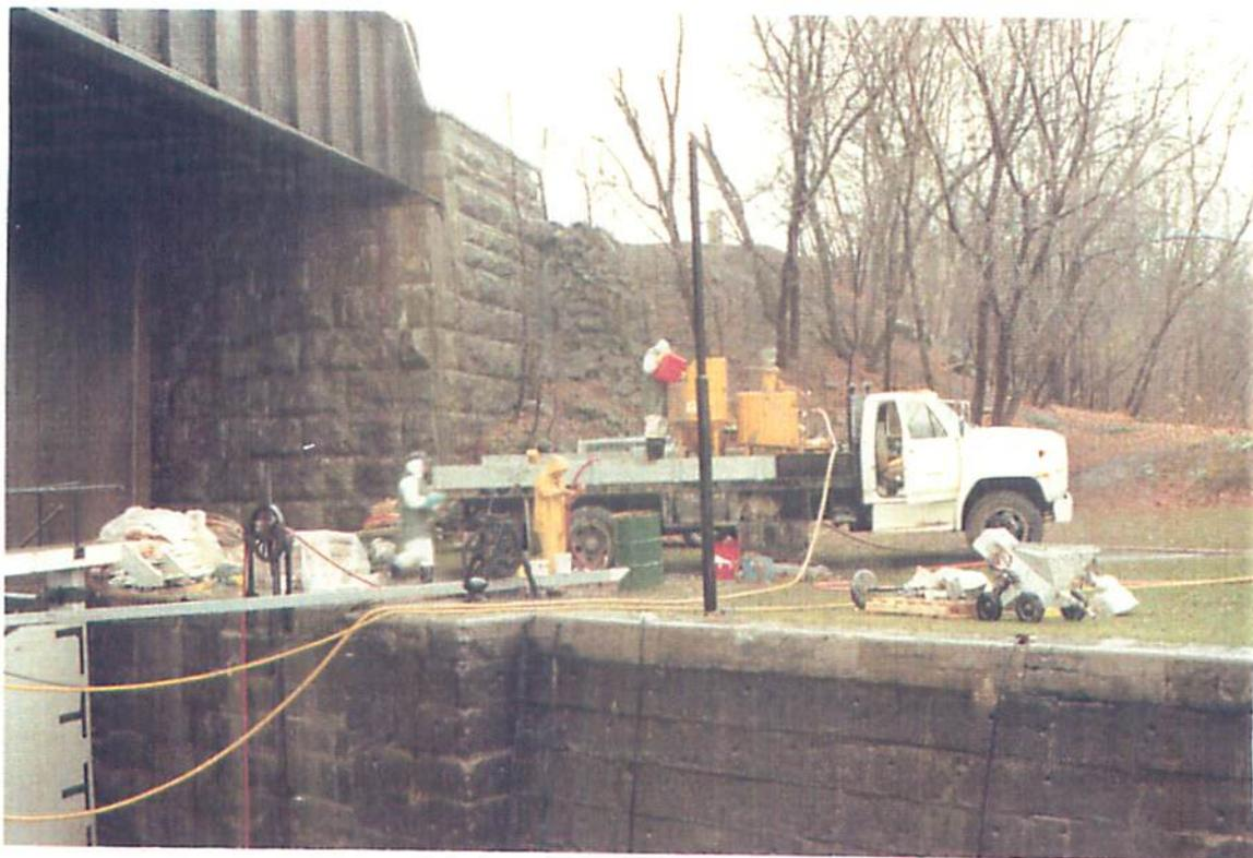
Colloidal Grouting Plant Shown During Test Program
