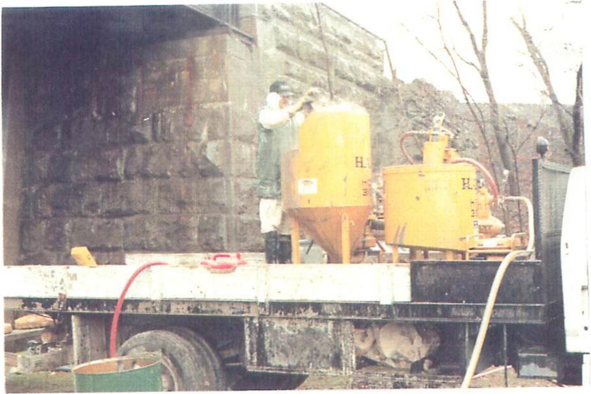
Colloidal Grouting Plant Shown During Test Program
