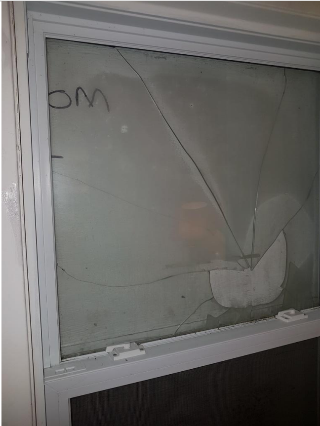
Photo 29 – Trailer, Broken Sealed Unit in Window (Window is Covered with Plywood on Exterior)
