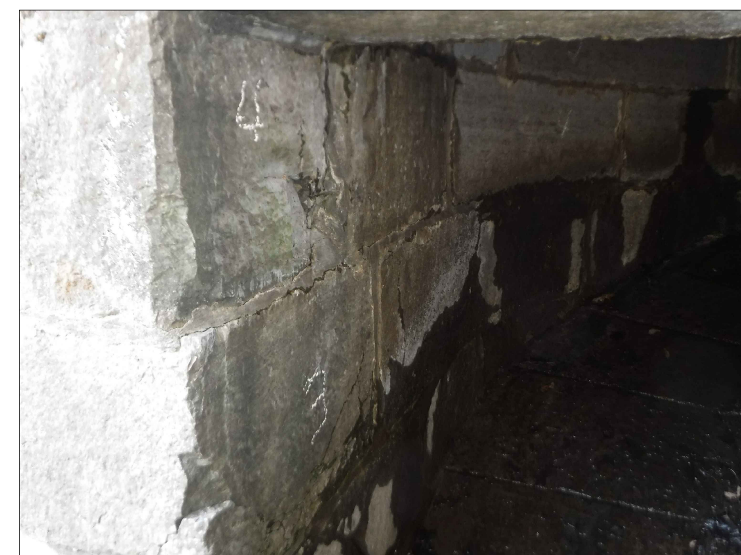
WEST SLUICE TUNNEL LOOKING UP - 2017
