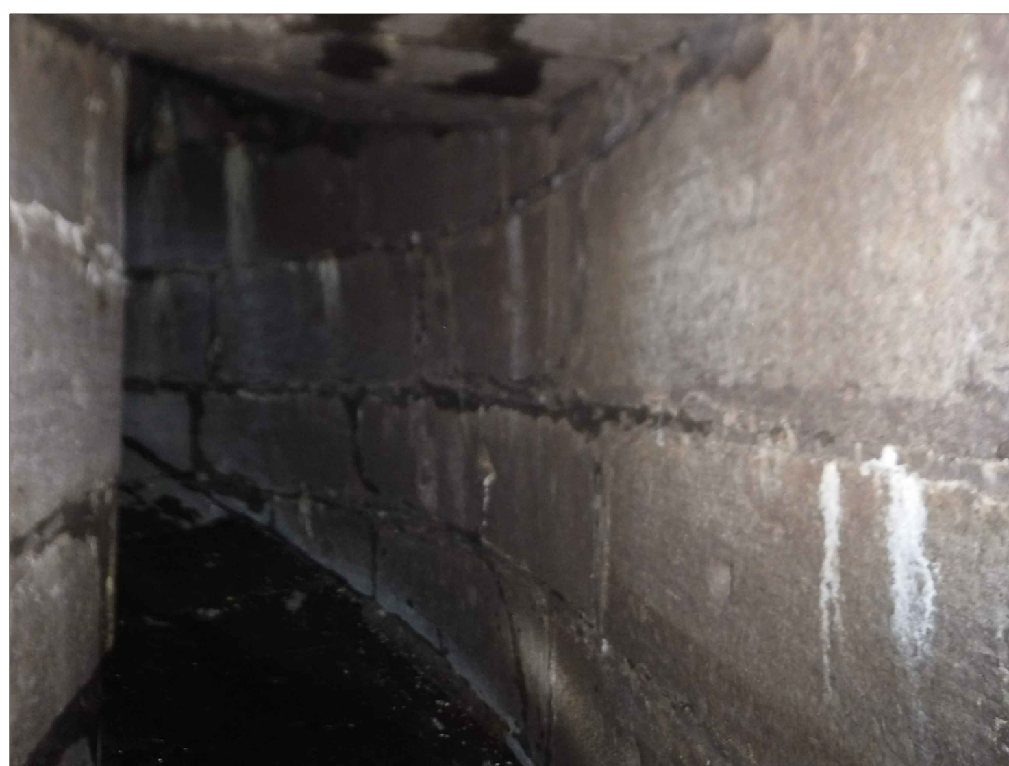
EAST SLUICE TUNNEL LOOKING UP - 2017
