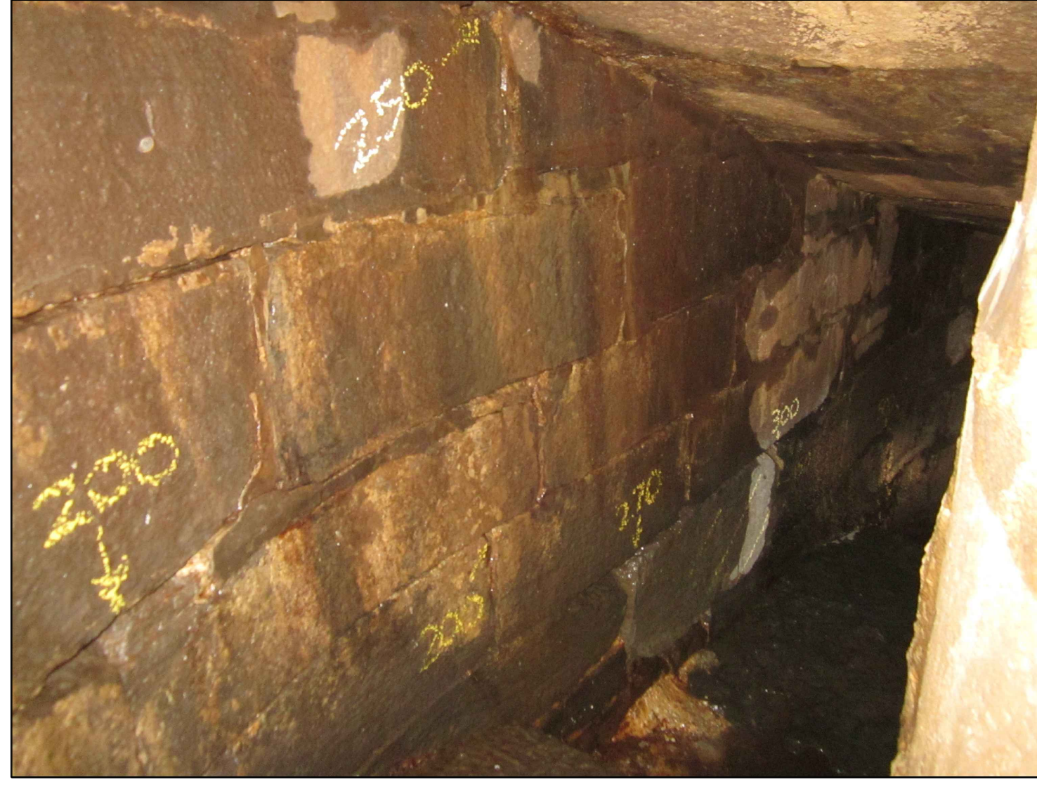
EAST SLUICE TUNNEL LOOKING DOWN 2017
