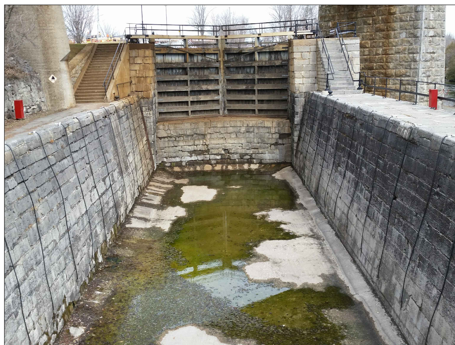
CHAMBER FLOOR (LOOKING NORTH) - 2017
