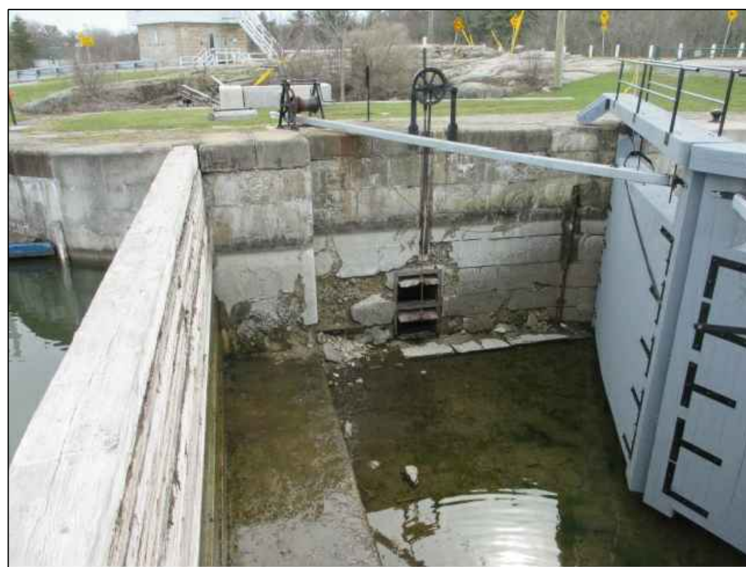
EAST UPPER GATE WALL
