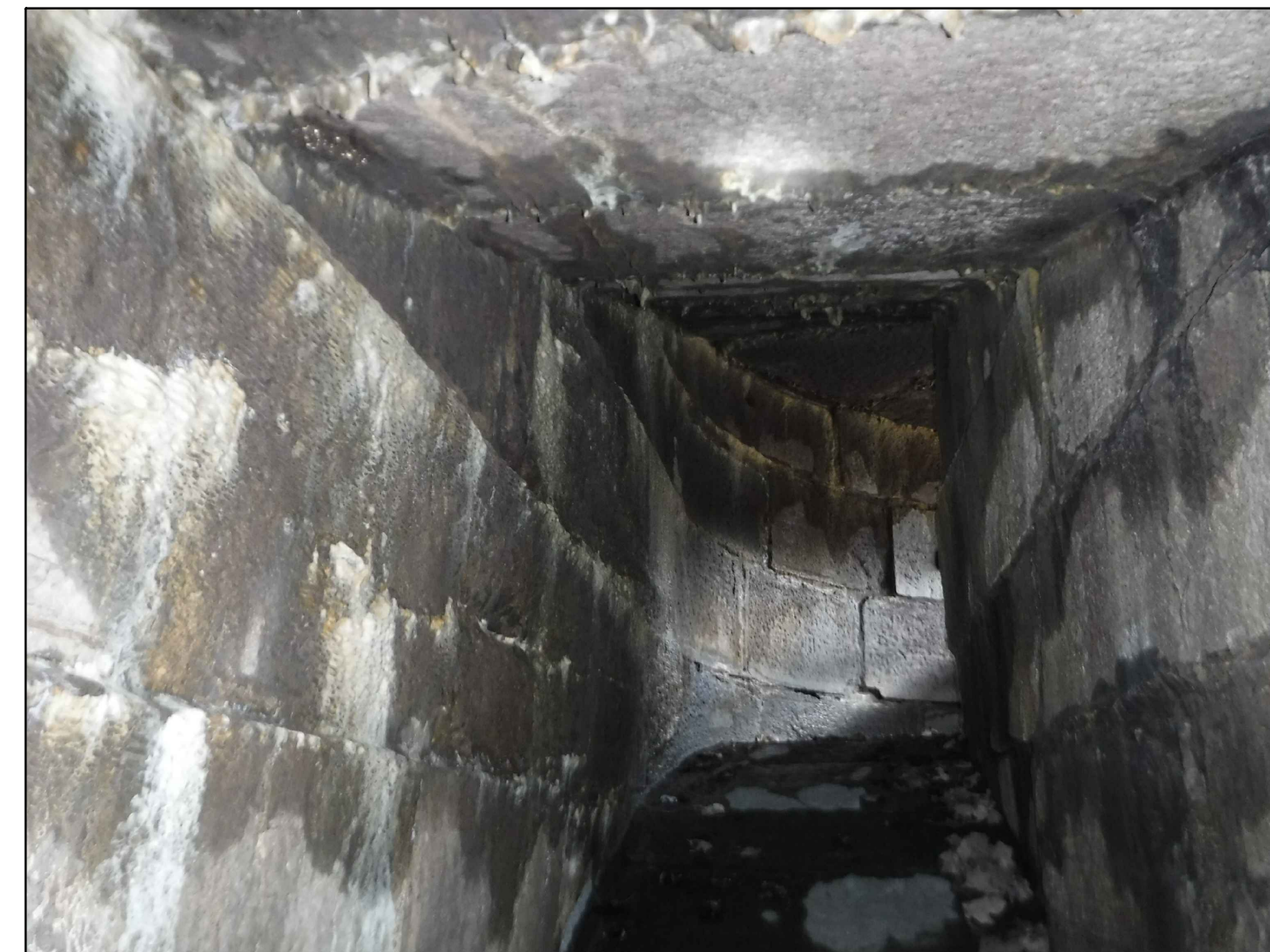
WEST SLUICE TUNNEL LOOKING DOWN - 2017
