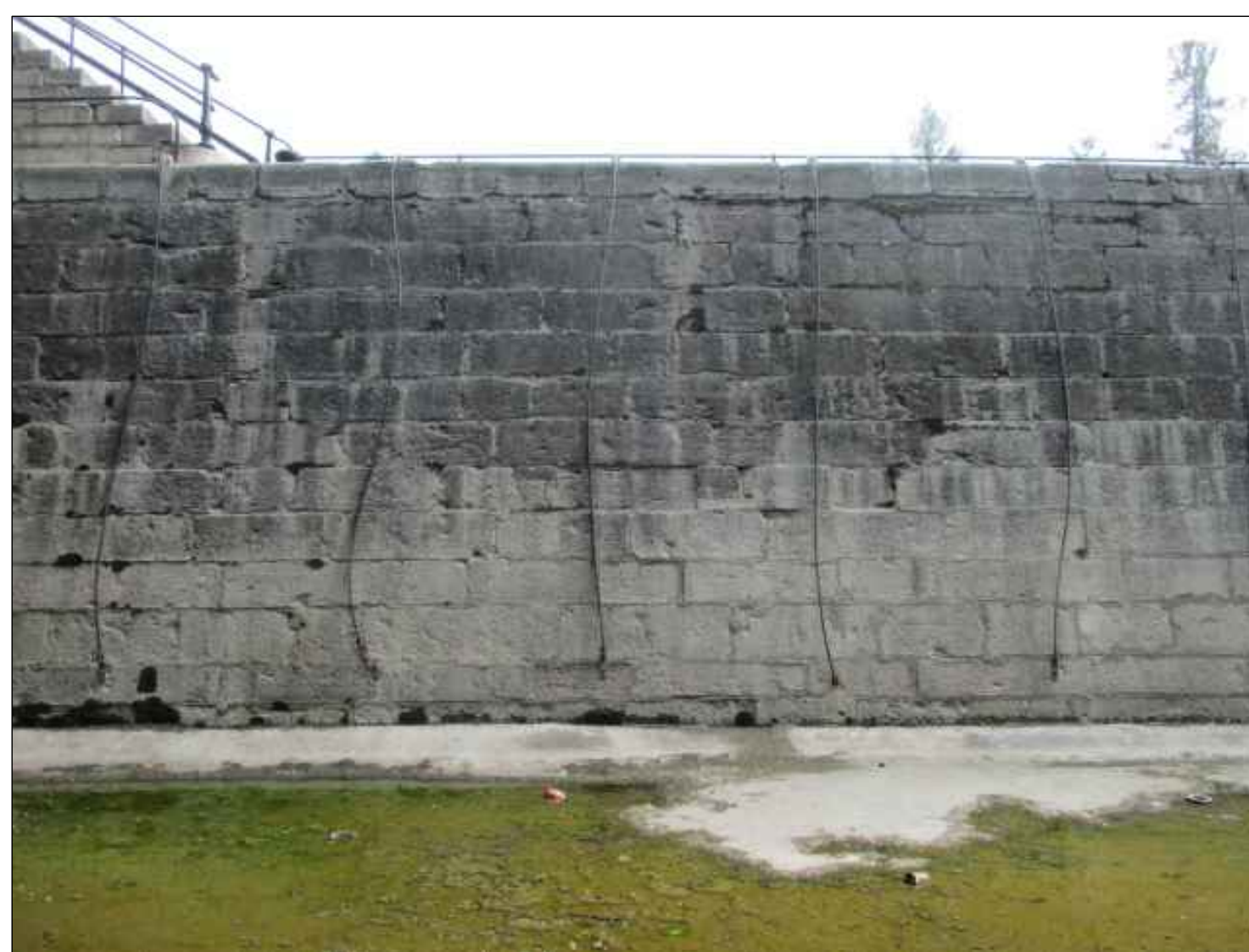
EAST CHAMBER WALL
