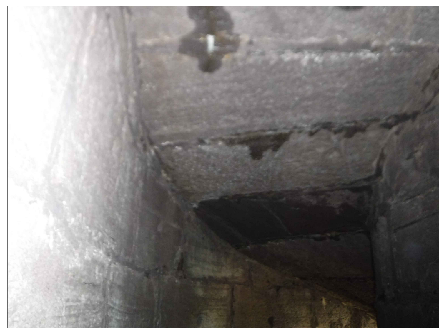
EAST SLUICE TUNNEL LOOKING DOWN - 2017
