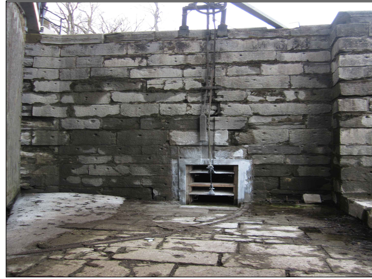
WEST WALL LOWER PIER
