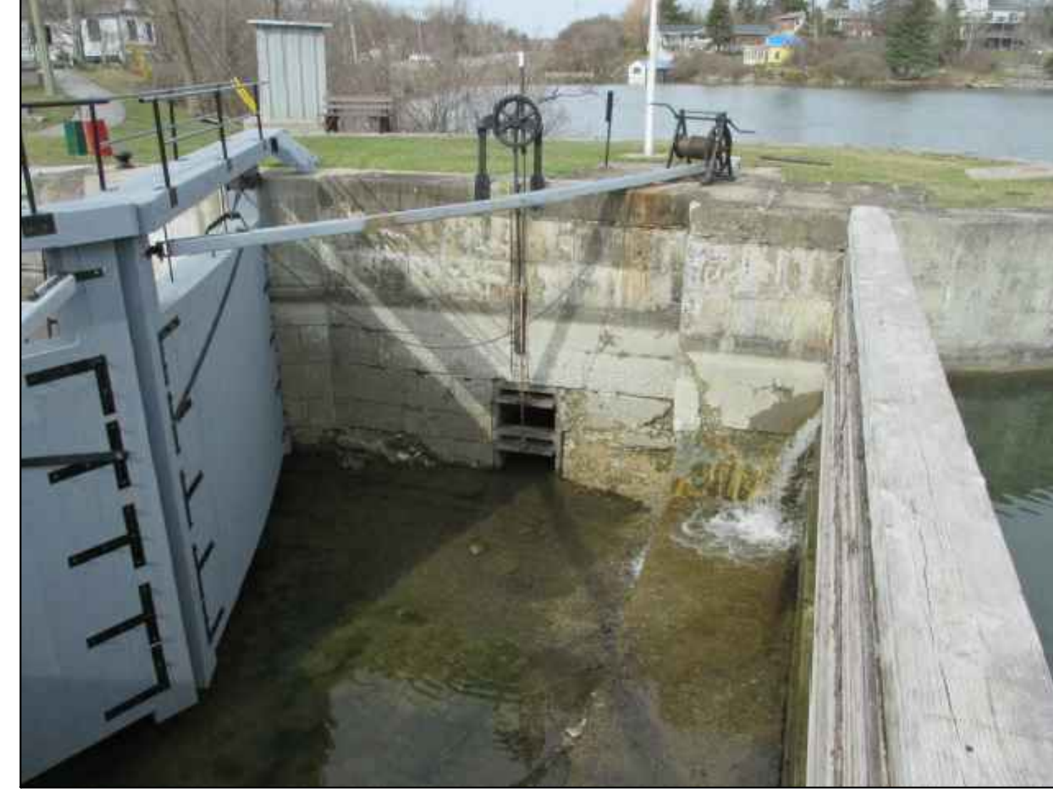
WEST UPPER GATE WALL
