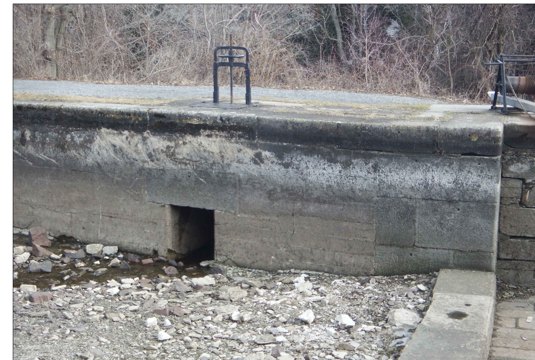
EAST BASIN WALL (SOUTH END) - 2017
