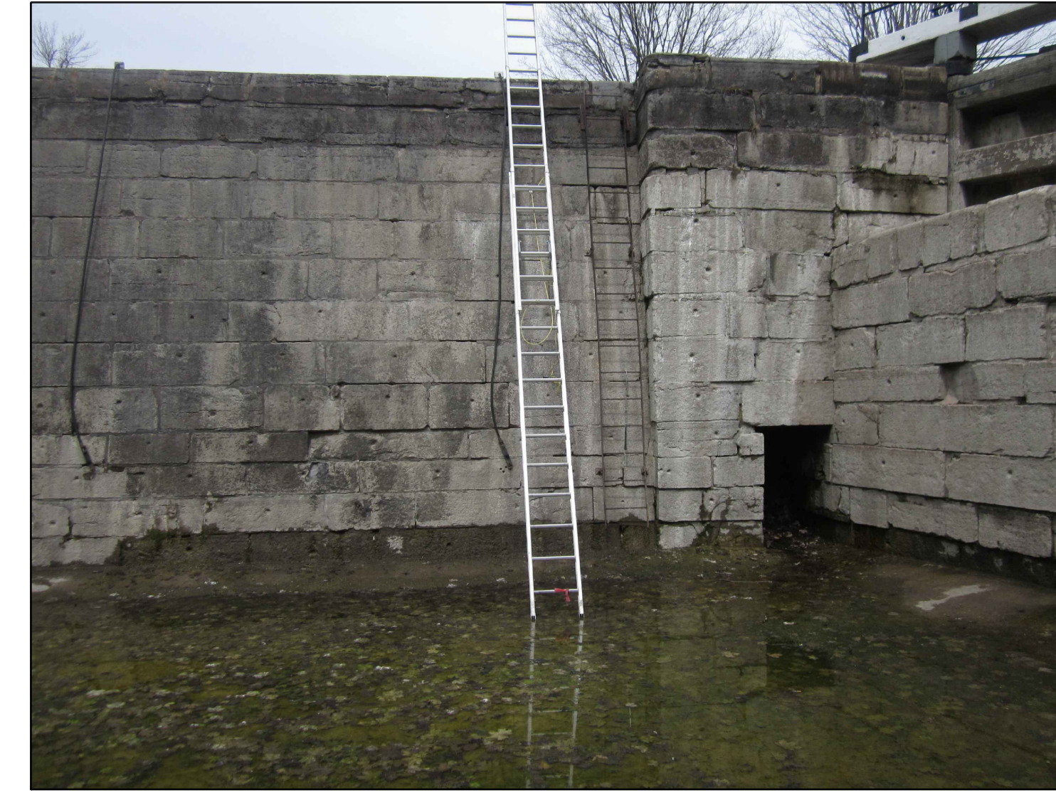
WEST WALL UPPER PIER
