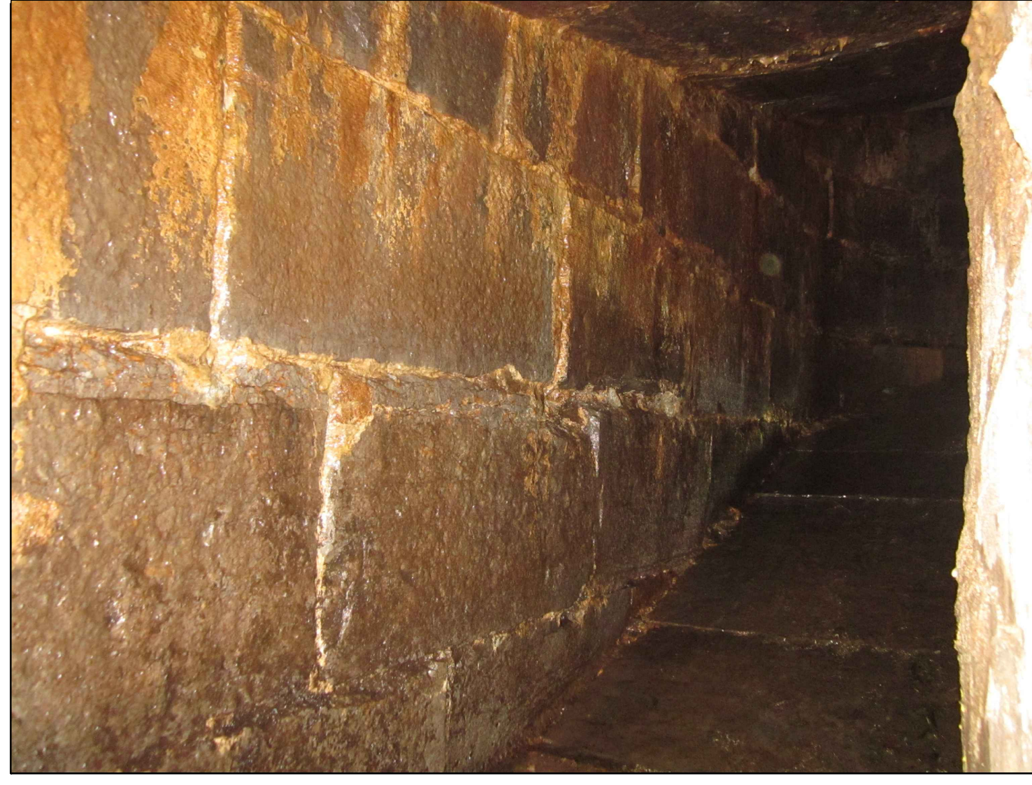
WEST SLUICE TUNNEL LOOKING UP - 2017
