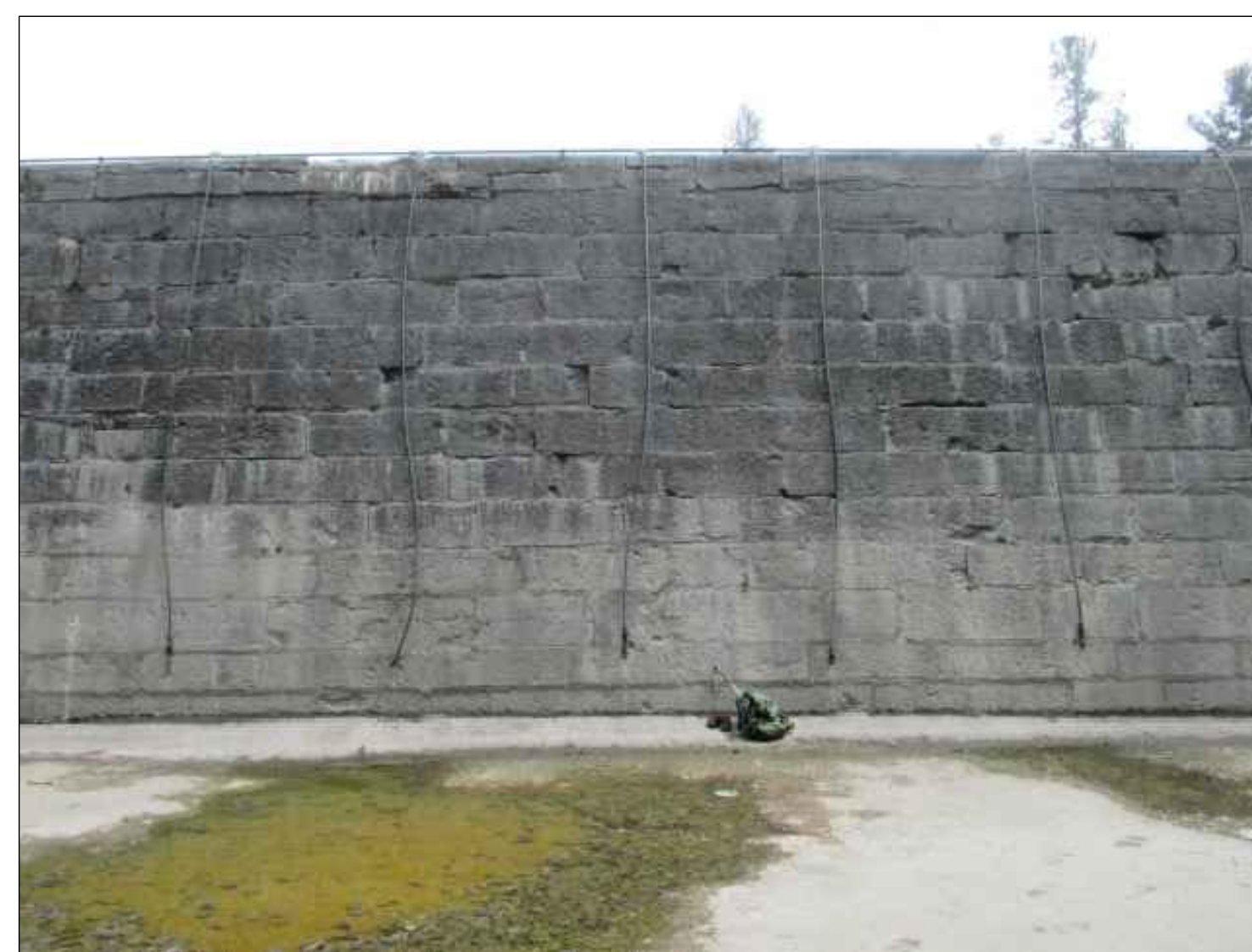
EAST CHAMBER WALL
