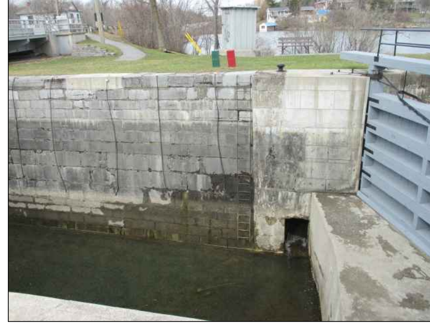
WEST WALL UPPER PIER
