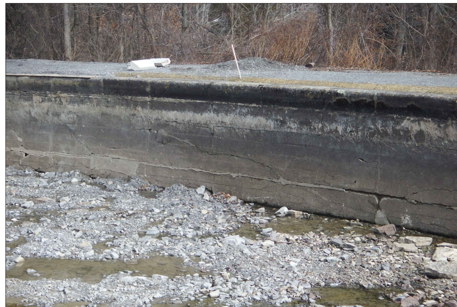
EAST BASIN WALL (CENTER) - 2017
