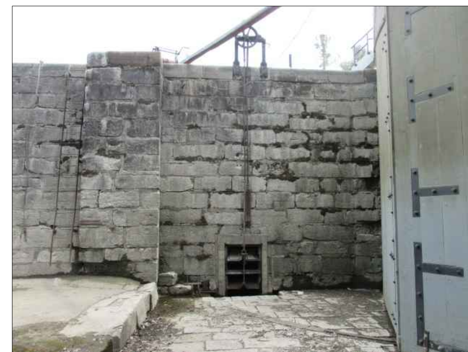
EAST WALL LOWER PIER
