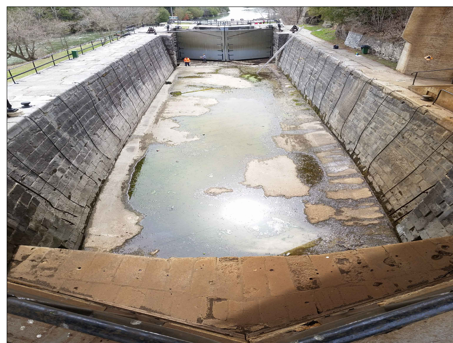
CHAMBER FLOOR (LOOKING SOUTH)
