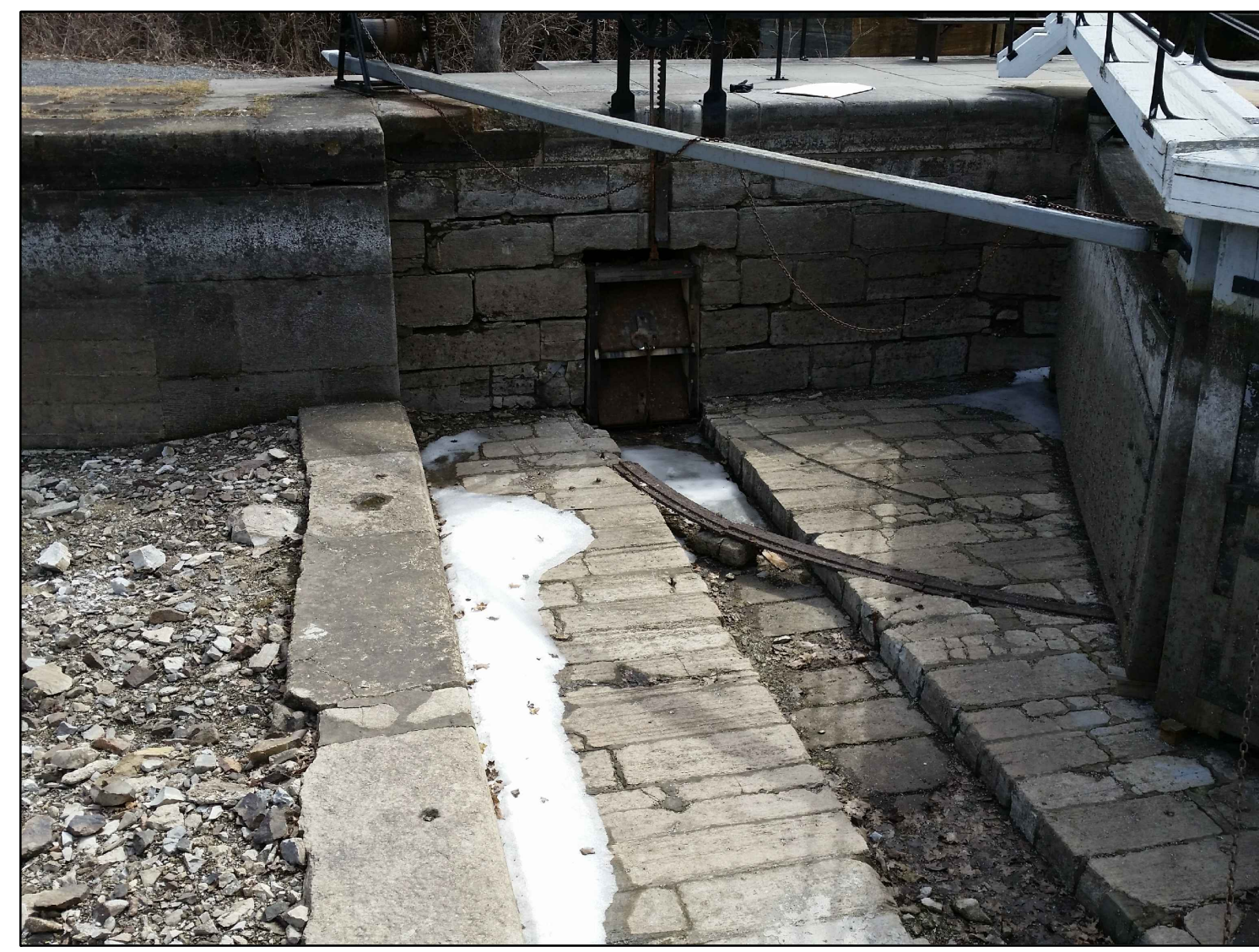
EAST UPPER GATE WALL - 2017
