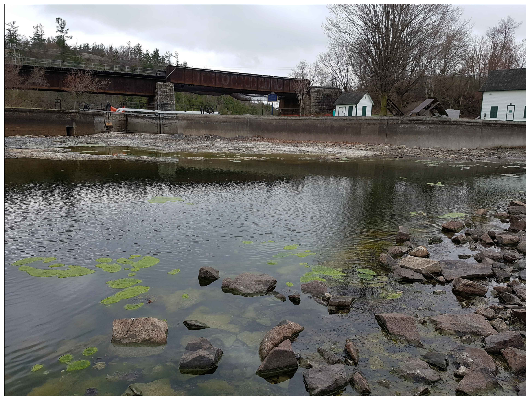
SOUTH BASIN WALL - 2017
