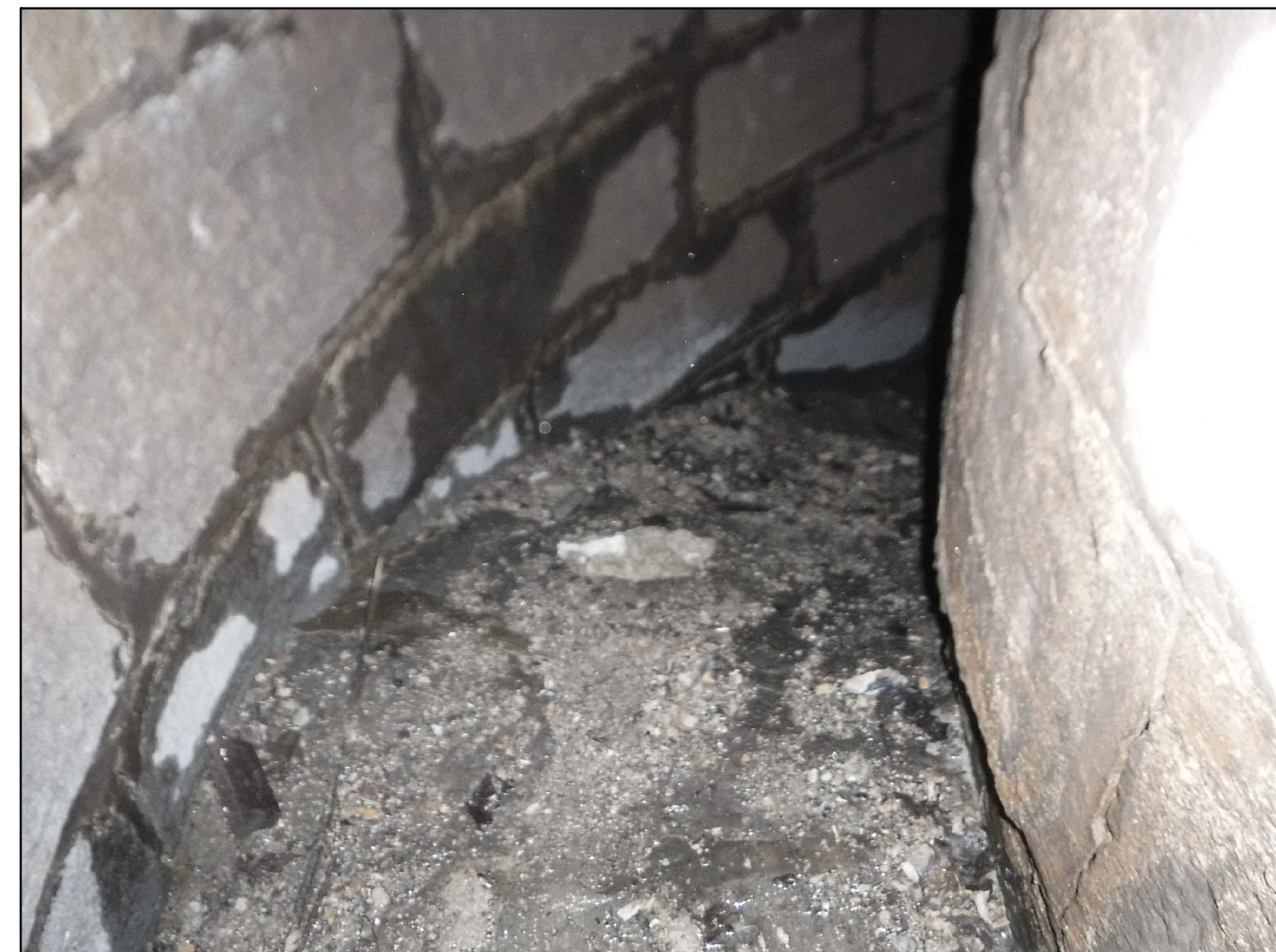
EAST SLUICE TUNNEL LOOKING DOWN - 2017
