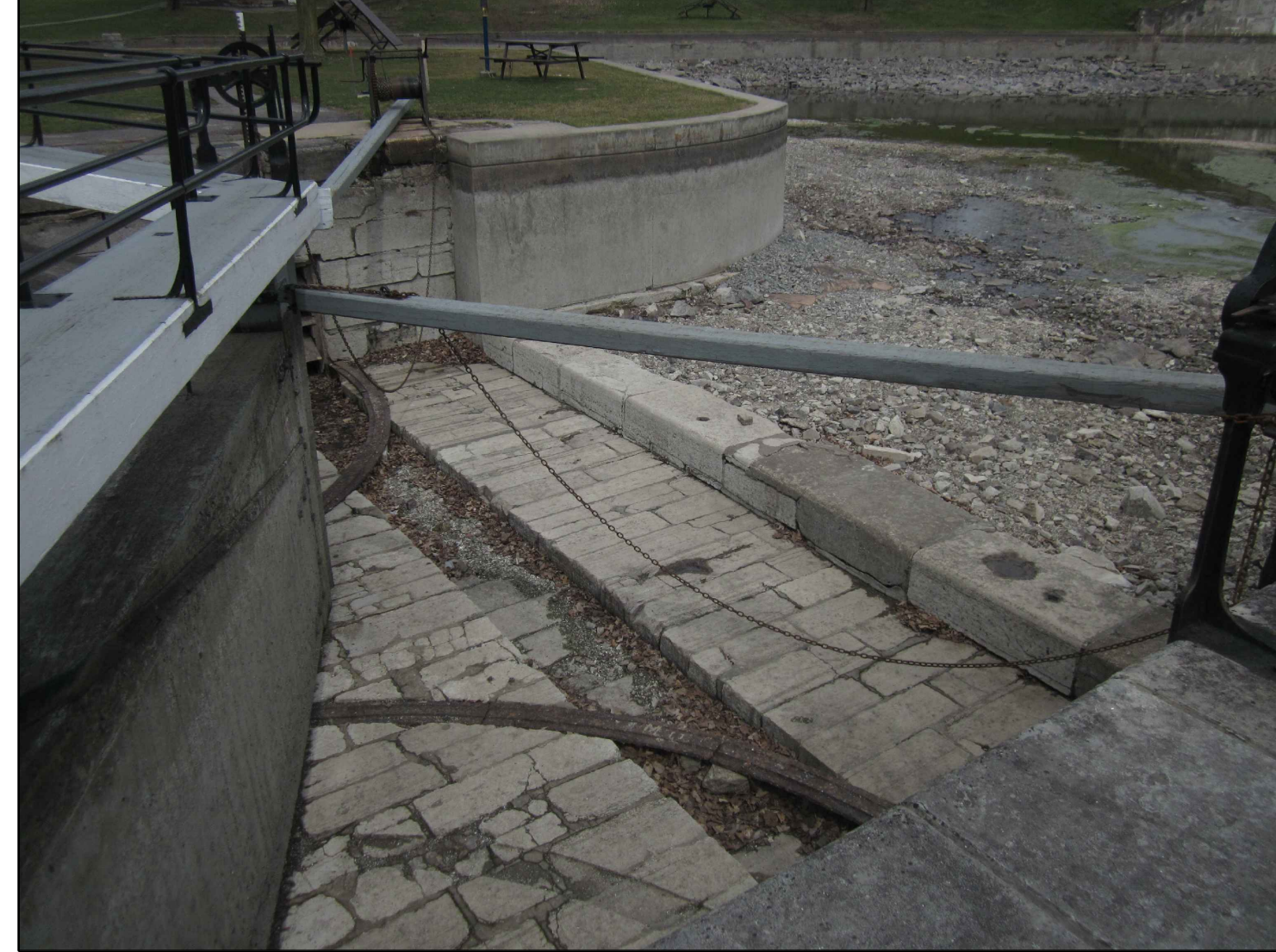
UPPER GATE RECESS FLOOR
