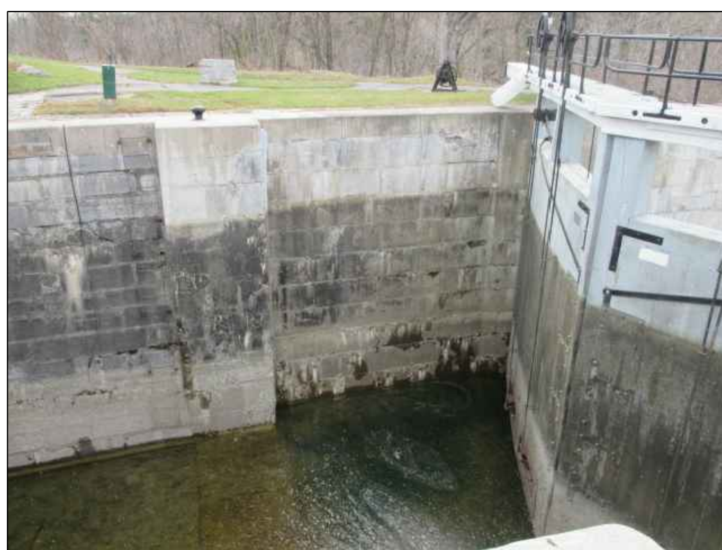
EAST WALL LOWER PIER
