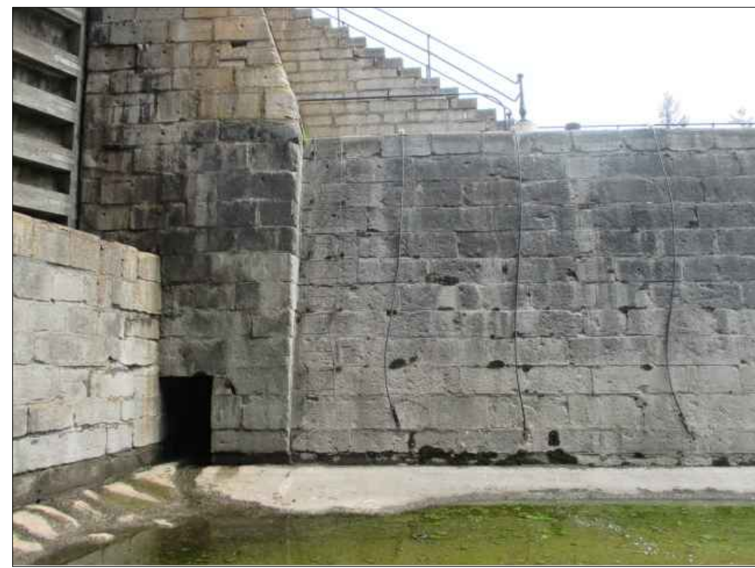
EAST WALL UPPER PIER
