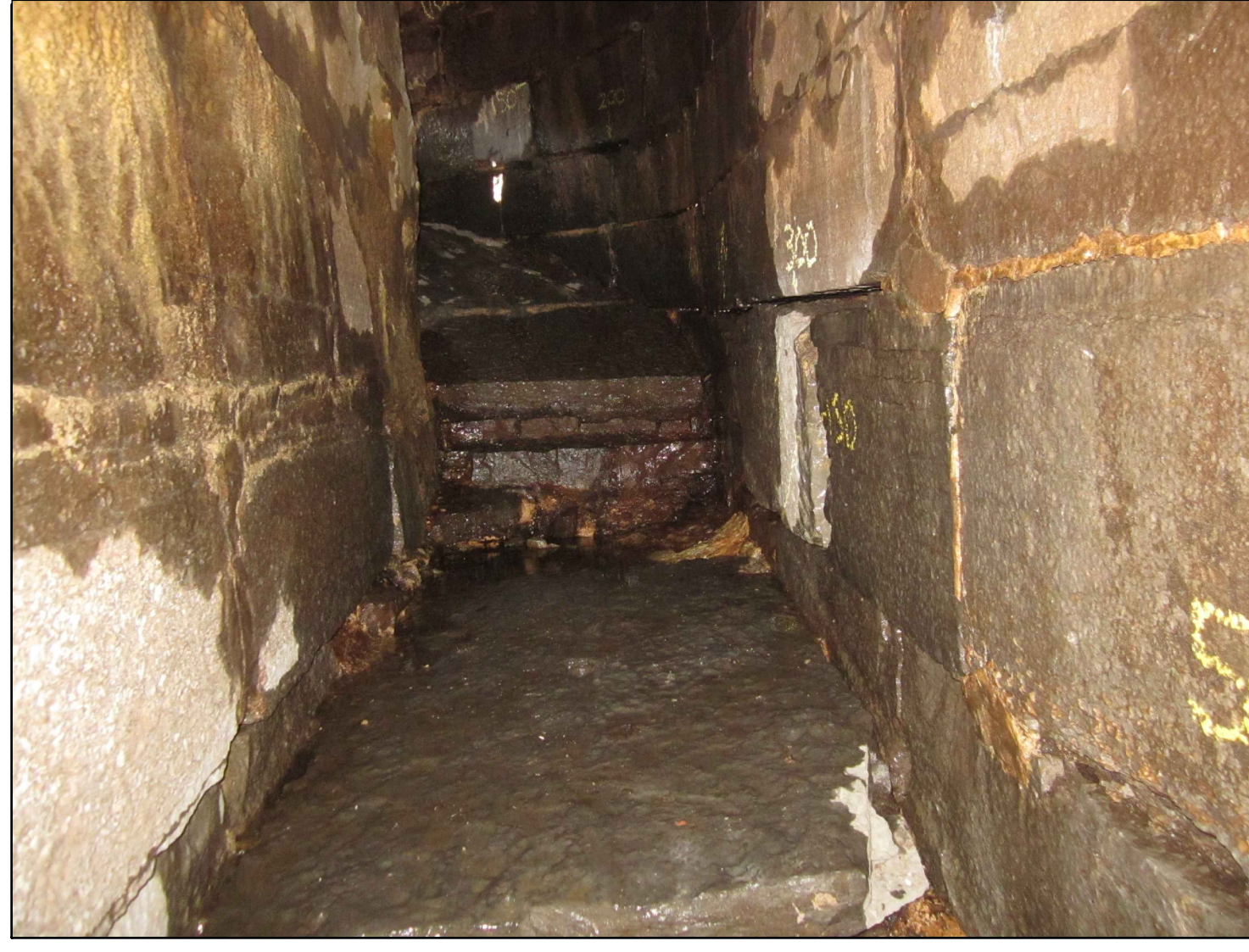
EAST SLUICE TUNNEL LOOKING UP - 2017
