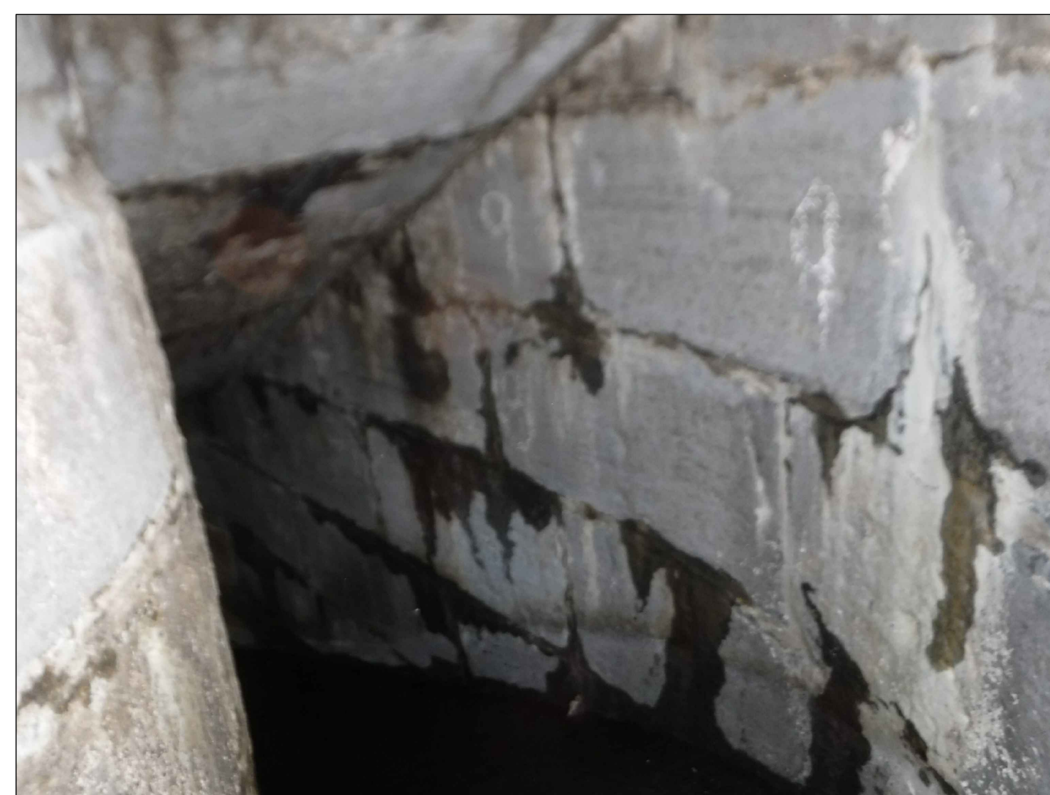
WEST SLUICE TUNNEL LOOKING DOWN - 2017
