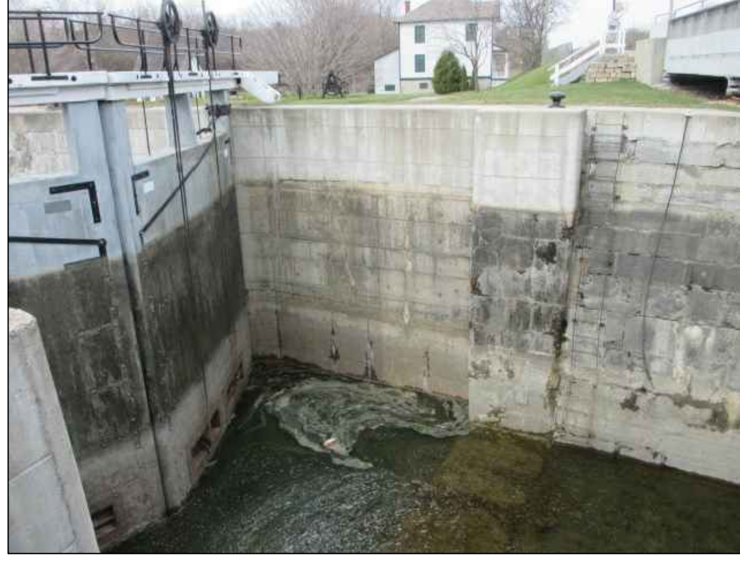
WEST WALL LOWER PIER
