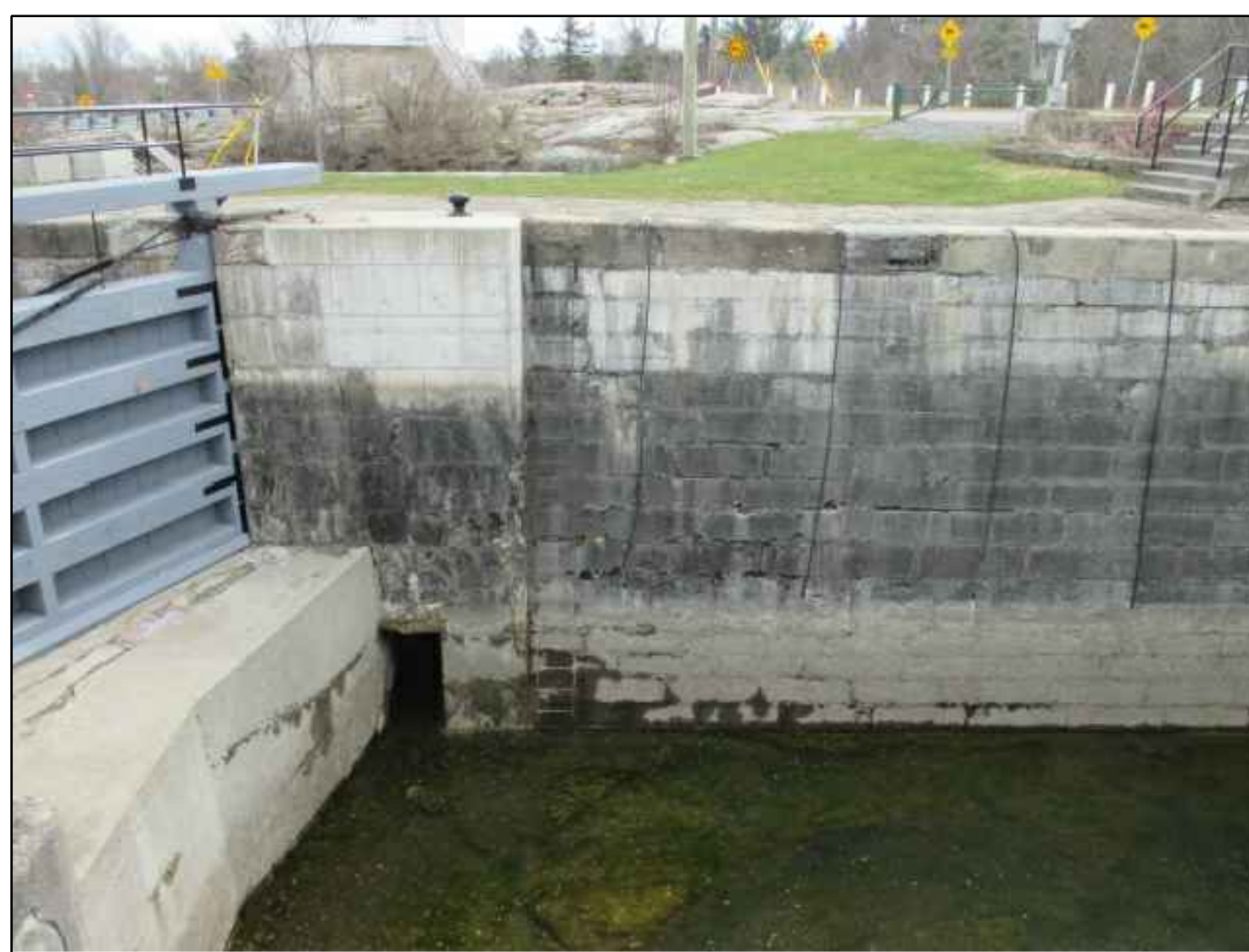
EAST WALL UPPER PIER
