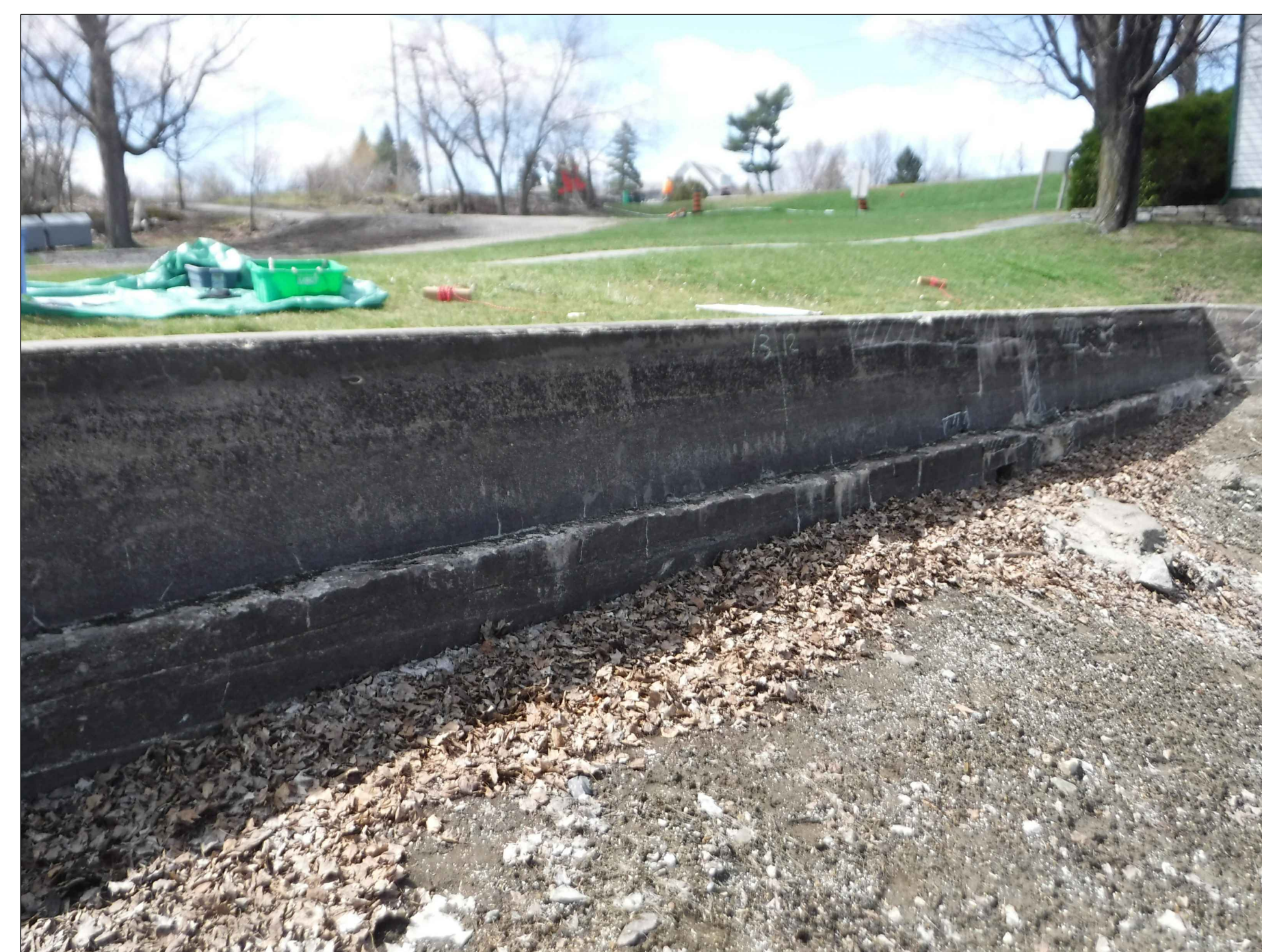
WEST BASIN WALL - 2017
