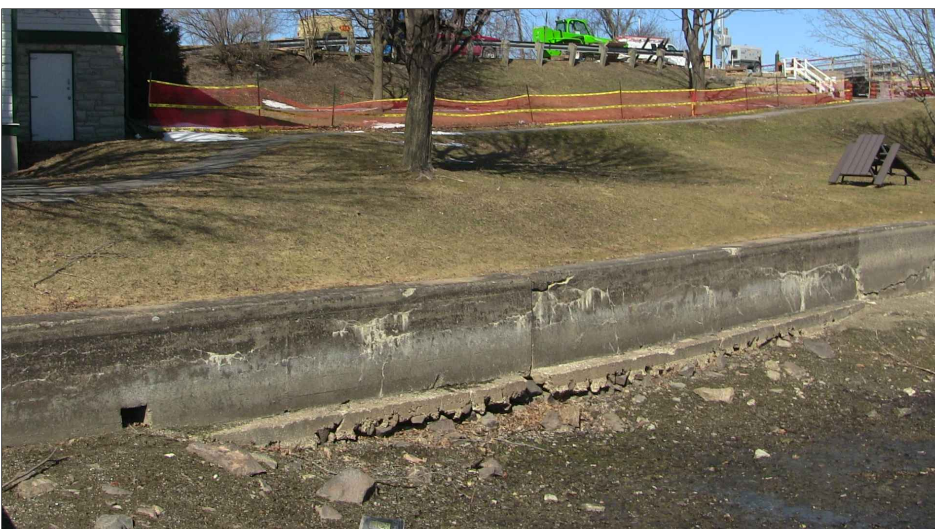
NORTH BASIN WALL (WEST END) - 2017
