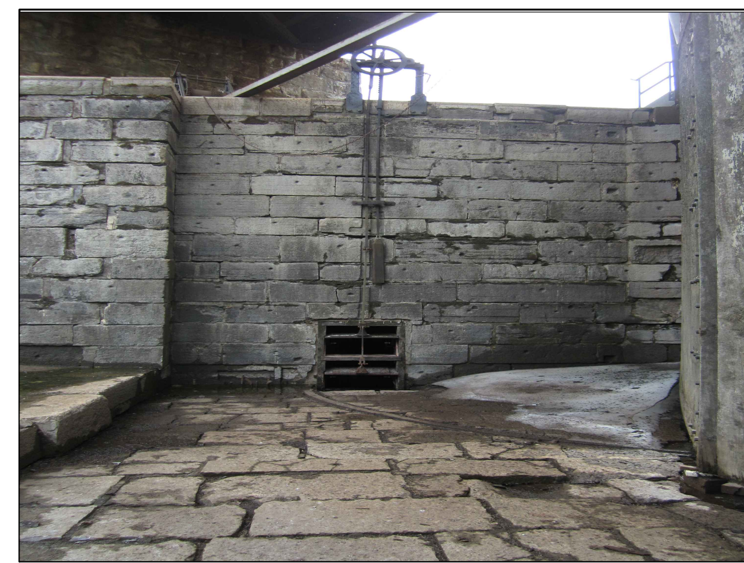
EAST WALL LOWER PIER
