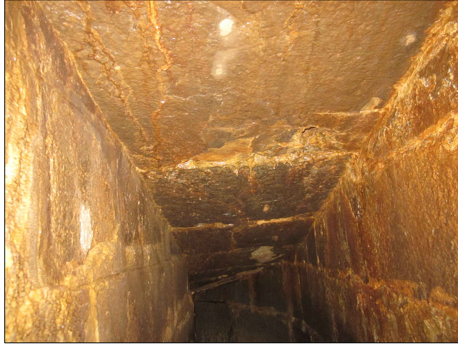
WEST SLUICE TUNNEL LOOKING DOWN - 2017
