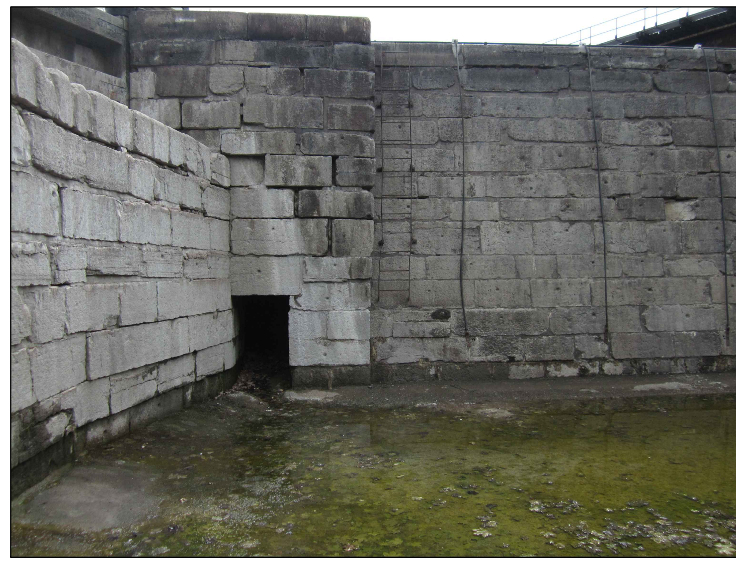
EAST WALL UPPER PIER
