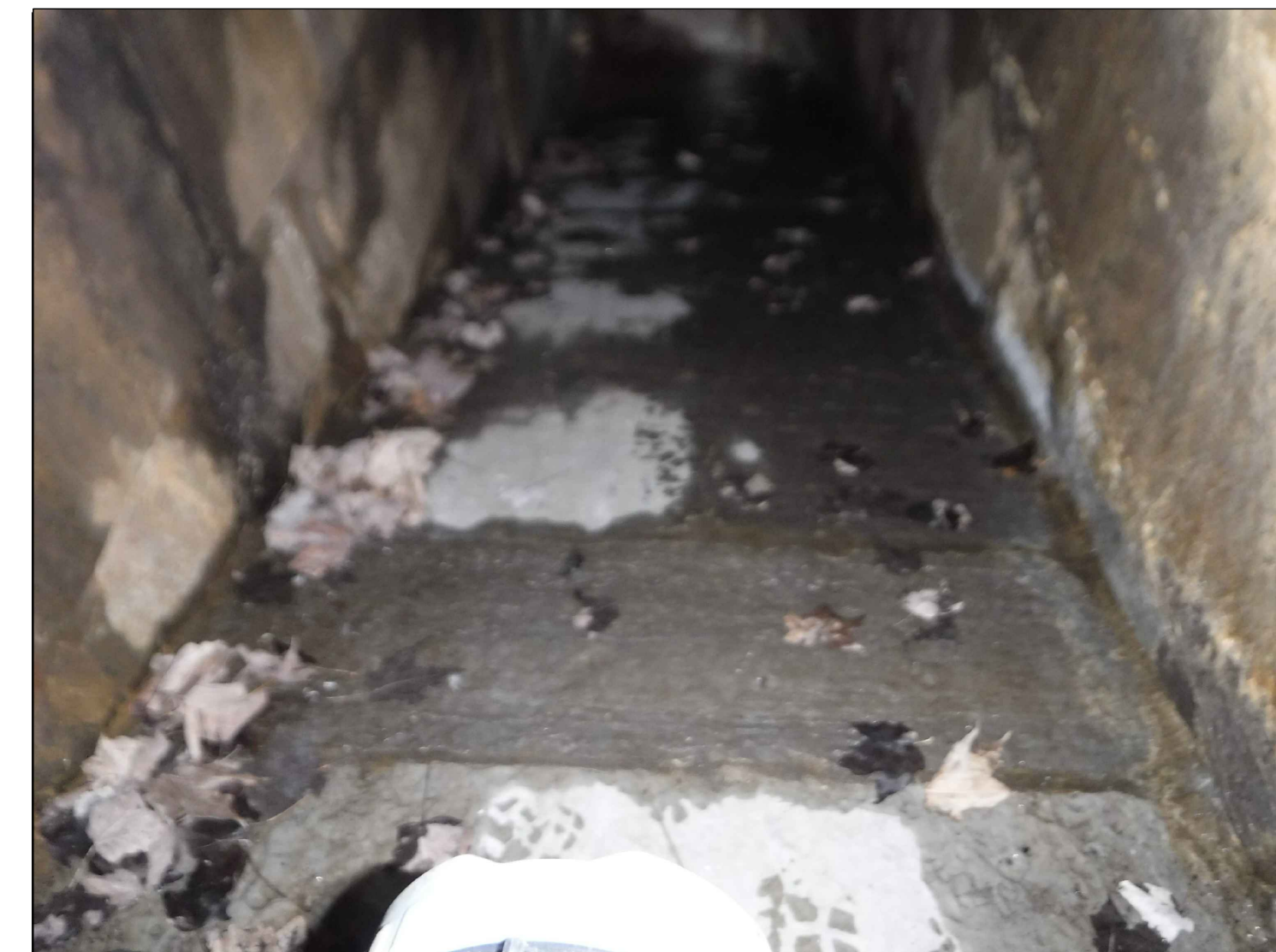
WEST SLUICE TUNNEL LOOKING UP - 2017
