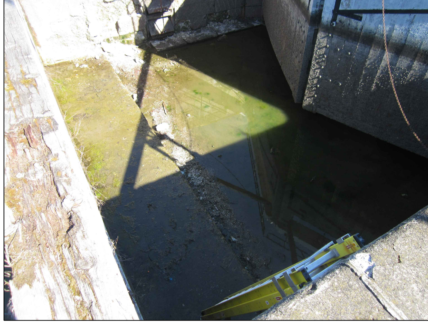
UPPER GATE RECESS FLOOR
