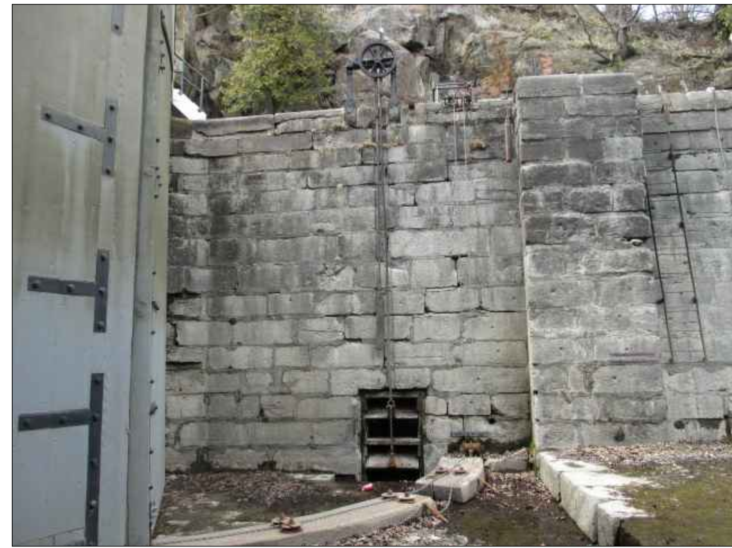
WEST WALL LOWER PIER
