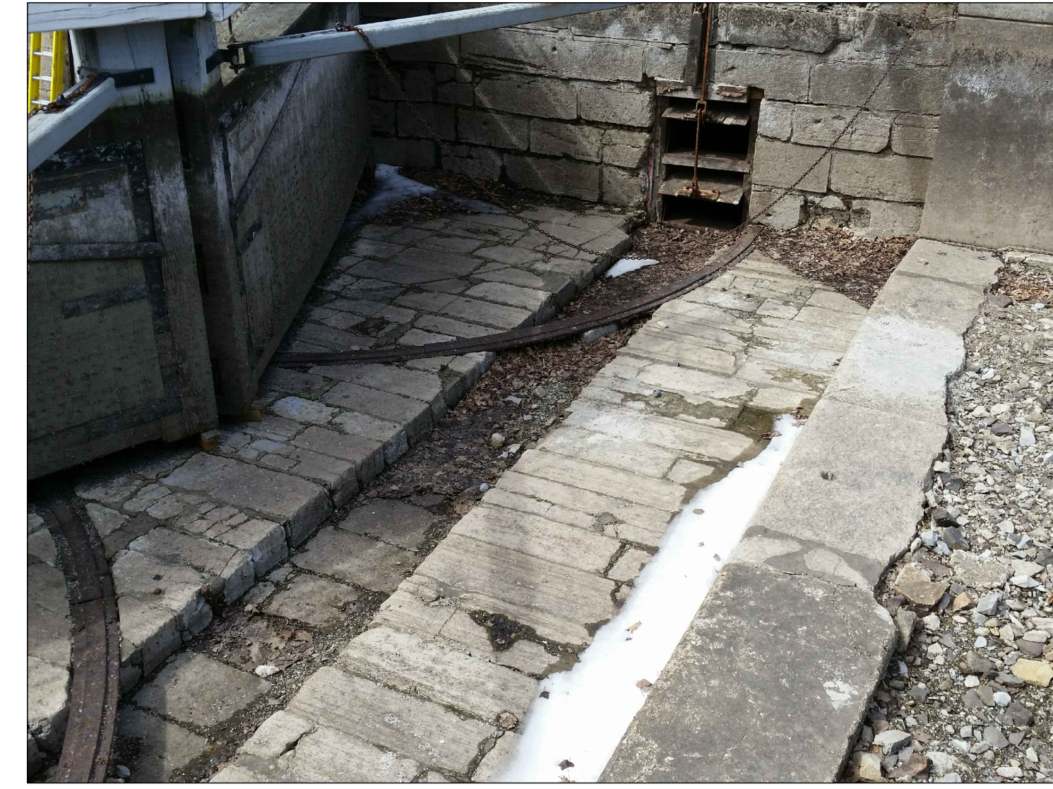
WEST UPPER GATE WALL - 2017
