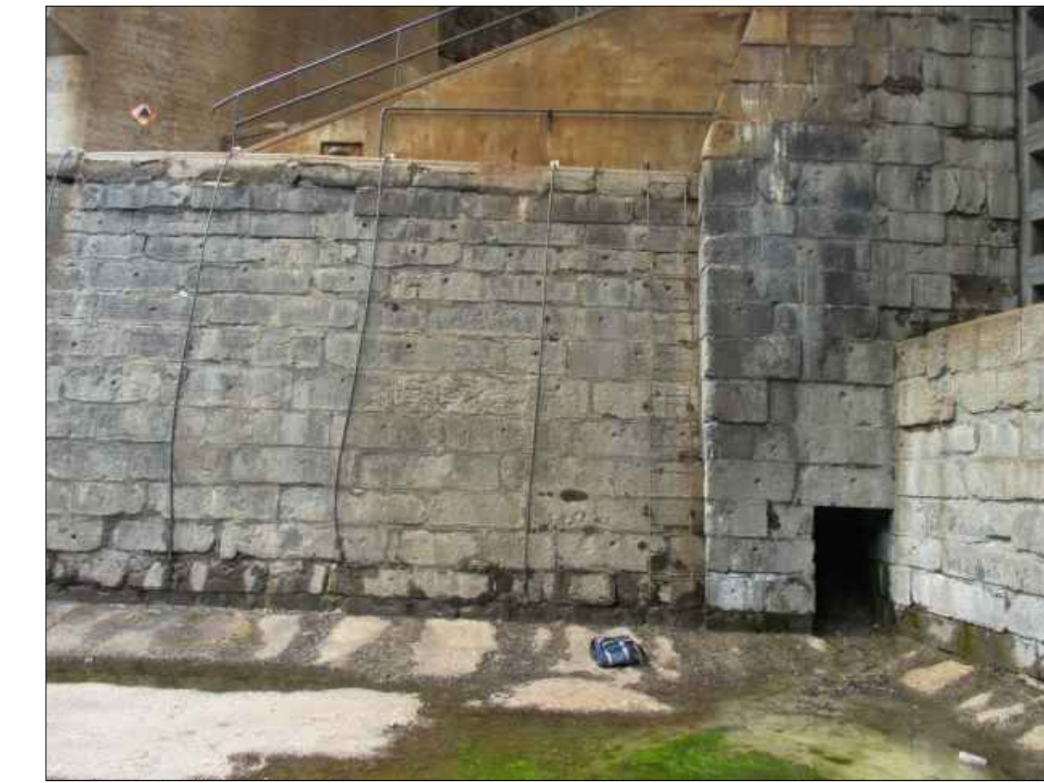
WEST WALL UPPER PIER
