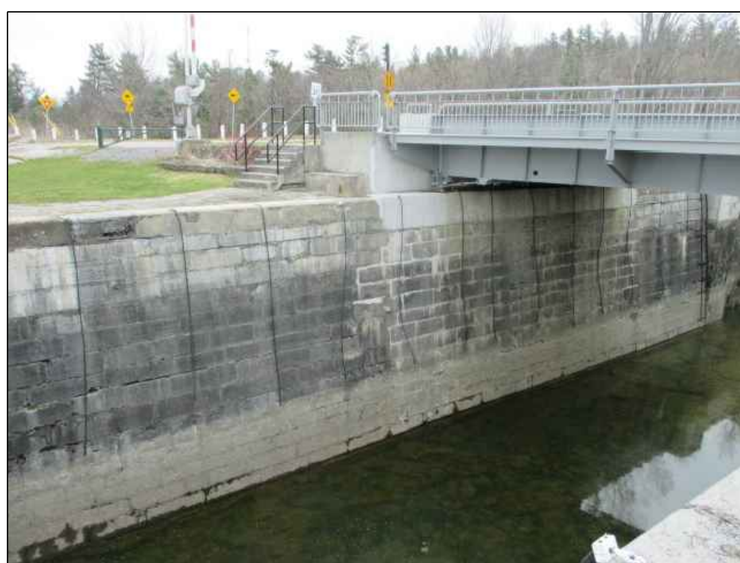
EAST CHAMBER WALL
