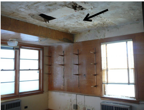
#2 Administration Office – Main Floor Water damage and failure of the main floor ceiling
