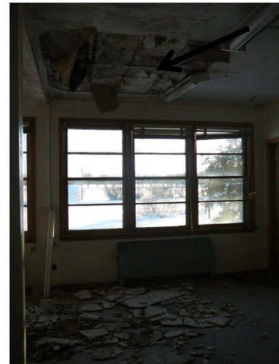
#2 Administration Office – 2 nd Floor Water Damage and debris from failure of the 2 nd floor ceiling
