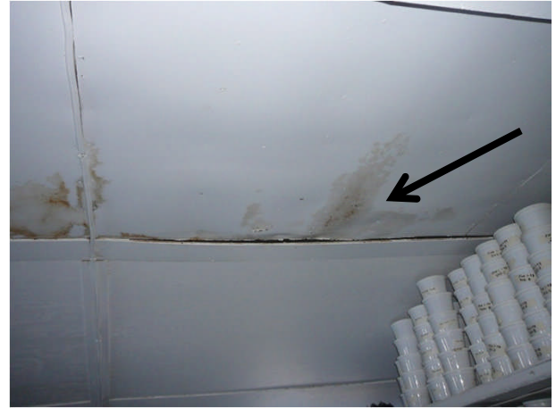
#14 Drying and Threshing Shed Water damaged ceiling
