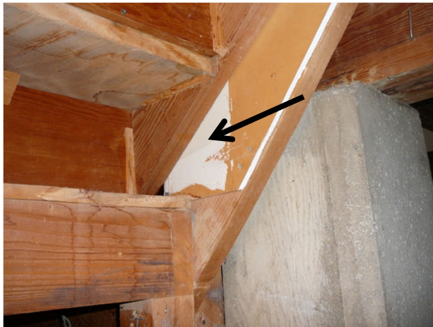
#60 Duplex House Sample A15 : Drywall mud containing asbestos
