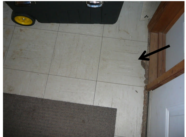
#60 Duplex House Sample A17 : Floor tile containing asbestos
