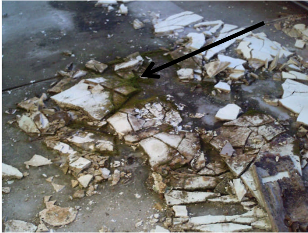
#2 Administration Office – 2 nd Floor Ceiling material on the floor with biological growth
