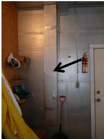
#33 Processing and Carpenter Shop Sample A1 : Duct insulation containing asbestos
