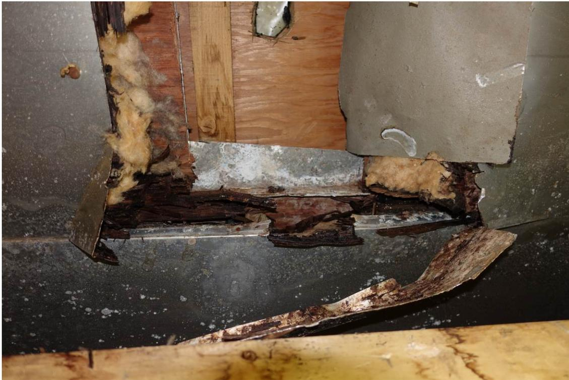
**Photograph 9.** View of rotted wood and mould-contamination in the attic space.
