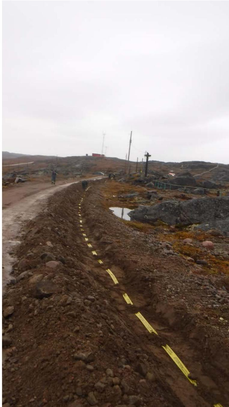
**Figure 6: Trench containing existing power cable**
