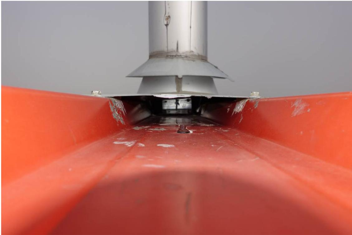
**Photograph 5.** View of the base of flue vent showing underlying cavity.
