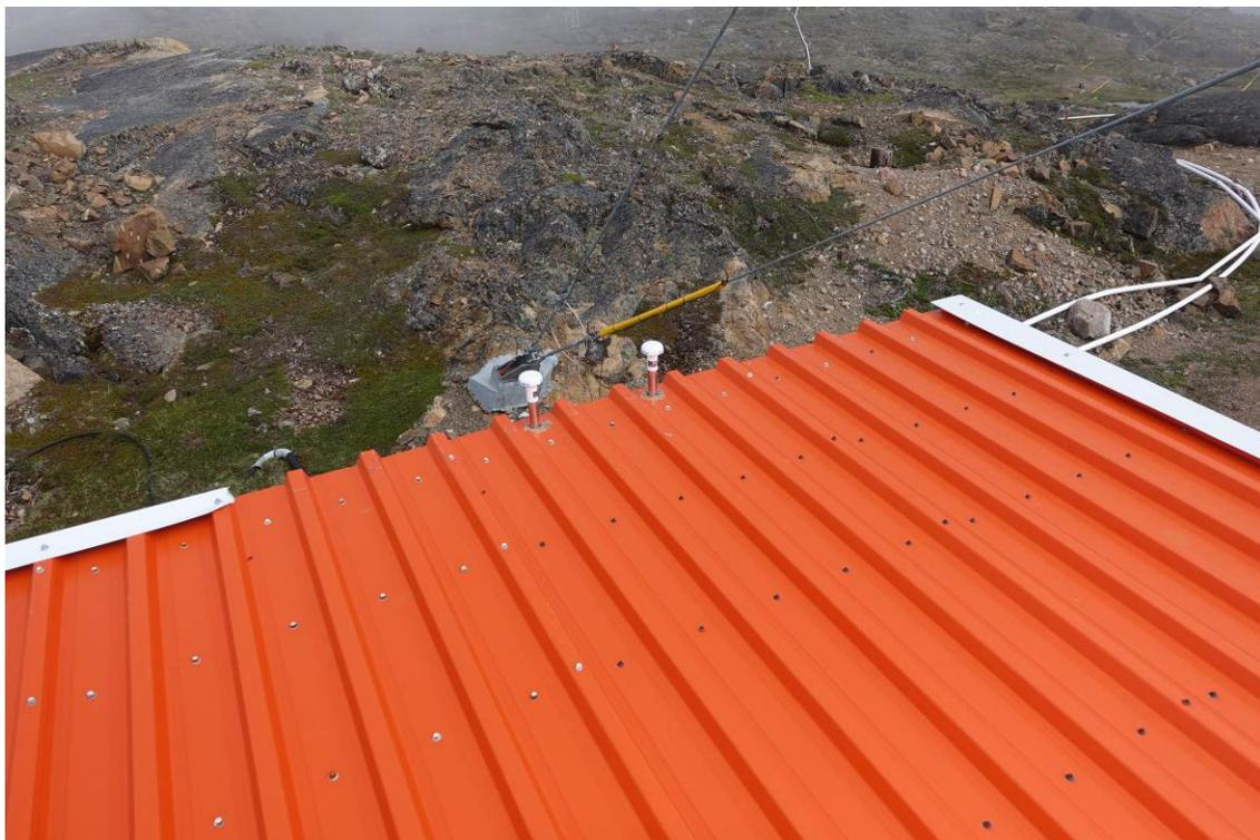
**Photograph 2.** View of the northeast corner of metal batten roof with flashing removed.
