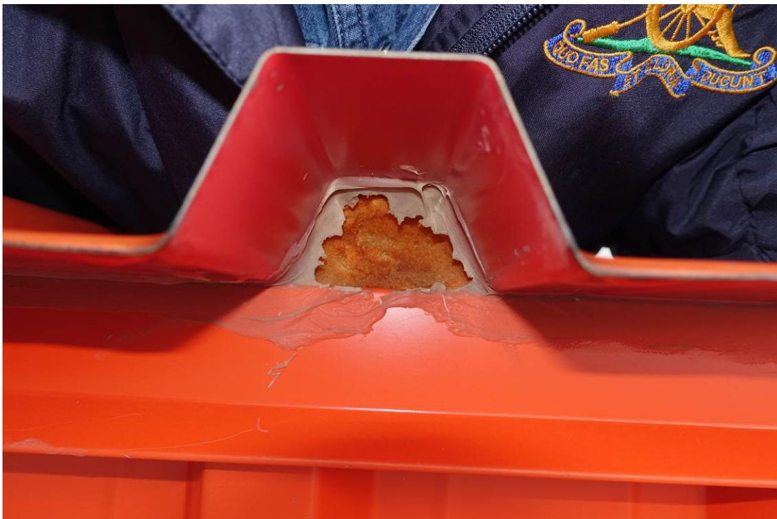
**Photograph 4.** View of deteriorating sealant and insulation in flute opening of roof.
