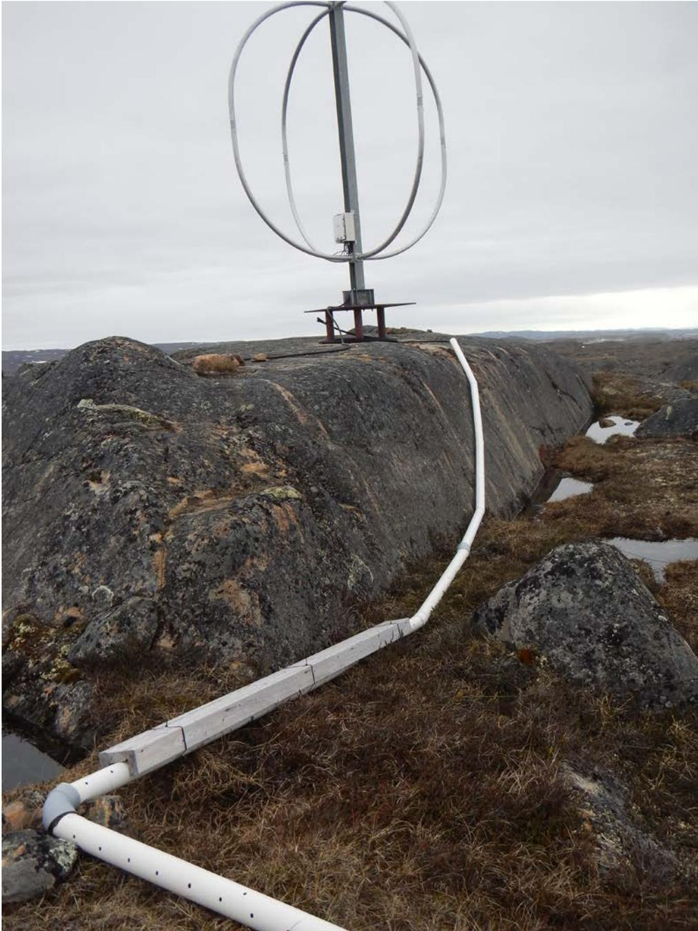
**Figure 5: Existing conduit, note drain holes**
