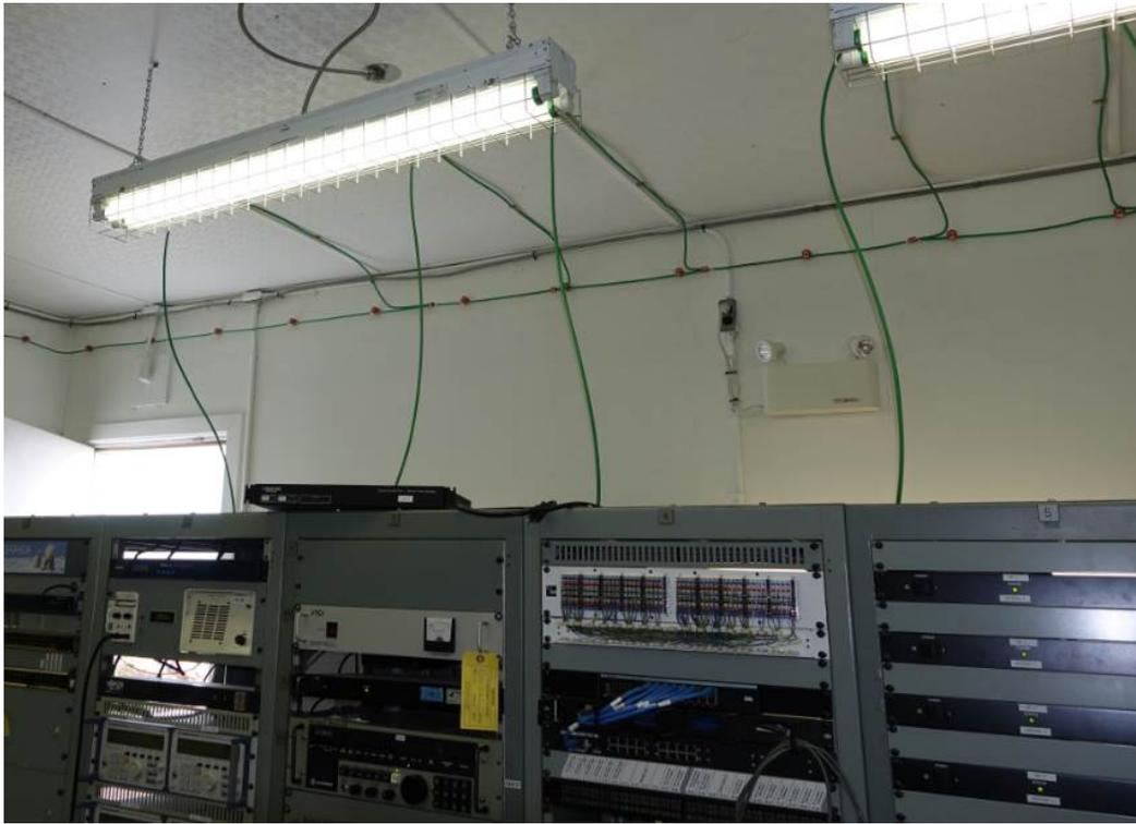
**Photograph 11.** View of the generator room showing emergency lighting and fluorescent light tubes with potentially PCB containing ballasts.
