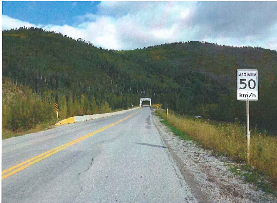
P03 - General view of S approach facing bridge
