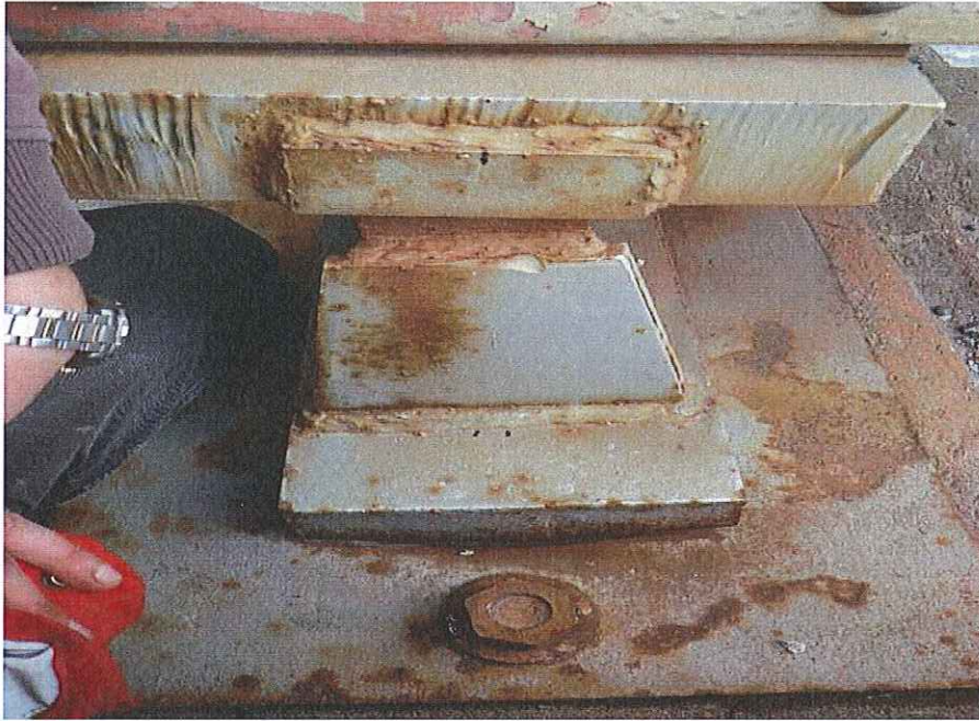
P45 - W truss bearing at N Pier facing E
