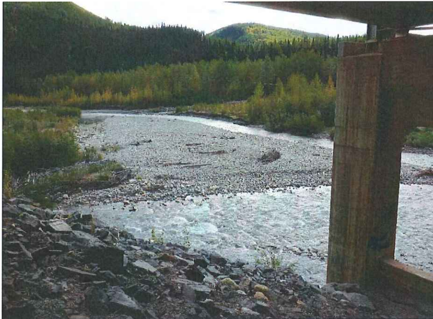
P07 - Downstream channel facing SE from embankment beneath N Abutment
