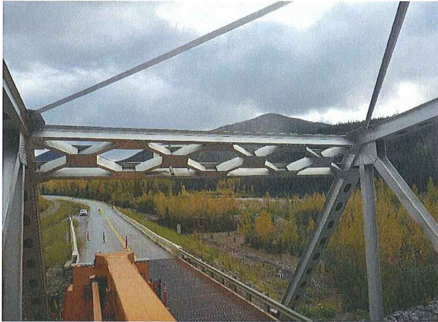
P13 - S truss portal frame facing S
