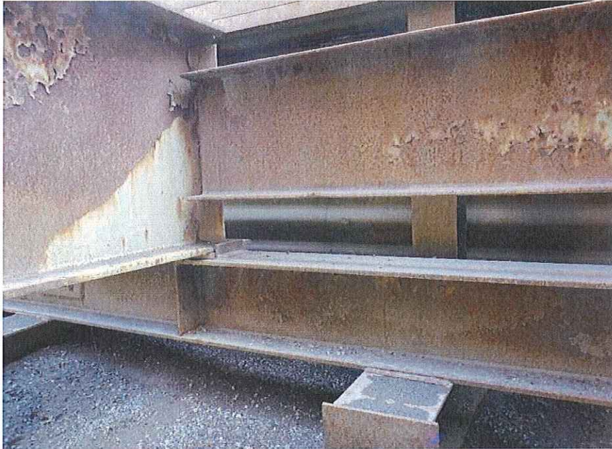
P17 - Typical bearing at S Abutment
