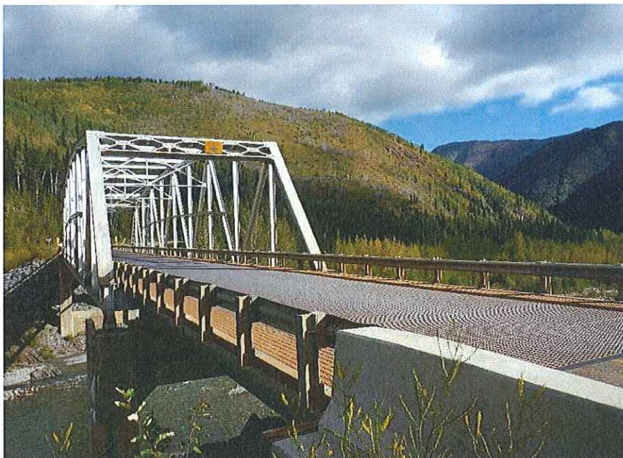
P02 - Span 1 and S portal of truss facing NE
