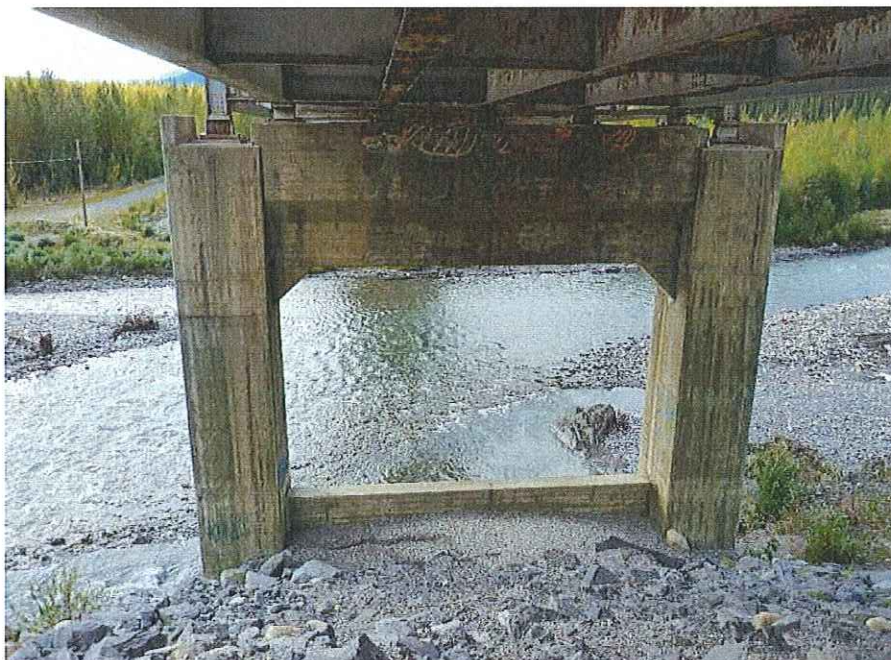
P06 - N Pier facing S
