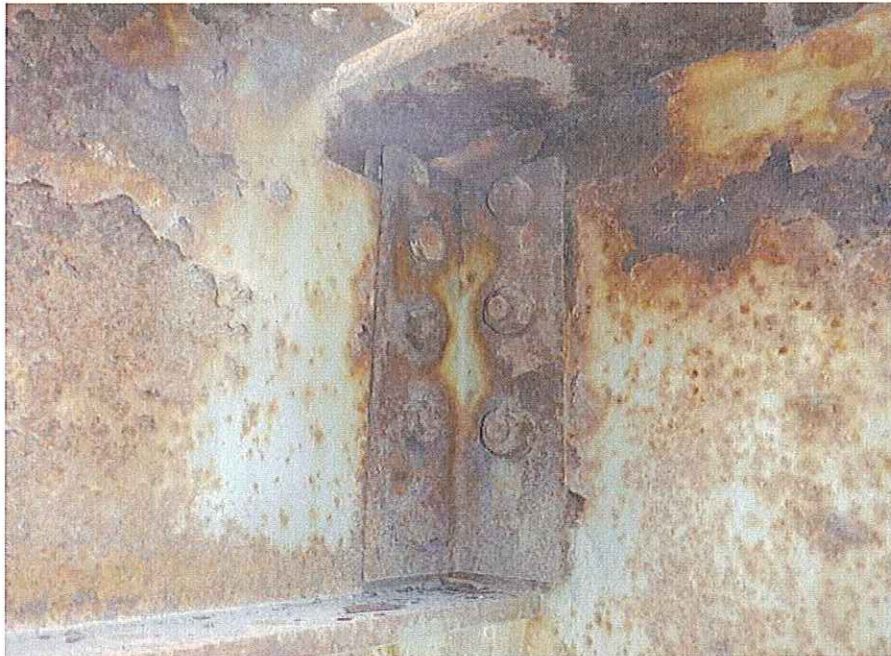
P37 - Typical connection of stringer to floor beam
