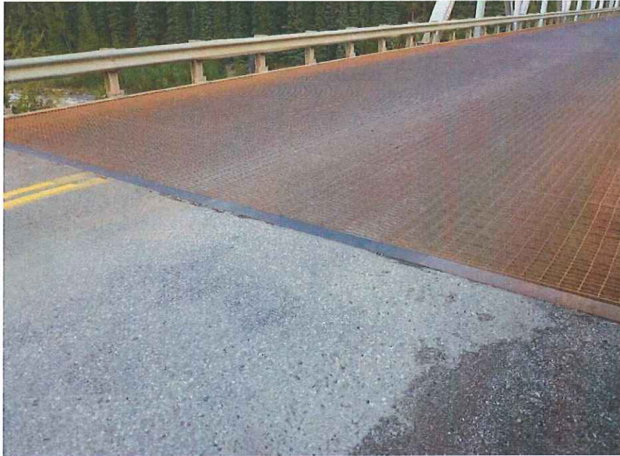
P47 - Deck joint at S Abutment
