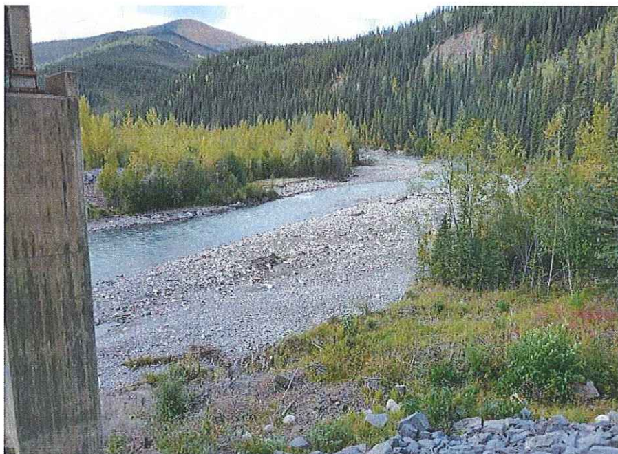
P14 - Upstream view facing SW from N Abutment
