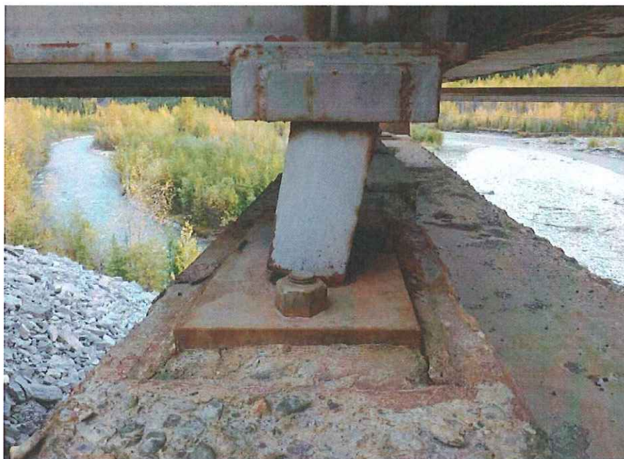
P44 - Typical rocker bearing for Span 3 girder at N Pier
