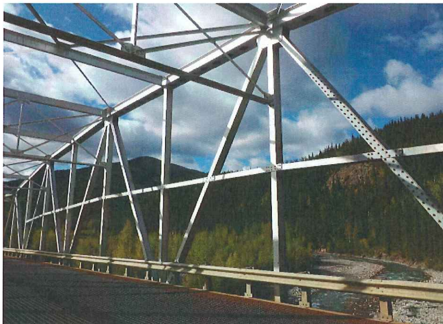
P04 - W truss facing SW from near midspan
