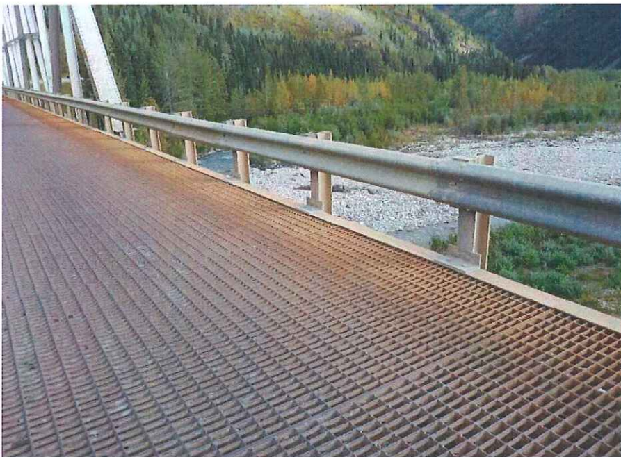
P52 - Typical bridge barrier
