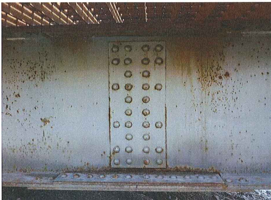
P38 - Typical girder splice on Span 3
