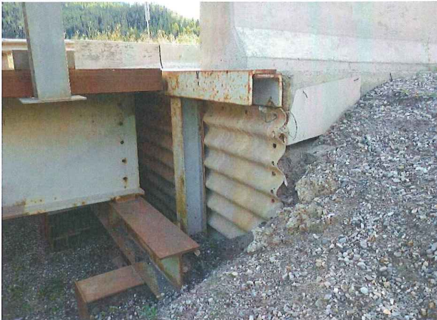
P16 - General view of S Abutment facing E
