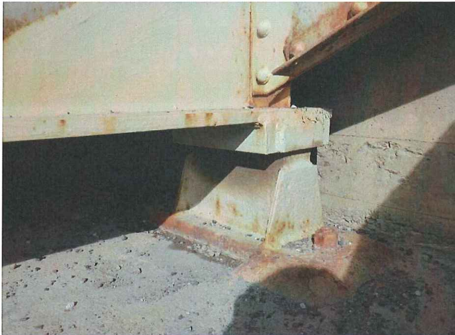
P43 - Typical fixed girder bearing at N Abutment
