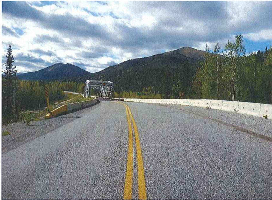
P49 - General view of bridge from N approach facing SW
