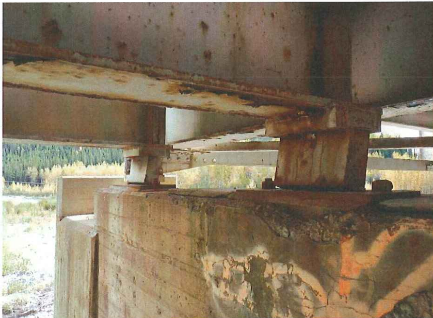
P24 - Span 3 girder bearings at E end of N Pier
