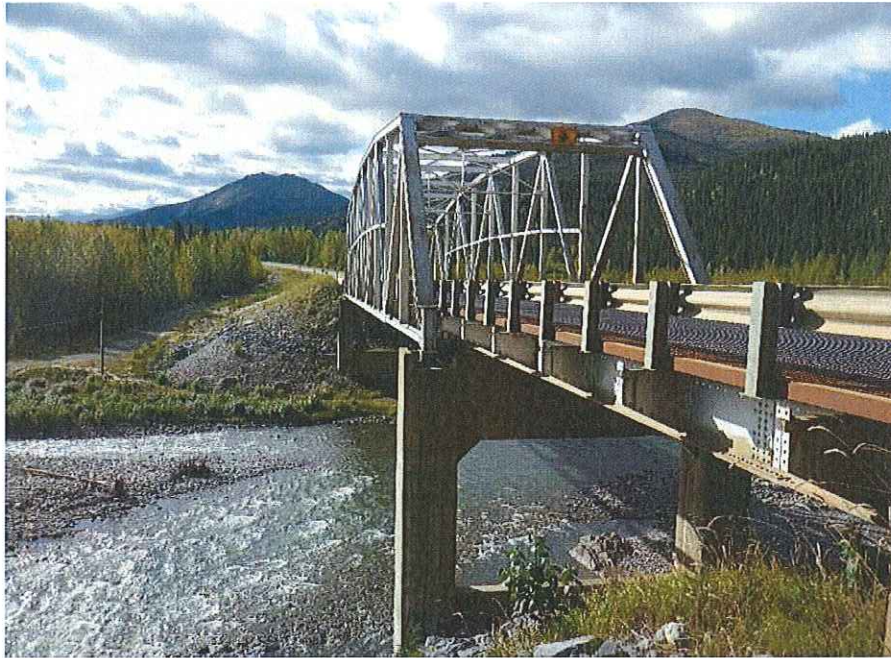
P05 - General view of bridge facing S from W side of N Abutment
