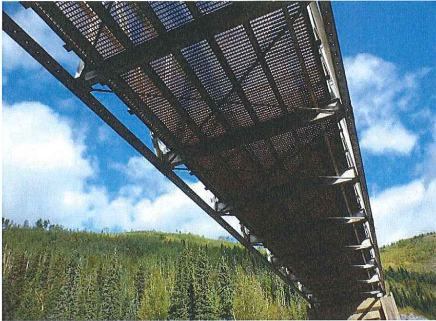
P01 - General view of Span 2 superstructure from stream bank
