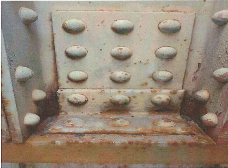
P31 - W truss end post at N pier facing S
