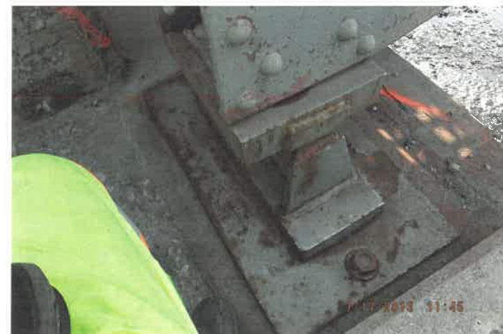
TYPICAL ROCKER BEARING
