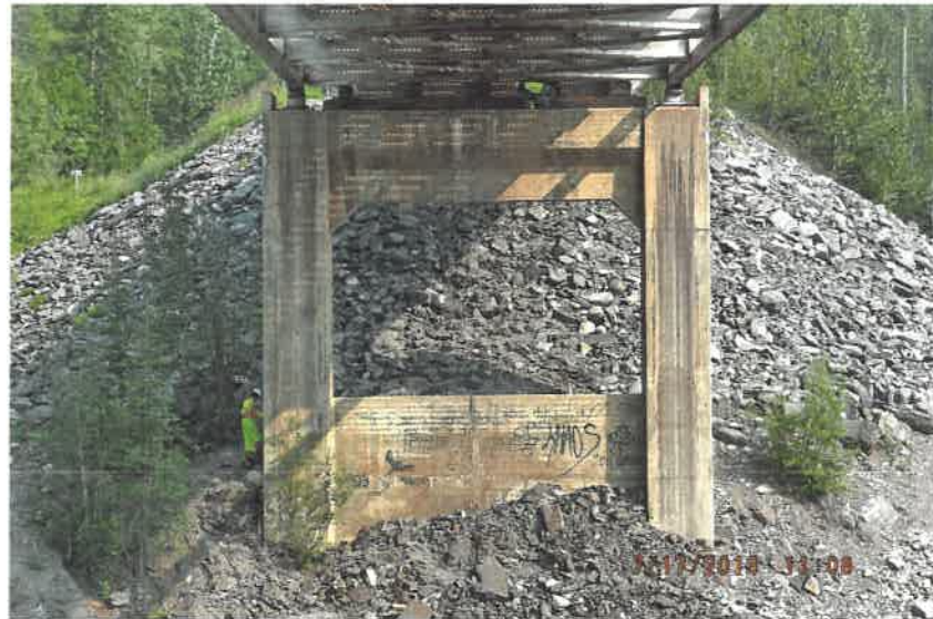
PIER 3 - SOUTH FACE
