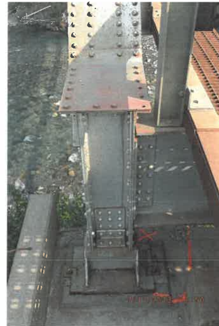
TYPICAL VERTICAL END POST
