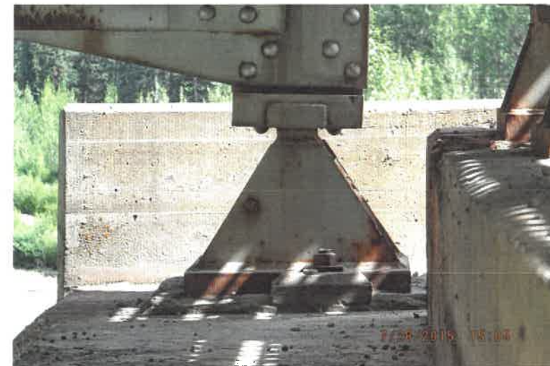
TYPICAL FIXED BEARING
