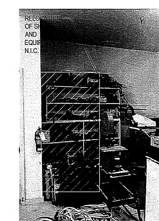
LOCATION FOR ELECTRICAL CLOSET IN MAINTENANCE WORK SHOP.
