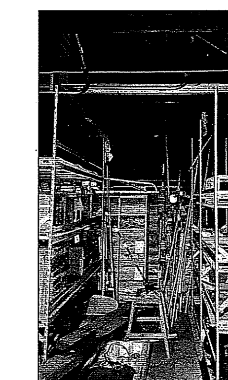
V1 - VIEW OF EXISTING MEZZANINE STORAGE AREA WHERE REMOTE VALVE ROOM IS TO BE LOCATED.
