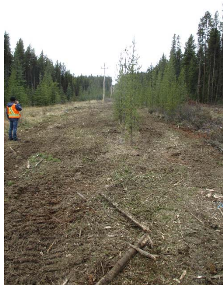
Debris/Mulch/Chipping acceptable volume this photo shows rough mulching (1-2 pass) treatment
