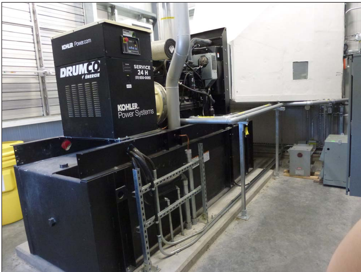
Figure 5: Diesel generator at Latchford Dam
