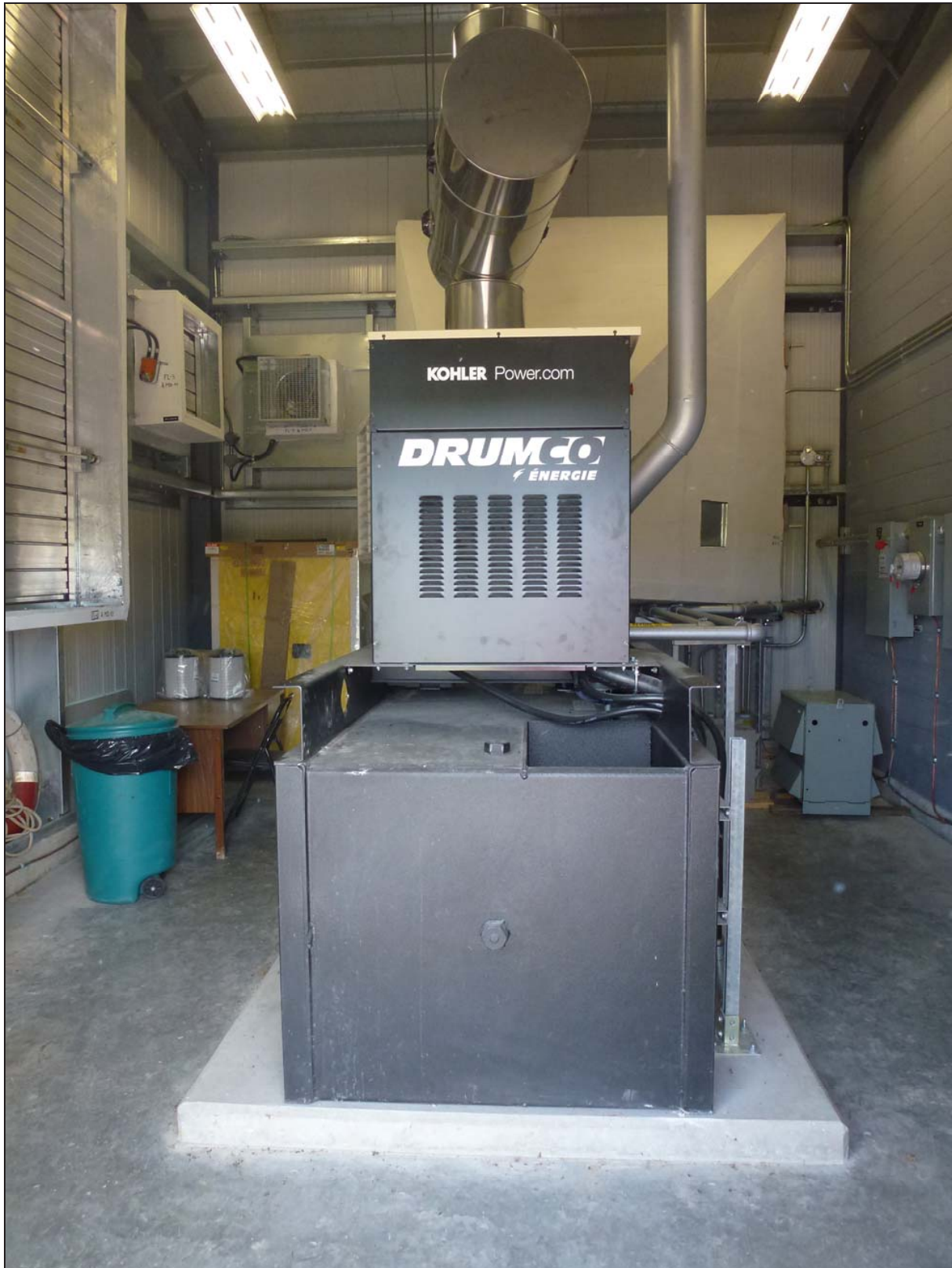
Figure 4: Diesel generator at Latchford Dam
