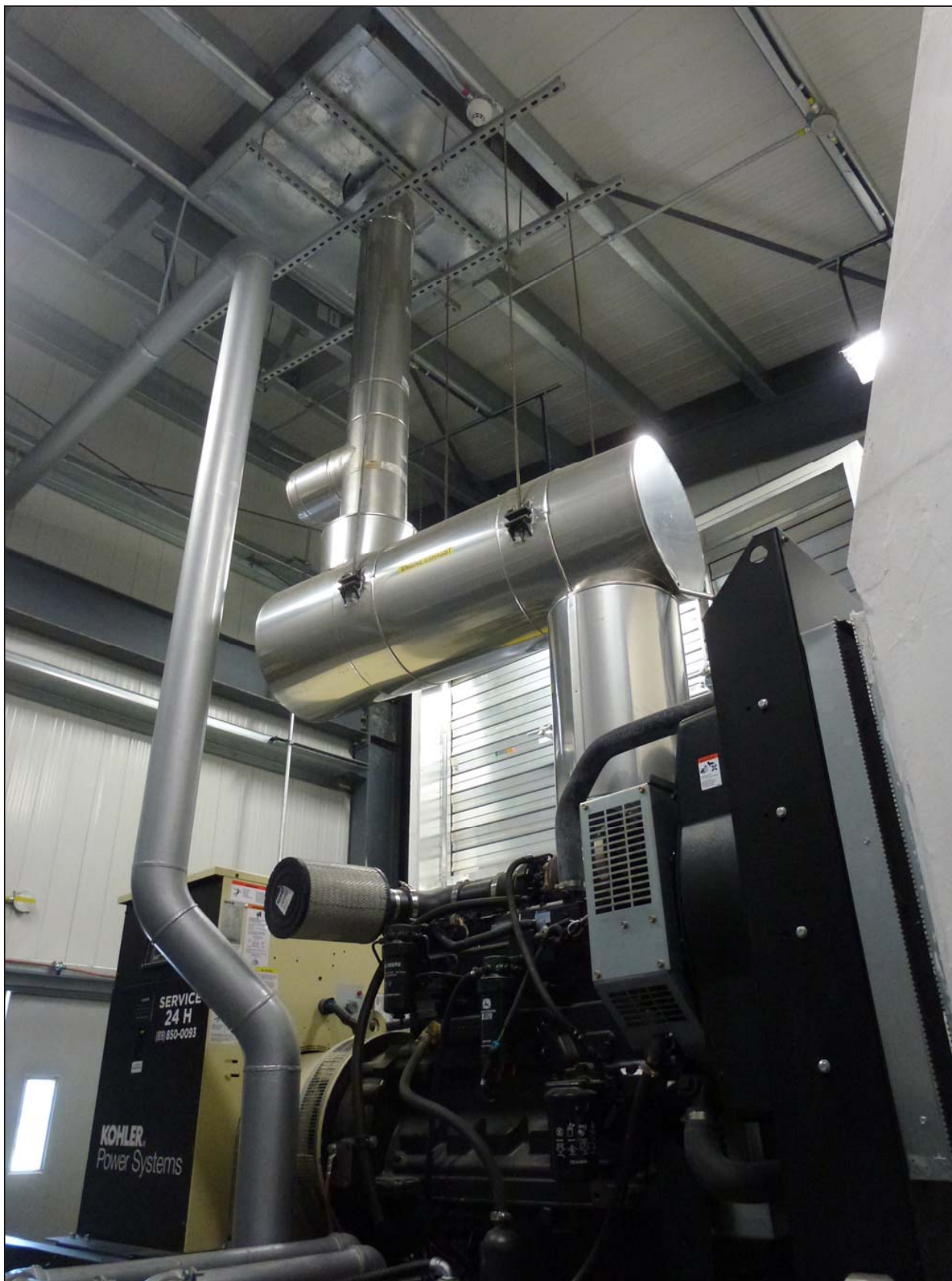
Figure 6: Exhaust piping.
