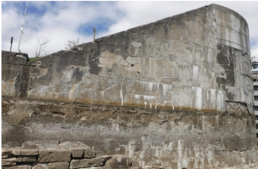
Lock 46 West Side of Lock – Southwest Wing wall
