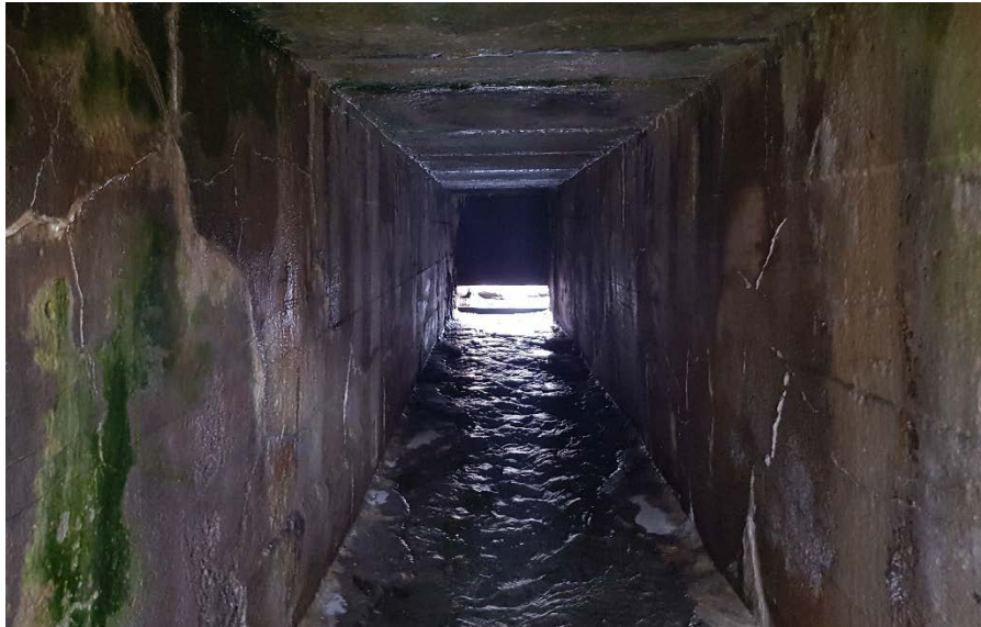
Turning Basin Basin Sluice
