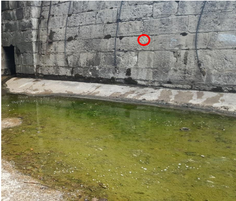
Core Location at East Chamber Wall
