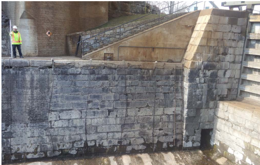
Lock 48 West Side – Chamber Wall
