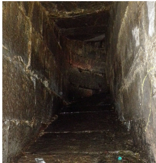
Lock 46 West Side – Sluice Tunnel
