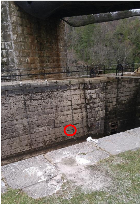
Core Location at West Chamber Wall
