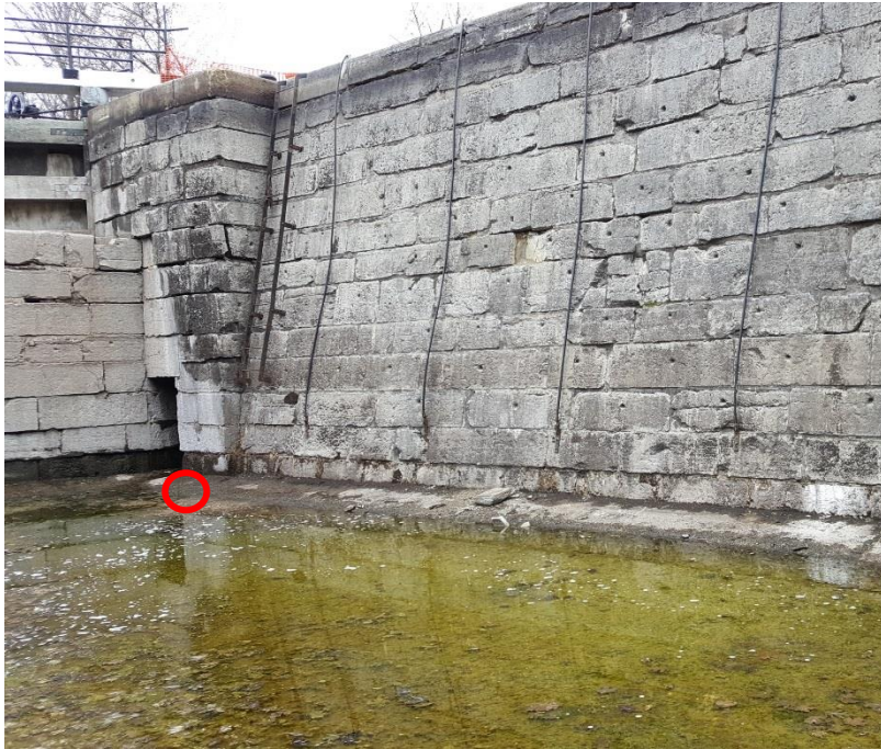
Core Location at Lock Floor
