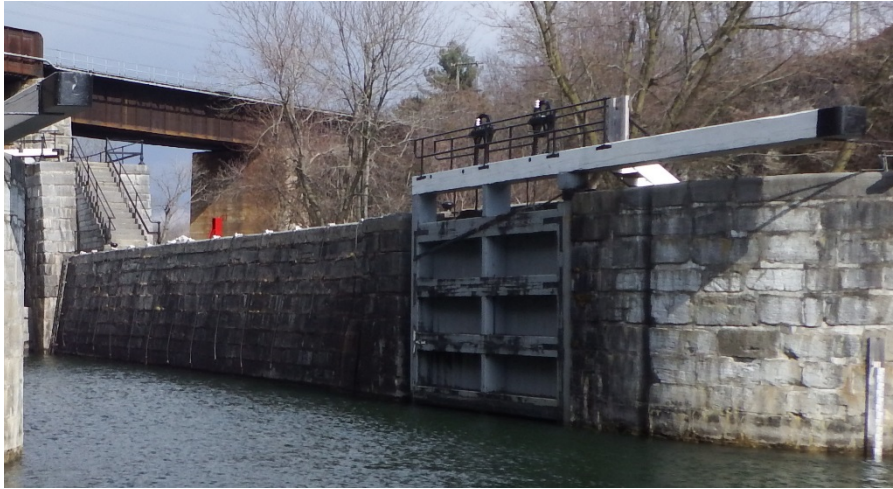
Lock 49 East Side – Chamber Wall
