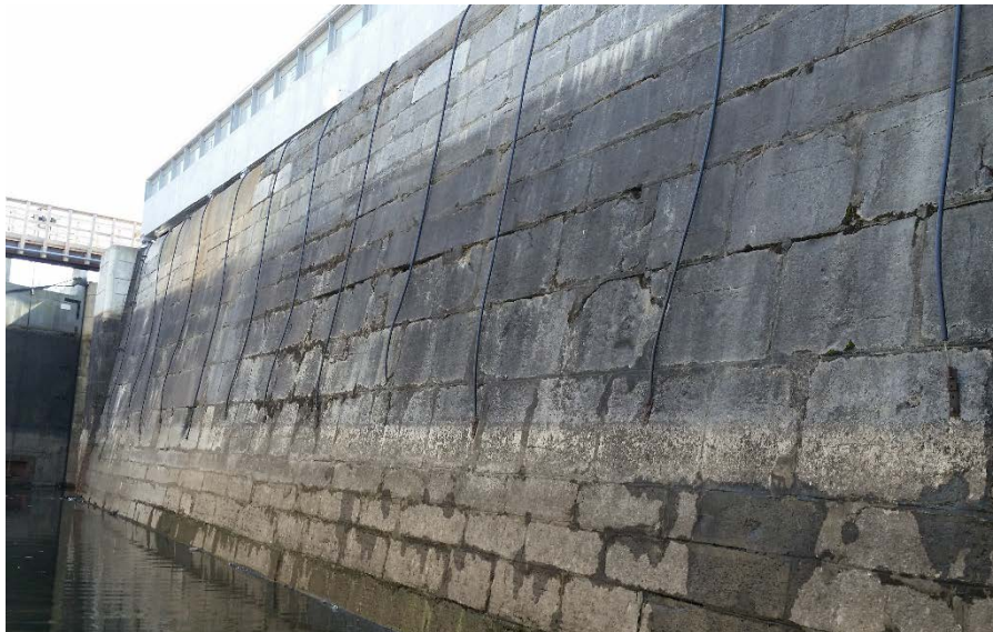
Lock 46 Chamber – West Wall
