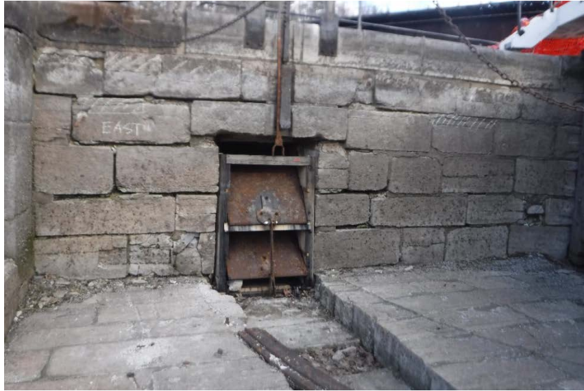
Lock 47 East Upstream Walls
