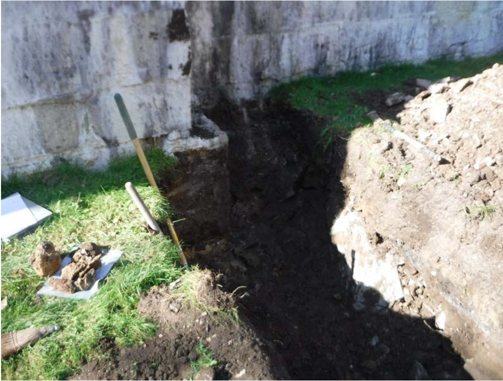
Test Pit #3 – Monolith #4 and back of lock chamber wall
