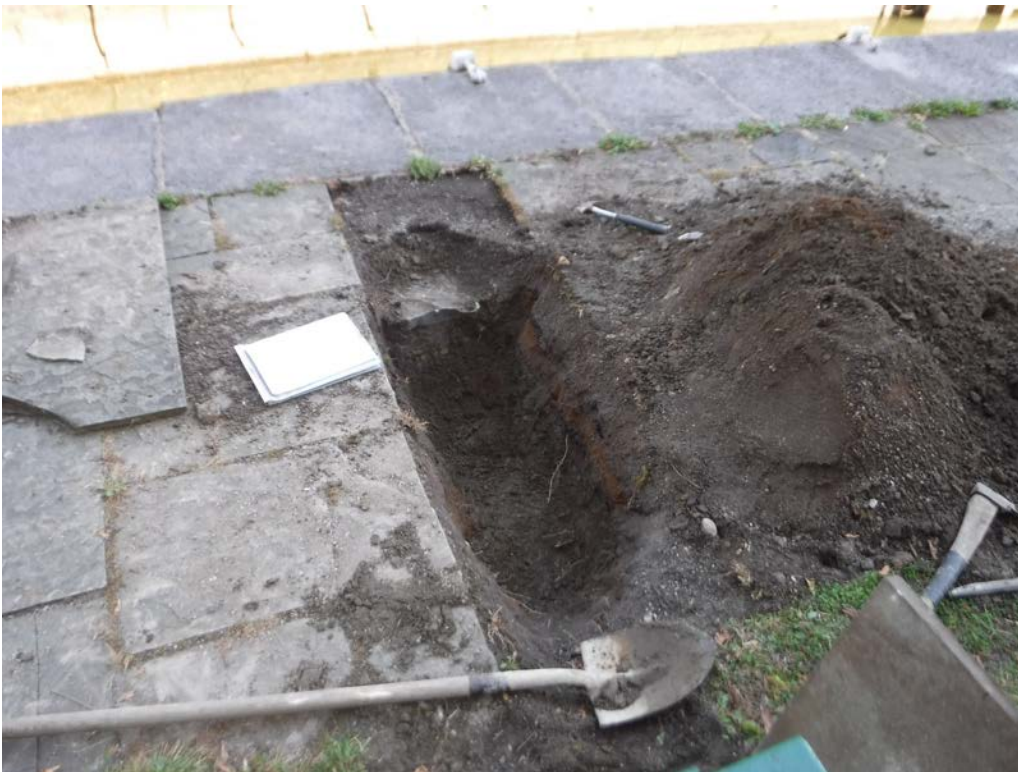
Test Pit #4 – Back of chamber wall
