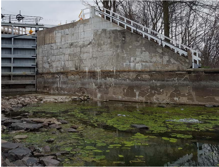
Lock 46 East Side of Lock – Southeast Wing wall
