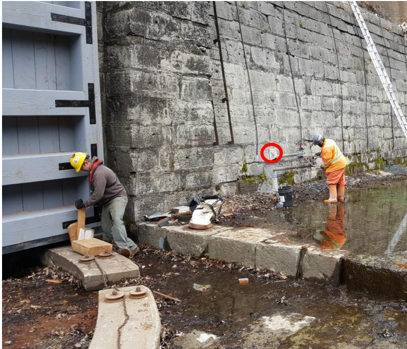
Core Location at West Chamber Wall
