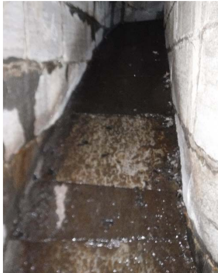
Lock 48 West Side – Sluice Tunnel
