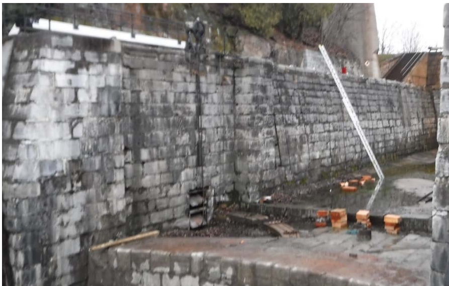
Lock 49 West Side – Chamber Wall
