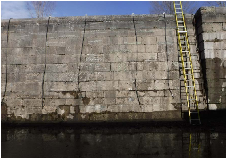
Lock 47 West Side – Chamber Wall
