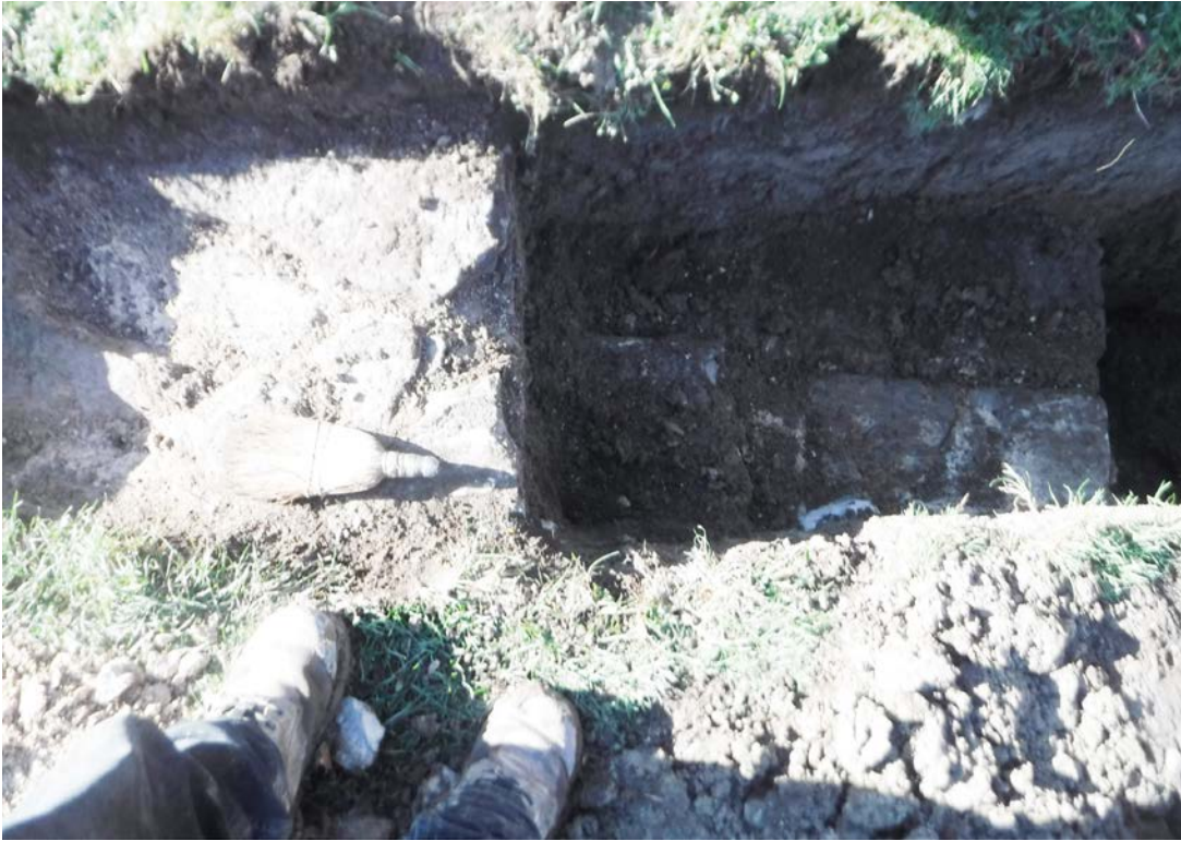
Test Pit #1 – Top of wall and buttress
