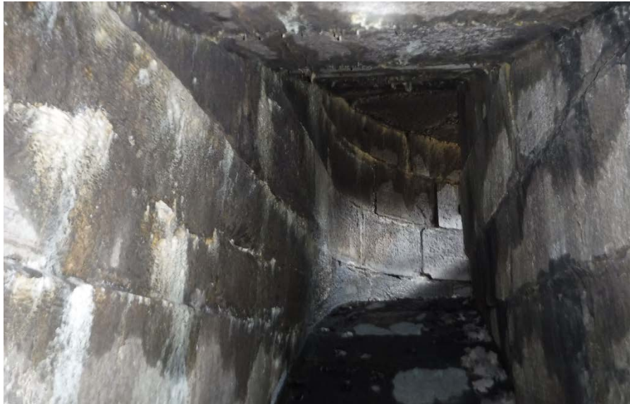
Lock 47 West Side – Sluice Tunnel
