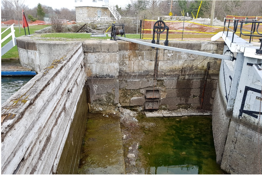
Lock 46 East Side of Lock Station – Lower Gate/Monolith
