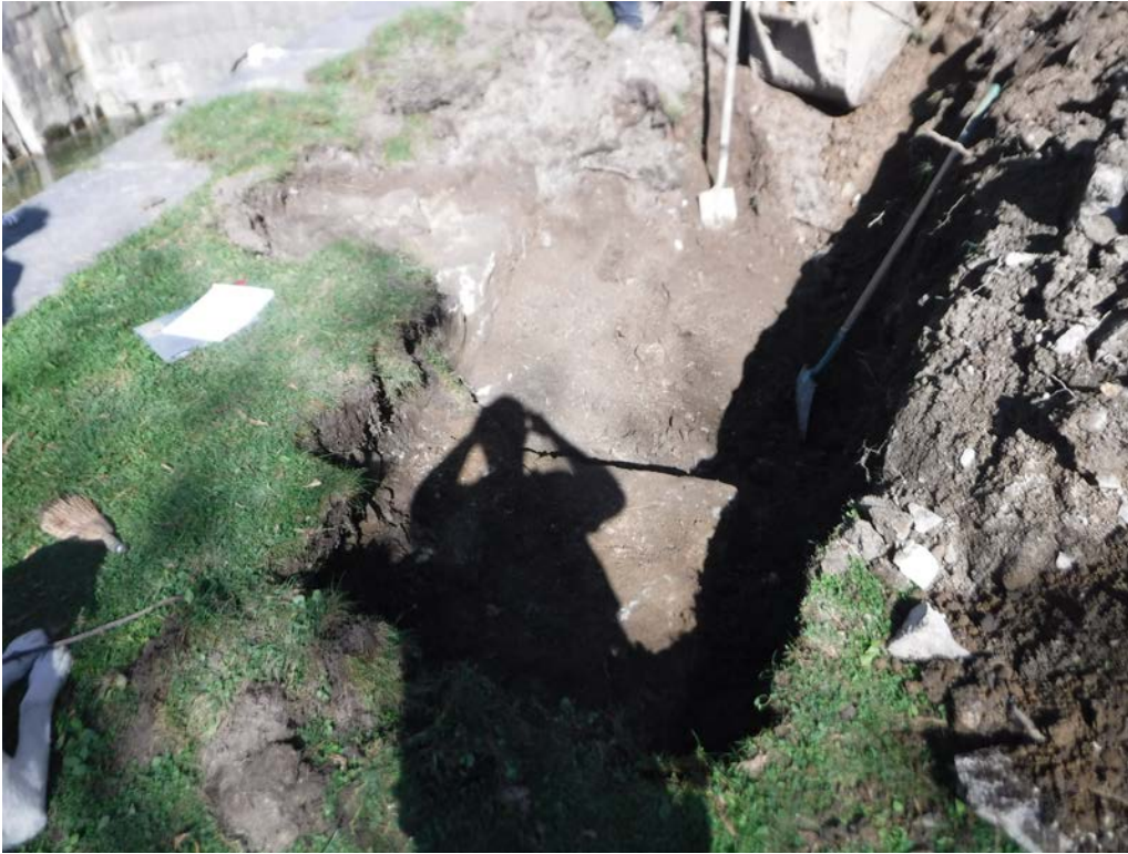
Test Pit #2 – Butters and back of chamber wall
