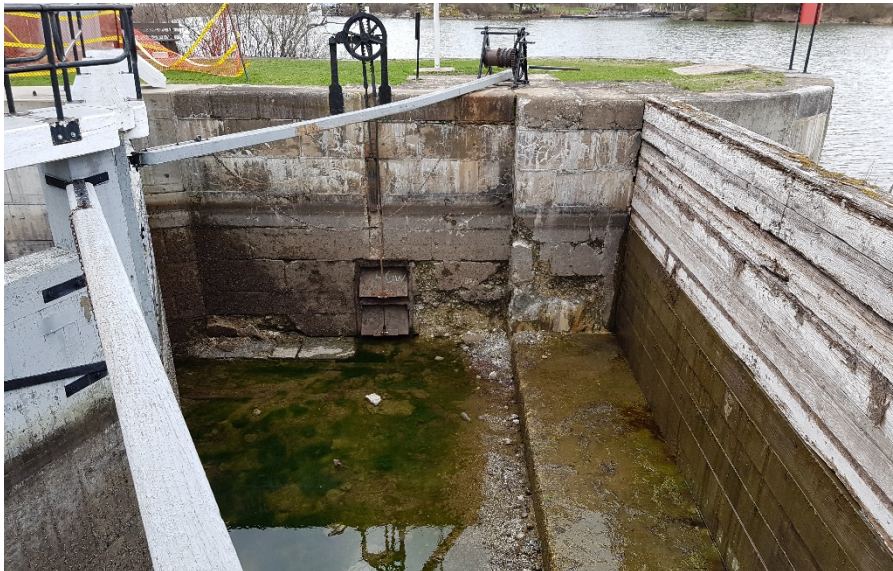
Lock 46 West Side of Lock Station – Lower Gate/Monolith/Buttress
