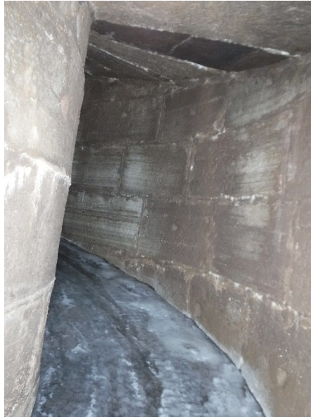
Lock 48 East Side – Sluice Tunnel
