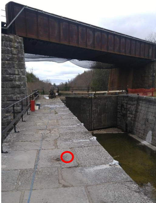
Core Location at East Chamber Wall
