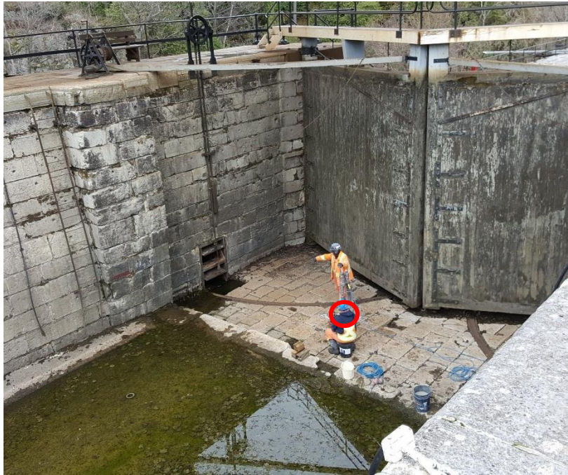
Core Location at Gate Recess Floor
