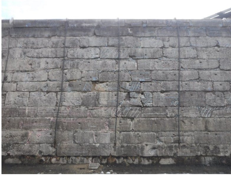
Lock 47 East Side – Chamber Wall
