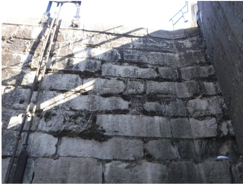
Lock 48 East Side – Buttress and Vertical Wall
