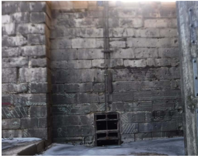
Lock 47 East Side – Buttress/Vertical Wall
