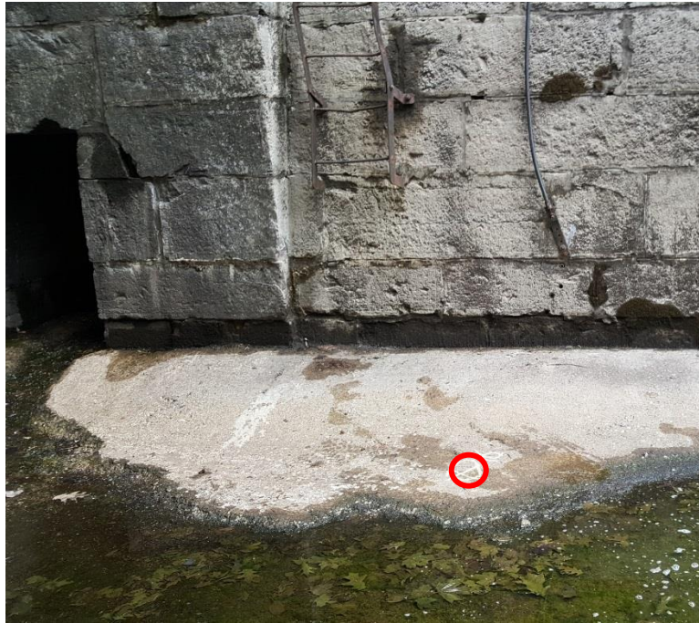
Core Location at Lock Floor
