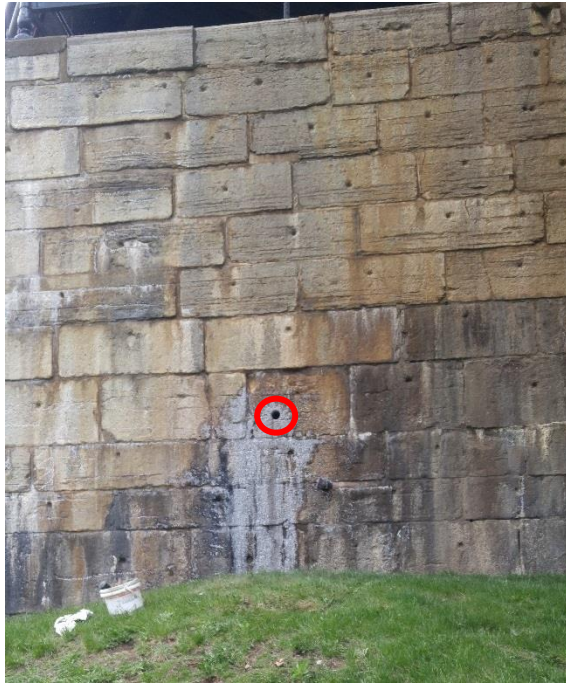
Core Location at East Pier
