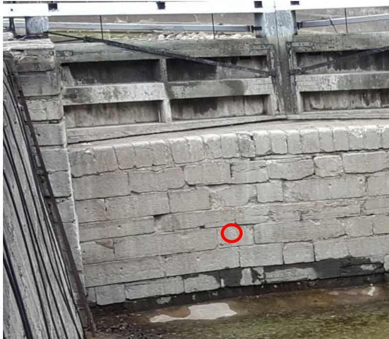
Core Location at Breast Wall
