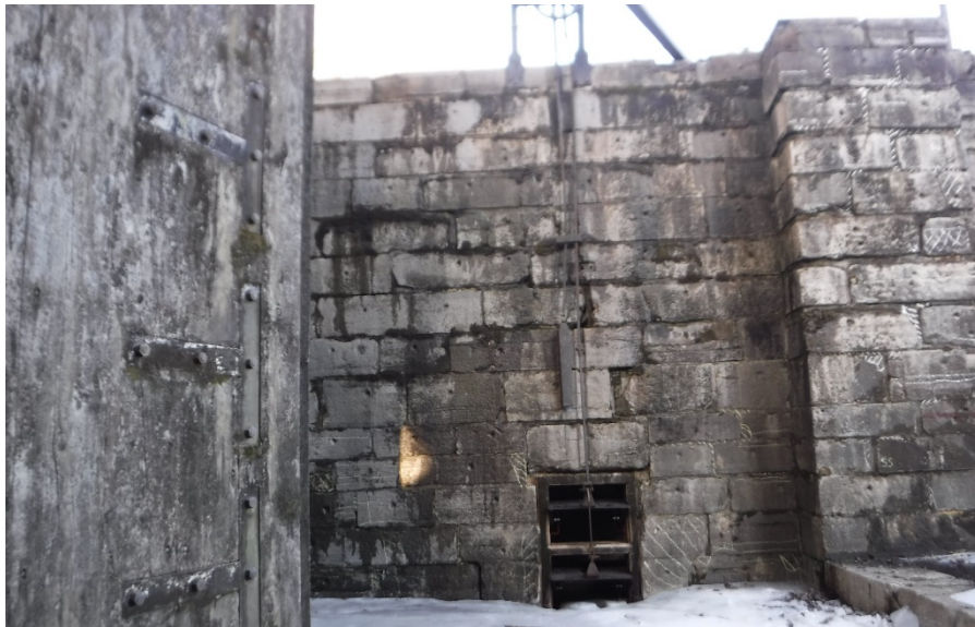
Lock 47 West Side – Buttress/Vertical Wall
