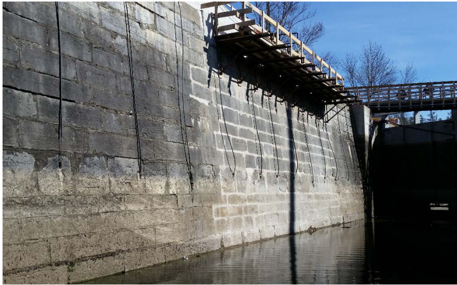
Lock 46 Chamber – East Wall
