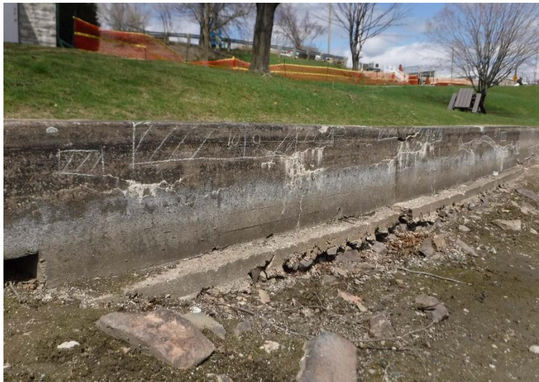
Turning Basin West Wall
