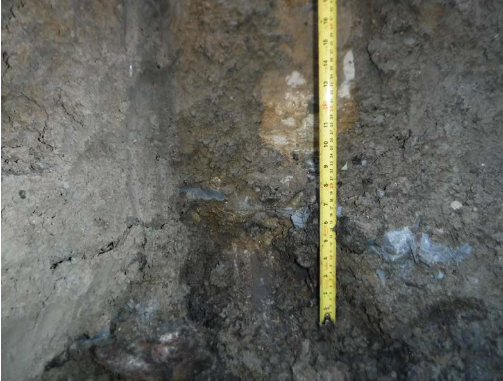
Test pit #1 – Layer of grout at bedrock
