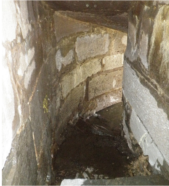
Lock 46 East Side – Sluice Tunnel
