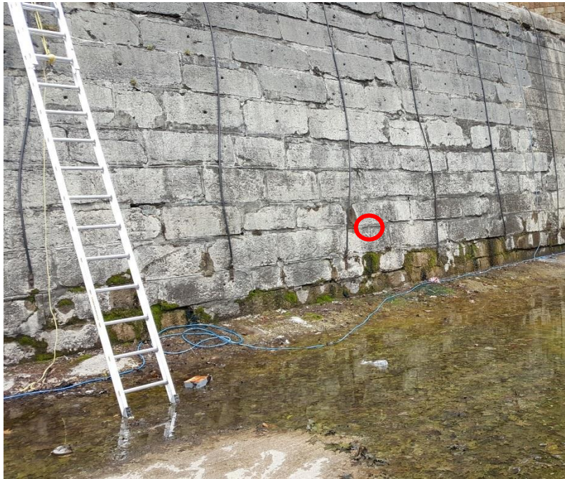
Core Location at West Chamber Wall
