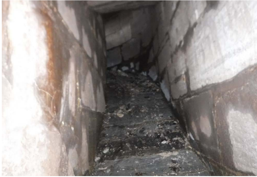
Lock 47 East Side – Sluice Tunnel
