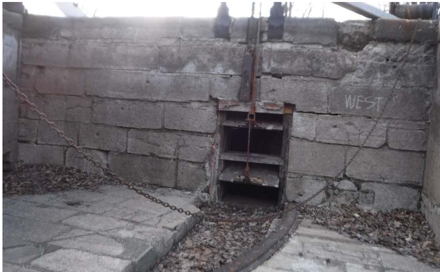
Lock 47 West Upstream Walls
