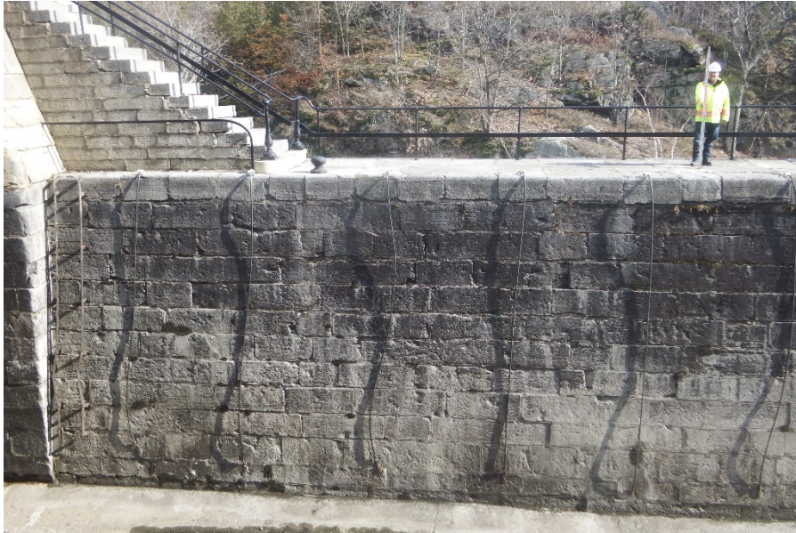
Lock 48 East Side – Chamber Wall
