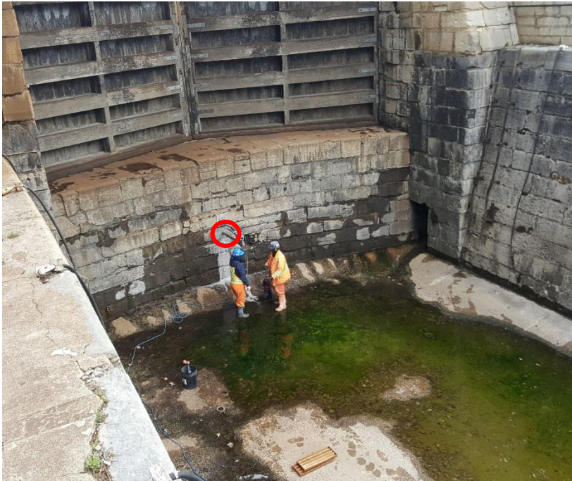
Core Location at Breast Wall
