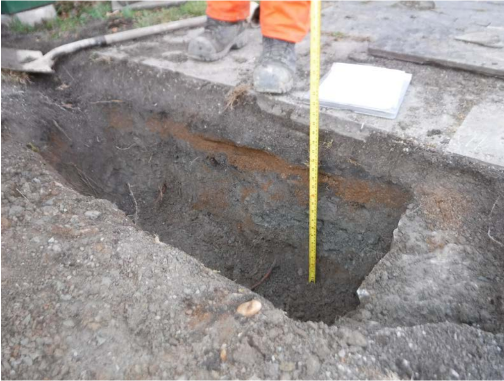
Test Pit #4 – Back of chamber wall
