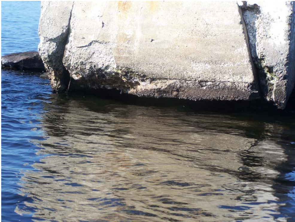
Figure 6: Existing weathered pier (to be removed)
