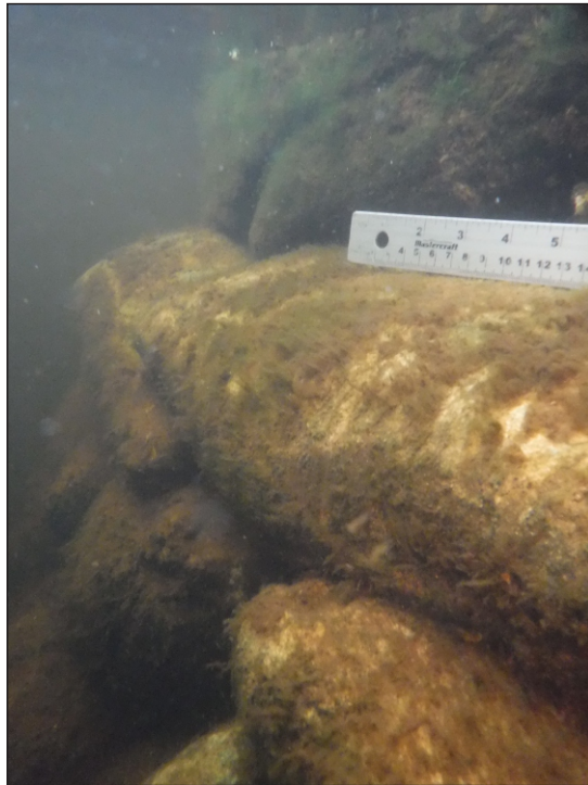
Image 1-59: Interface between grout bags and concrete cap at surface, west side of East Pier
