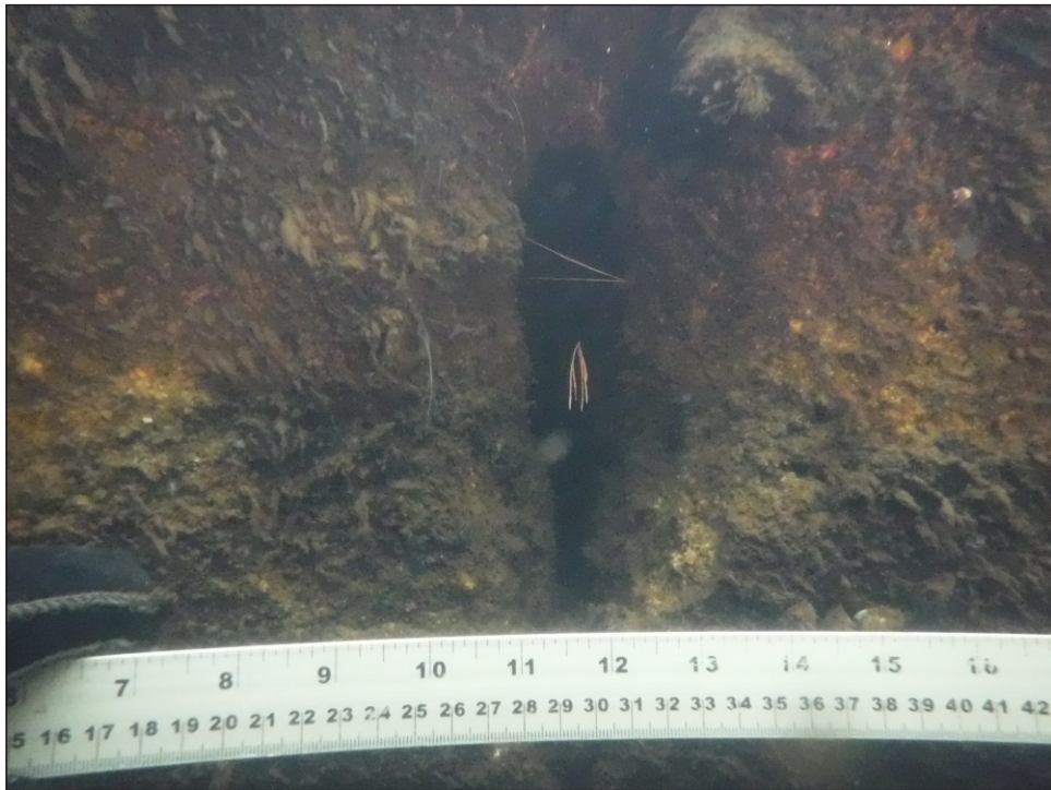
Image 1-46: Gap between concrete blocks west side of rest pier, gap/spall condition typical on west side of Rest Pier
