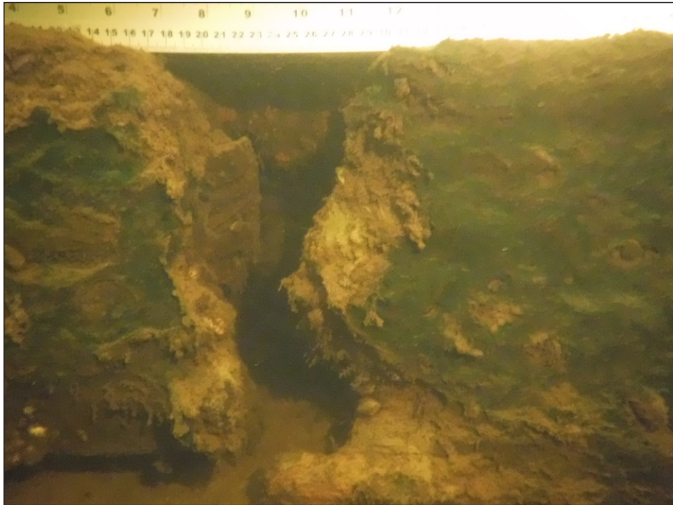
Image 1-31: Tieback timber, gap size typical on east side of Rest Pier
