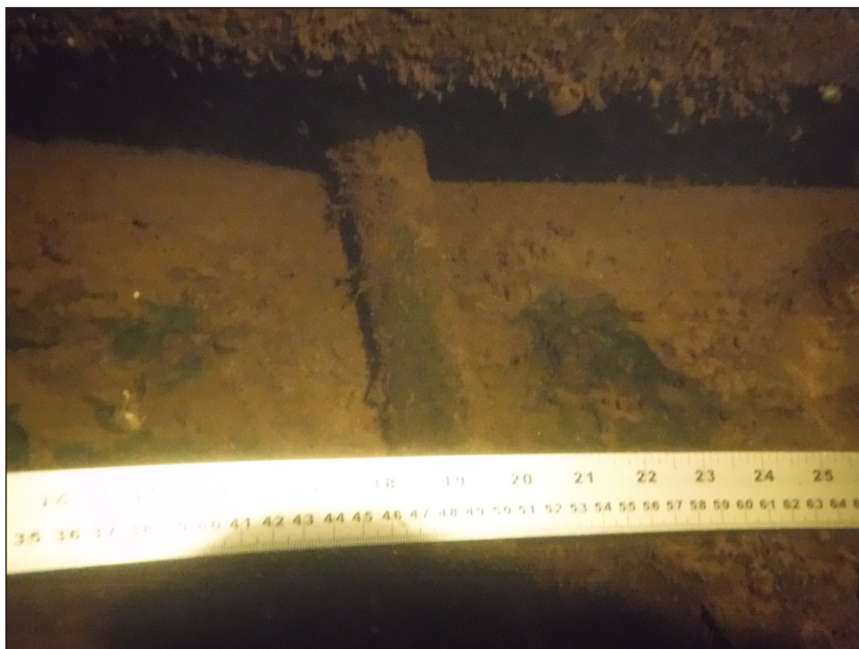
Image 1-24: Electrical conduit on east side of Rest Pier, extending into lake bottom
