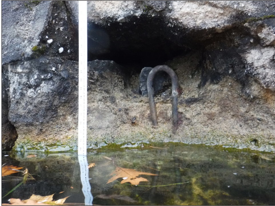
Image 1-45: Severe spall commencing above surface with exposed rebar, Rest Pier
