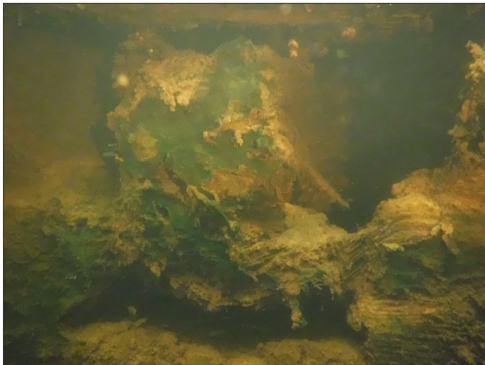
Image 1-40: Tieback timber, end grain rotted, Rest Pier
