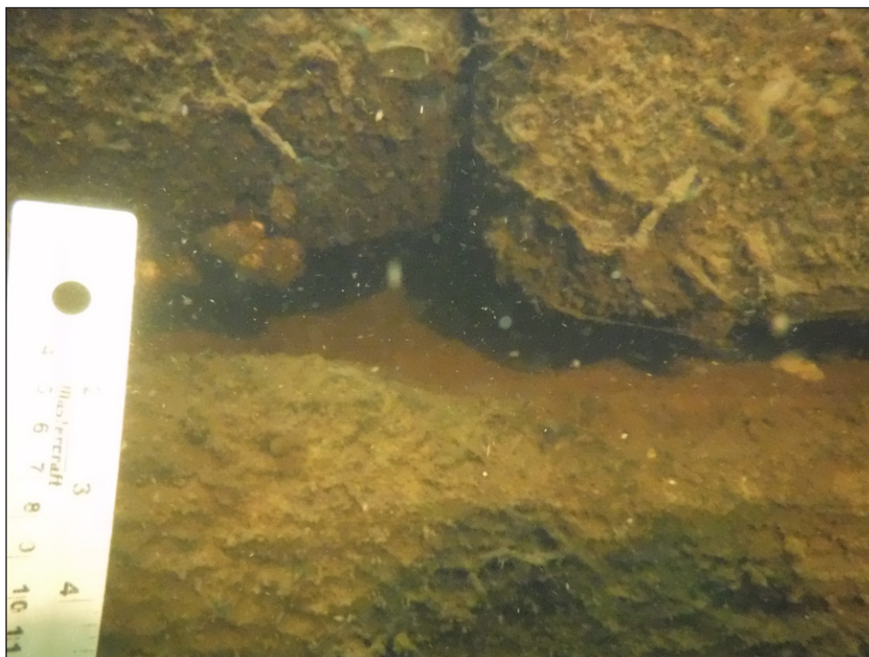
Image 1-37: Spall on concrete block, west side of Rest Pier. Gap/spall between blocks at corners typical throughout inspection
