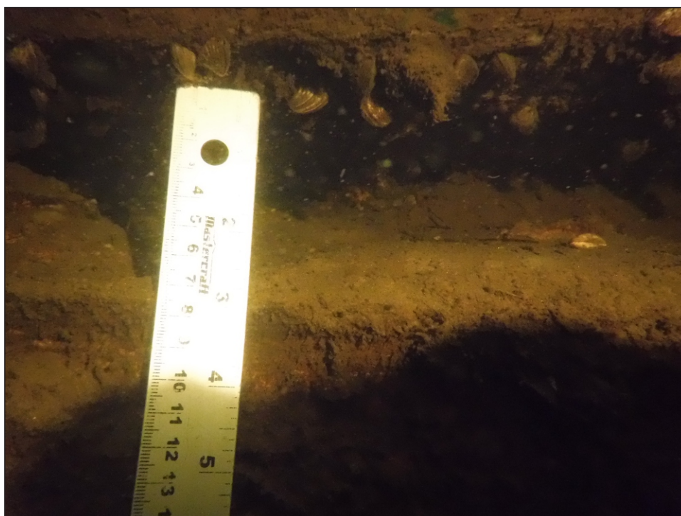
Image 1-28: Gap between timbers, east side of Rest Pier
