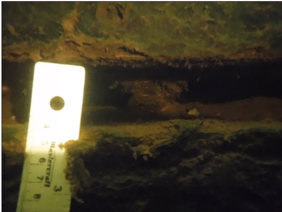
Image 1-32: Horizontal timbers, gap typical on east side of Rest Pier
