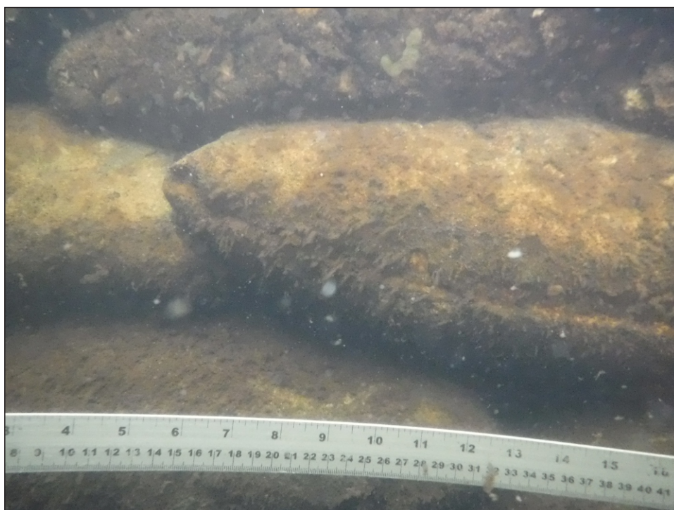
Image 1-54: Typical condition of grout bag, East Pier
