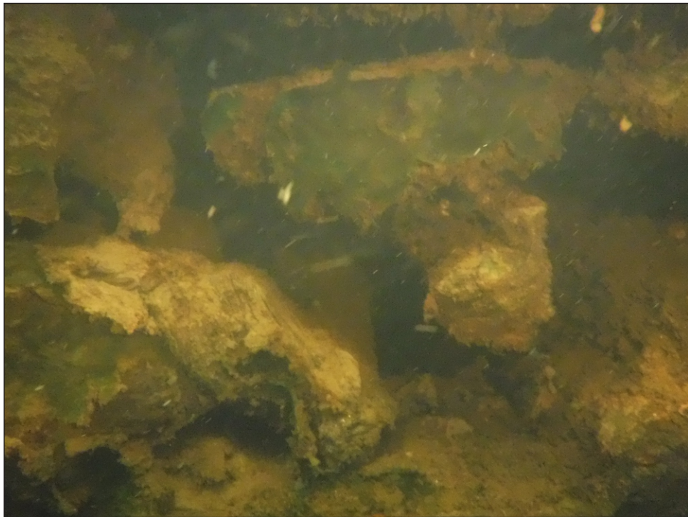
Image 1-42: Tieback timber, end grain rotted, west side of Rest Pier
