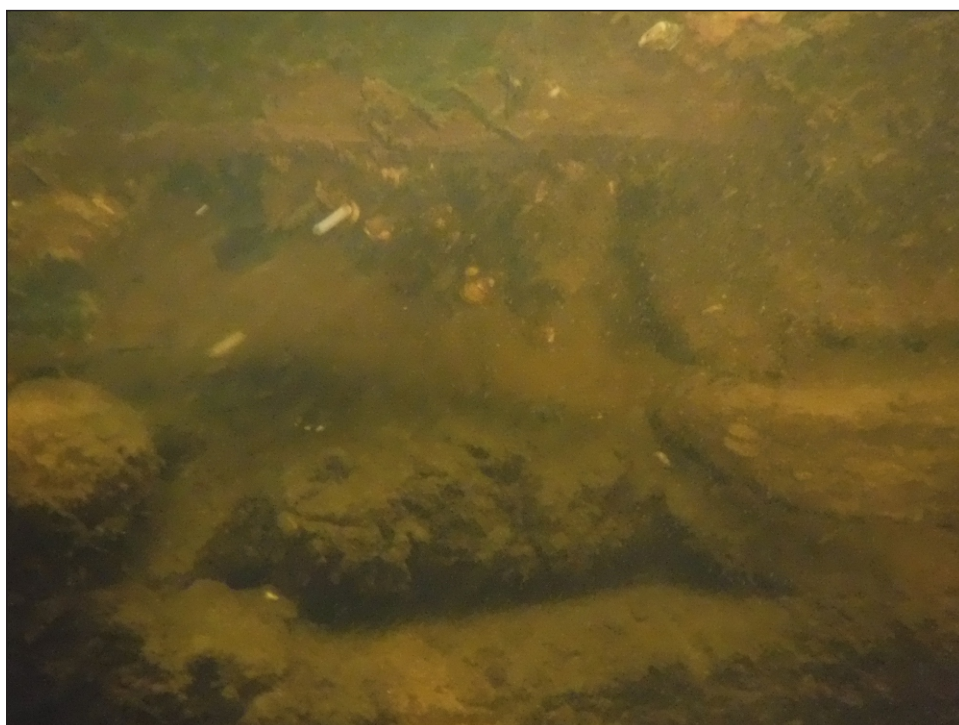
Image 1-30: Tieback timber in poor condition, east side of Rest Pier
