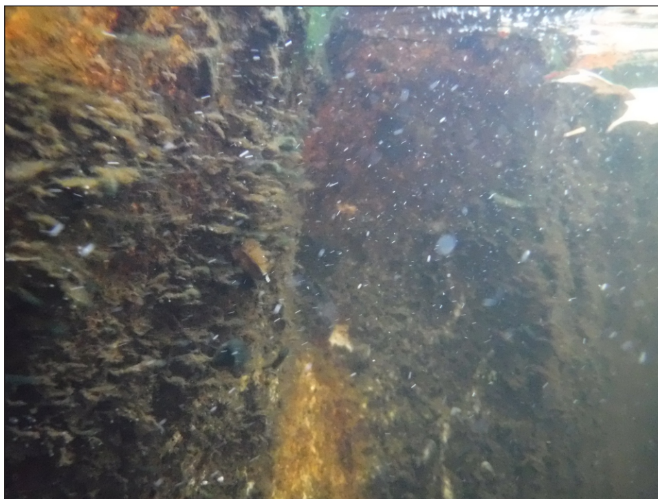
Image 1-48: Spall on concrete blocks, west side of Rest Pier
