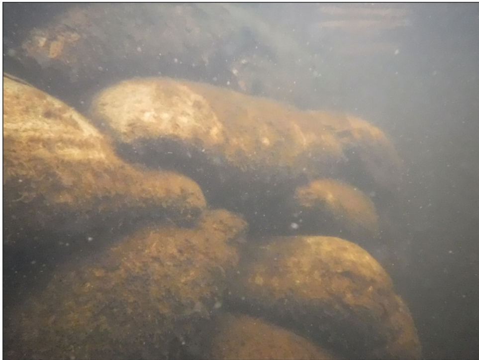
Image 1-56: Grout bags at base of East Pier
