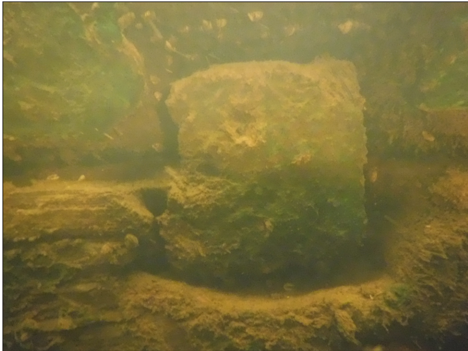
Image 1-43: Tieback timber end grain in good condition, Rest Pier
