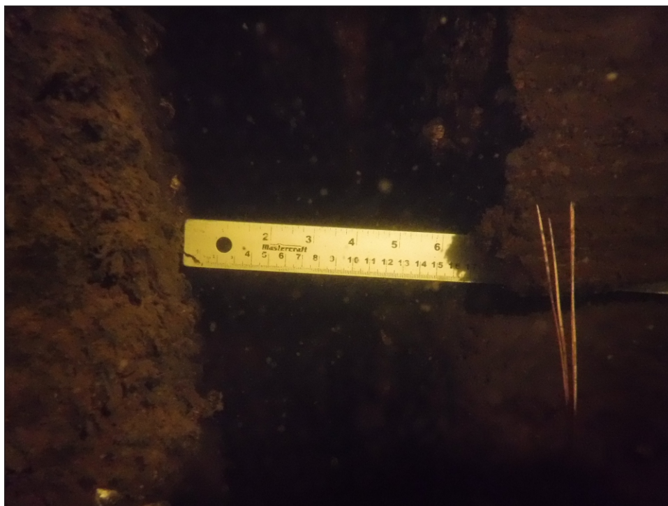
Image 1-27: Gap between timber crib and Pivot Pier, east side of Rest Pier
