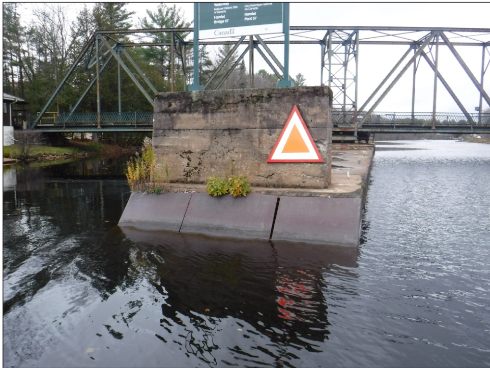
Image 1-6: South face of Rest Pier, looking north, steel plates extending into water
