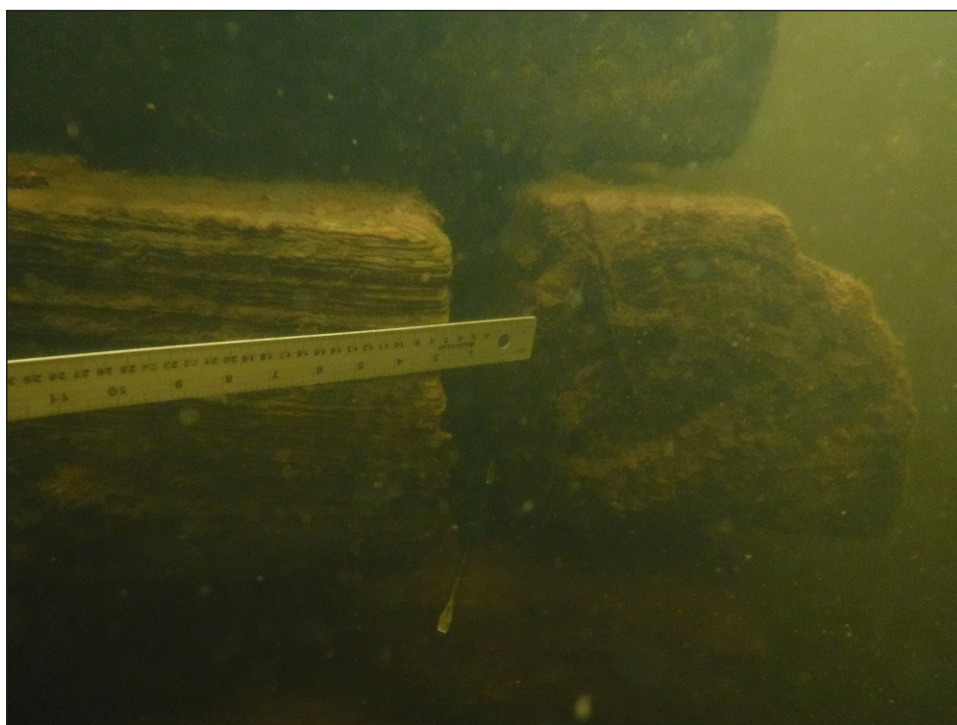
Image 1-20: North west corner of Rest Pier, looking south, gap between timbers
