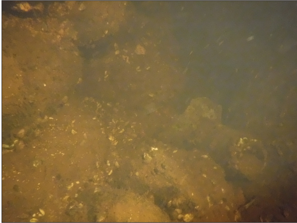
Image 1-63: Interface of grout bags and lakebed, East Pier
