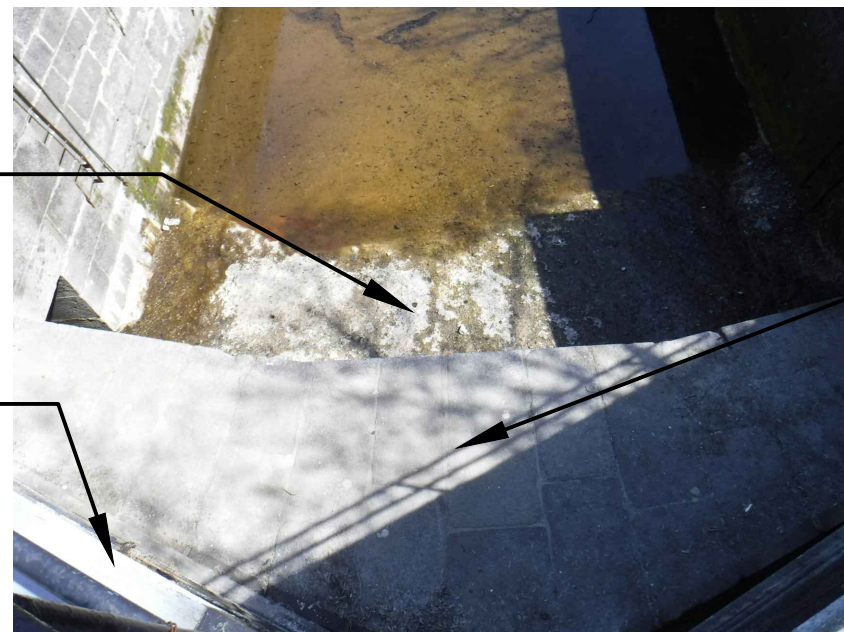
PHOTO 8 SCALE:NTS SKYWARD FACING JOINTS OF LOCK 27 BREAST WALL AT GATE 1
