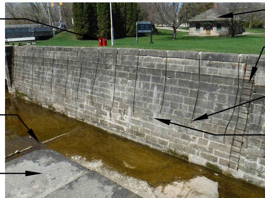
PHOTO 14 SCALE:NTS EAST LOCK WALL, REMOVE AND REINSTALL ANCHOR CABLES FOR BOATS, RECORD LOCATION PRIOR TO REMOVAL
