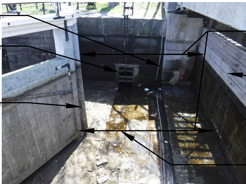
PHOTO 6 SCALE:NTS SLUICE TUNNEL GATE AND TRENCH, UPSTREAM LOCK 27 WEST WALL
