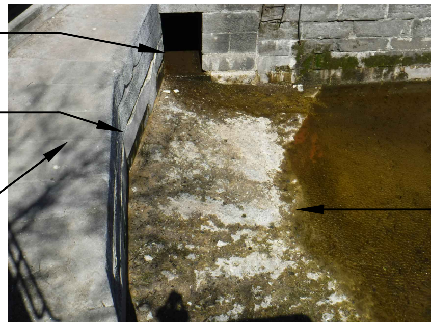
PHOTO 9 SCALE:NTS SLUICE TUNNEL ON SOUTH SIDE OF LOCK 27 BREAST WALL
