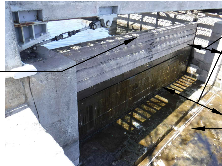
PHOTO 5 SCALE:NTS UPSTREAM STOP LOG GAINS UNDER BRIDGE
