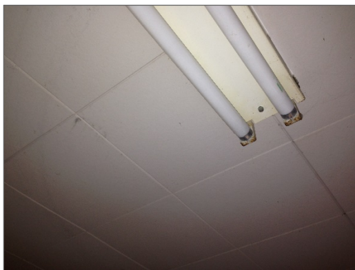
Photo 1 – Wood fibre ceiling tiles.
