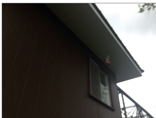
Photo 3 – Lead-based brown paint on exterior siding.
