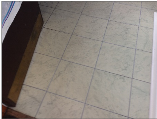
Photo 2 – Non-asbestos peel and stick vinyl floor tiles
