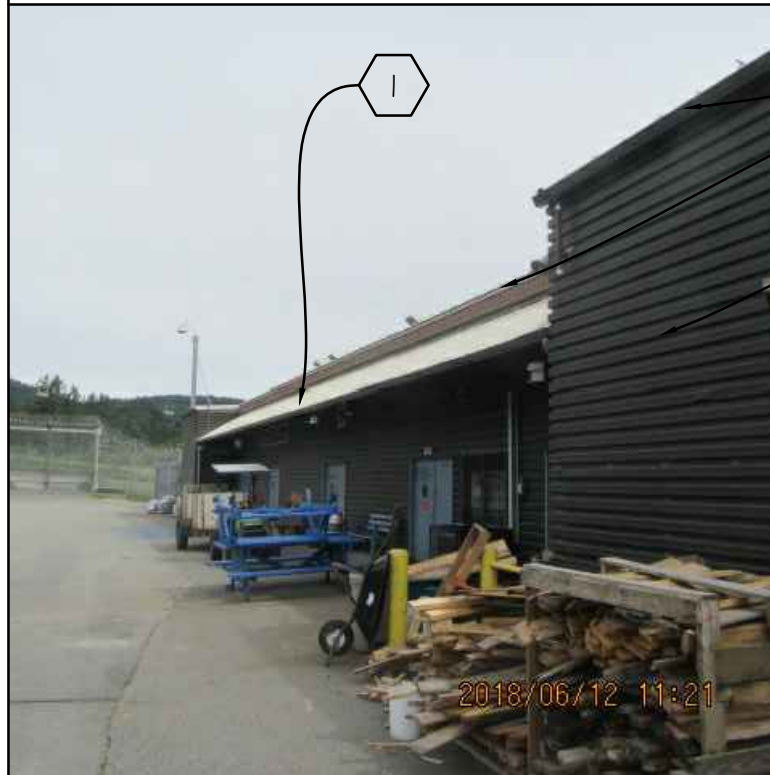
3 PHOTO OF EXISTING CONDITION
