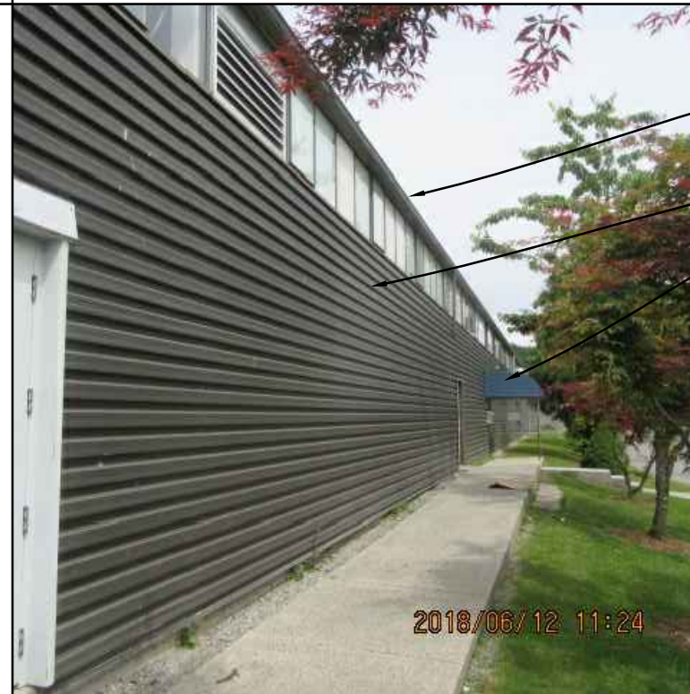
4 PHOTO OF EXISTING CONDITION
