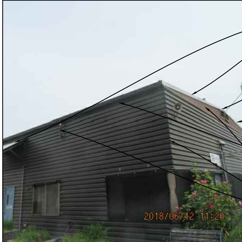
1 PHOTO OF EXISTING CONDITION
