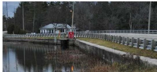
Scope: Replace the existing structures through the design and construction of new structures complete with all ancillary installations, operator safety features, fencing for public safety, shoreline stabilization and protection, landscape and embankment works, commissioning, demolition and/or removal of replaced installations and site restoration.
