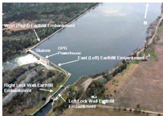
**Scope:** Improve operational effectiveness and modifications to prevent overflow, repairs to sills and piers, increase elevation of west and east approach walls.
