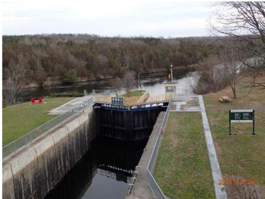
Scope: The scope will include the replacement of the six existing valves for Lock 11 and 12 with new valves and the associated works related to the installation. The scope will also include removal of existing gate hinges from the lower steel gates of Lock 11 and 12 and replacement with new as well as localized concrete repair and/or concrete design changes to anchor the new hinges into place. The lock gate gudgeon anchors (gate hinges) of the lower gates on Lock 11 and 12 will also be replaced
