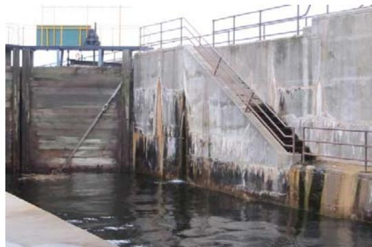
Scope: Repair the leakage through the common wall of the main dam pier #1 and the East lock wall as well as replace the lower staircase on the East side of the lock. Repair to the concrete cracks, spalls and delamination of upstream and downstream approach walls. Possible Construction of an extension of the lower entrance walls and/or construction of energy dissipating system or barriers,
