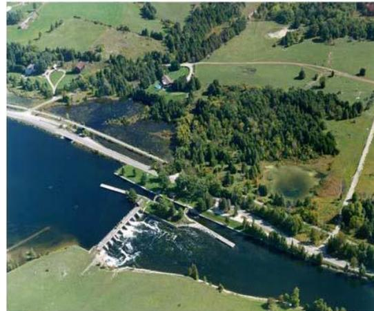
**Scope:** Replace the entire existing dam structure, including but not limited to the deck, piers, abutments, stop logs, spillways, upstream and downstream wing walls, and east and west approach slabs.
