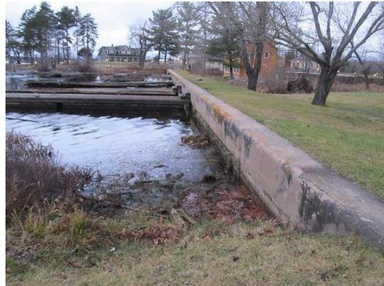
Scope: Repairs of joints and cracks using grout or other suitable methods for the concrete wall. Concrete patch repairs (minimum 200mm deep) in areas of degraded (spalled) surfaces is required. At the earth embankment, eroded soil material of the sinkholes is to be replaced by similar material and well compacted. Organic erosion control of the steepest section of the dam (approximately 15m length) is to be provided. This protection is to extend to the downstream slope.
