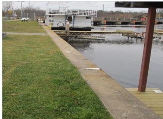
Scope: The scope of work includes concrete repairs for the majority of the length of the wall in areas of deep spalls which are located at low water levels (ice line).
