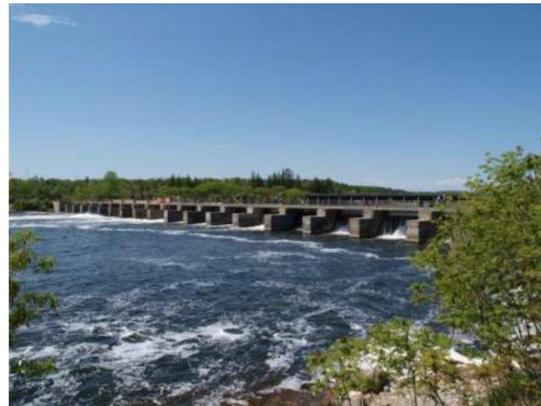
Scope: The demolition and replacement of the entire existing dam structure, including but not limited to the deck, piers, abutments, spillways, downstream apron, including the rehabilitation of the upstream west training wall.
