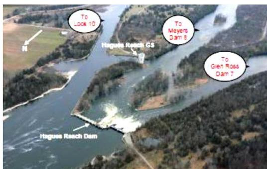
**Scope:** Improve operational effectiveness and modifications to prevent overflow, repairs to sills and piers, increase elevation of west and east approach walls, reconstruct the river wall as and where required and construction of an access bridge upstream of the radial gates.
