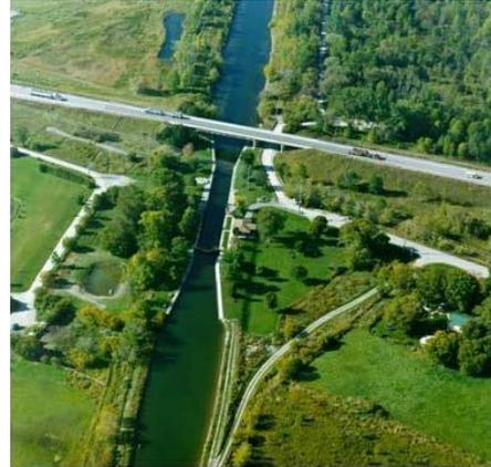
Scope: Ongoing site investigations will determine the extent of concrete repairs. Any work within the up and down stream gates can be achieved with closing the gates and pumping. Repairs outside the gates may require temporary measures for access.
