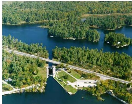
**Scope:** The entire existing dam structure at Lock 38 will be rehabilitated subject to specific conditions and design determinations, including but not limited to the deck, piers, abutments, spillways, south wing-wall and north wing-wall.
