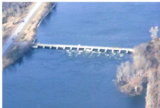
**Scope:** The demolition and replacement of the entire existing dam structure and restore and construct an erosion control mitigation and backfill embankment to restore the original profile.
