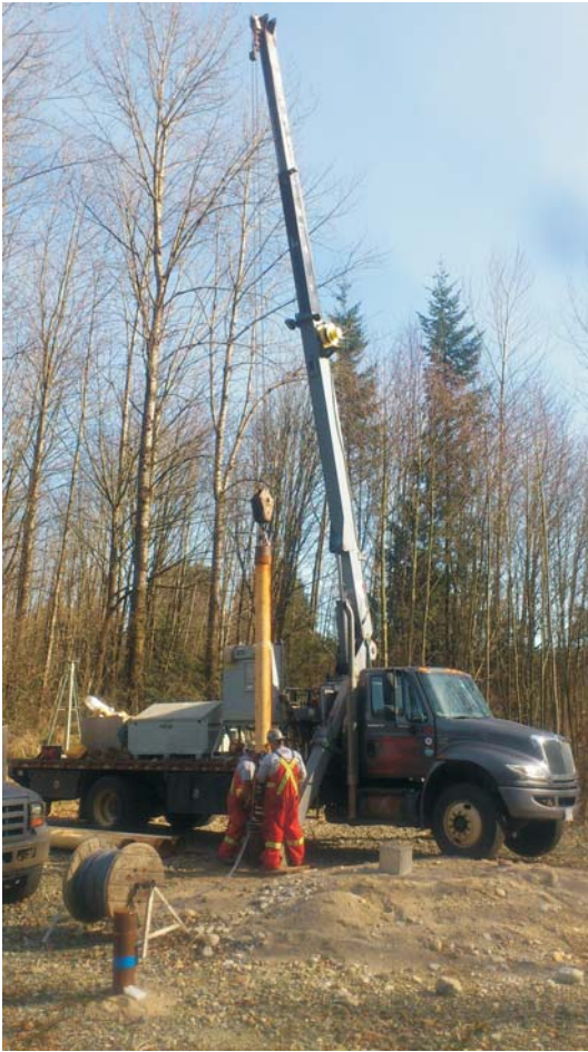
Photo 1. Installation of the test pump in Well #5.
