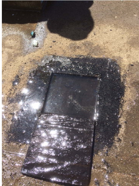
Water accumulation under monolithic membrane
