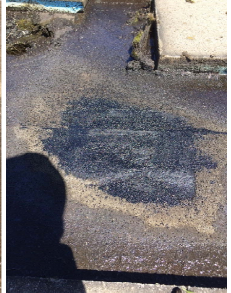
Water accumulation under monolithic membrane
