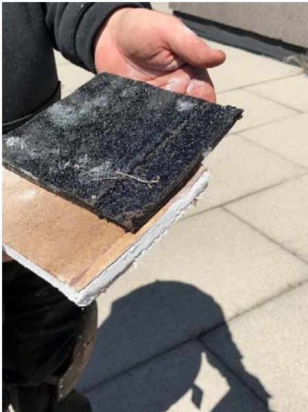
Gypsum decking and monolithic membrane
