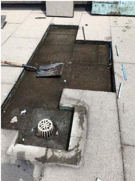
Removal of insulated panels
