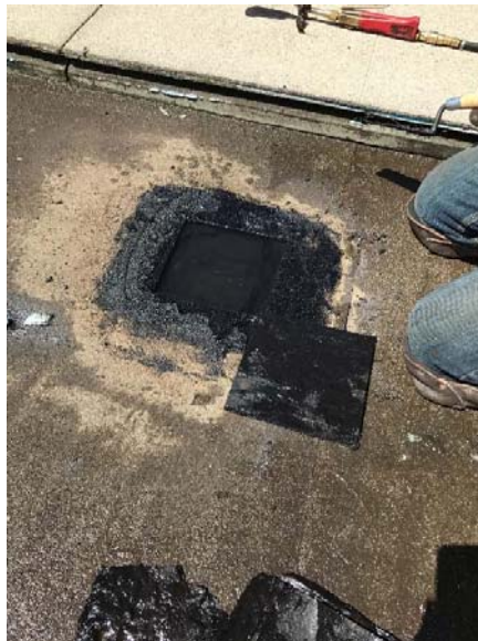
Water infiltration under monolithic membrane
