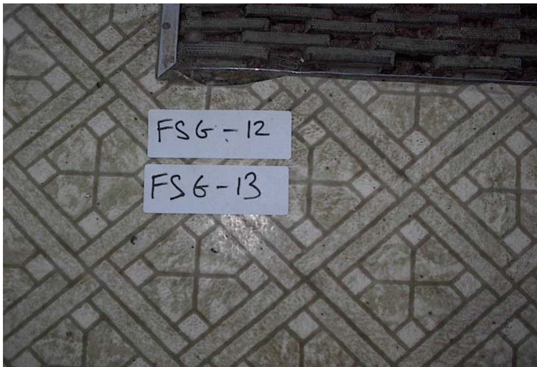
Photo 9: Sheet flooring and adhesive compound, Samples 12 and 13.
