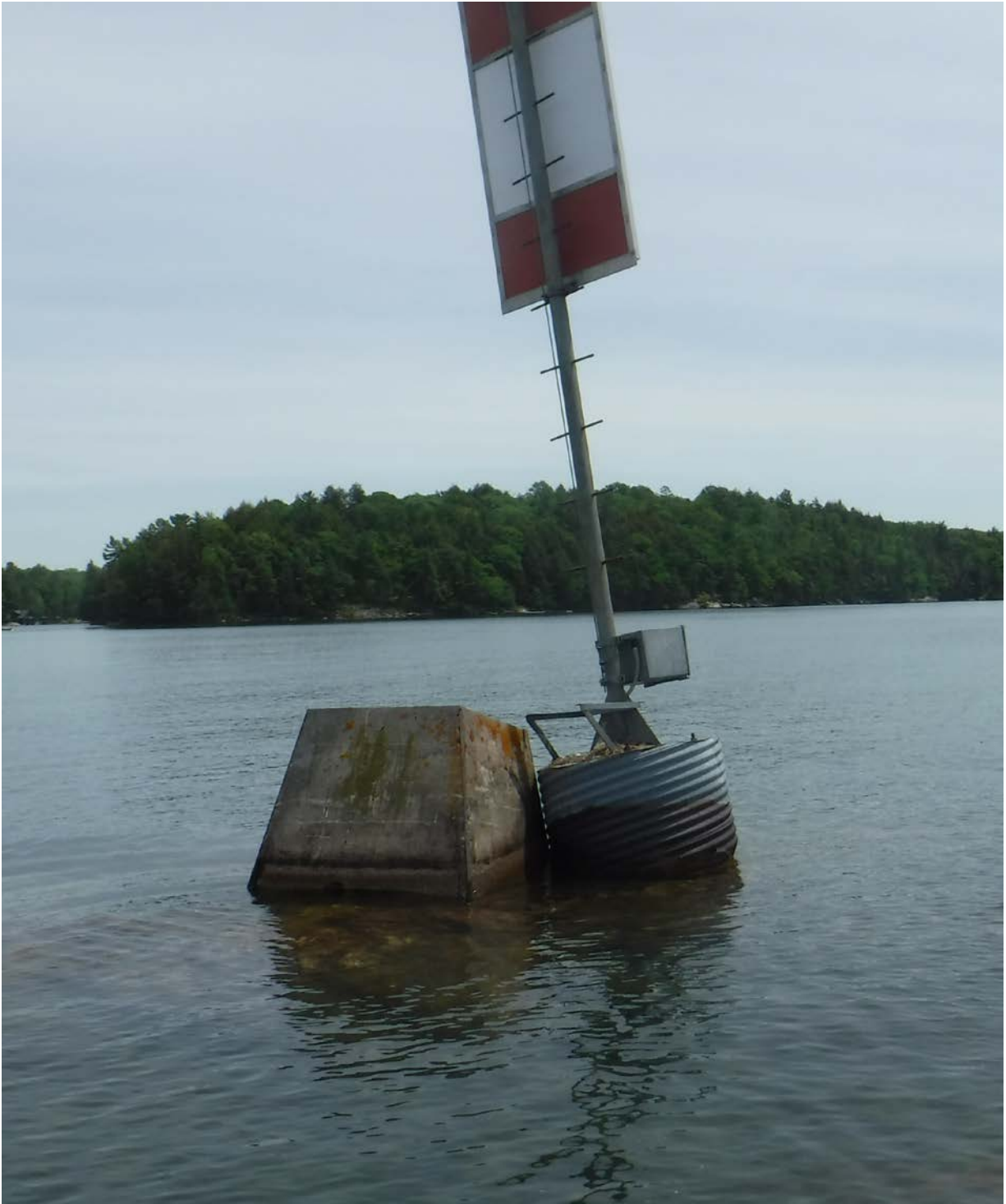
Figure 5: Existing Navaid with Current and Abandoned Foundations, Both to be Removed
