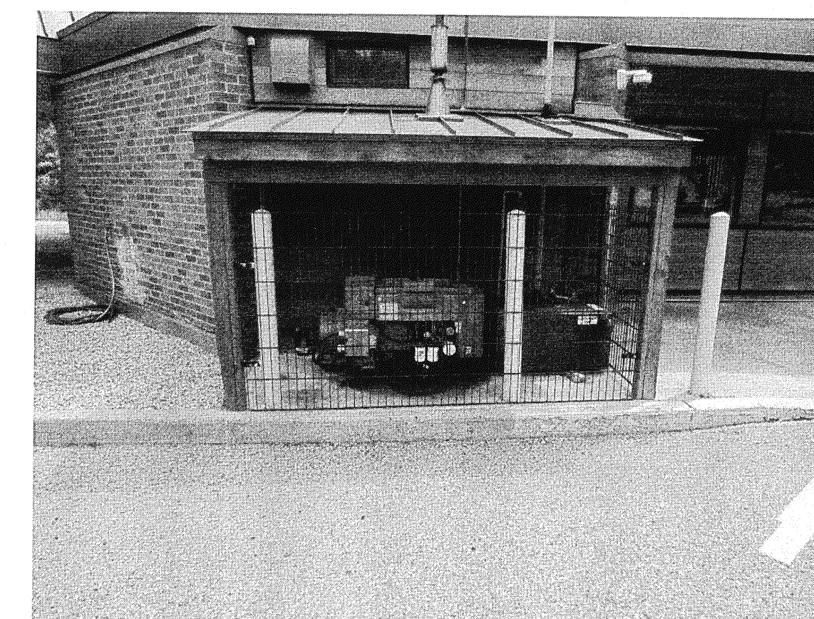
REMOVE EXISTING 12 KW GENERATOR AND THE WOOD STRUCTURE ATTACHED TO WANETA BORDER CROSSING BUILDING
