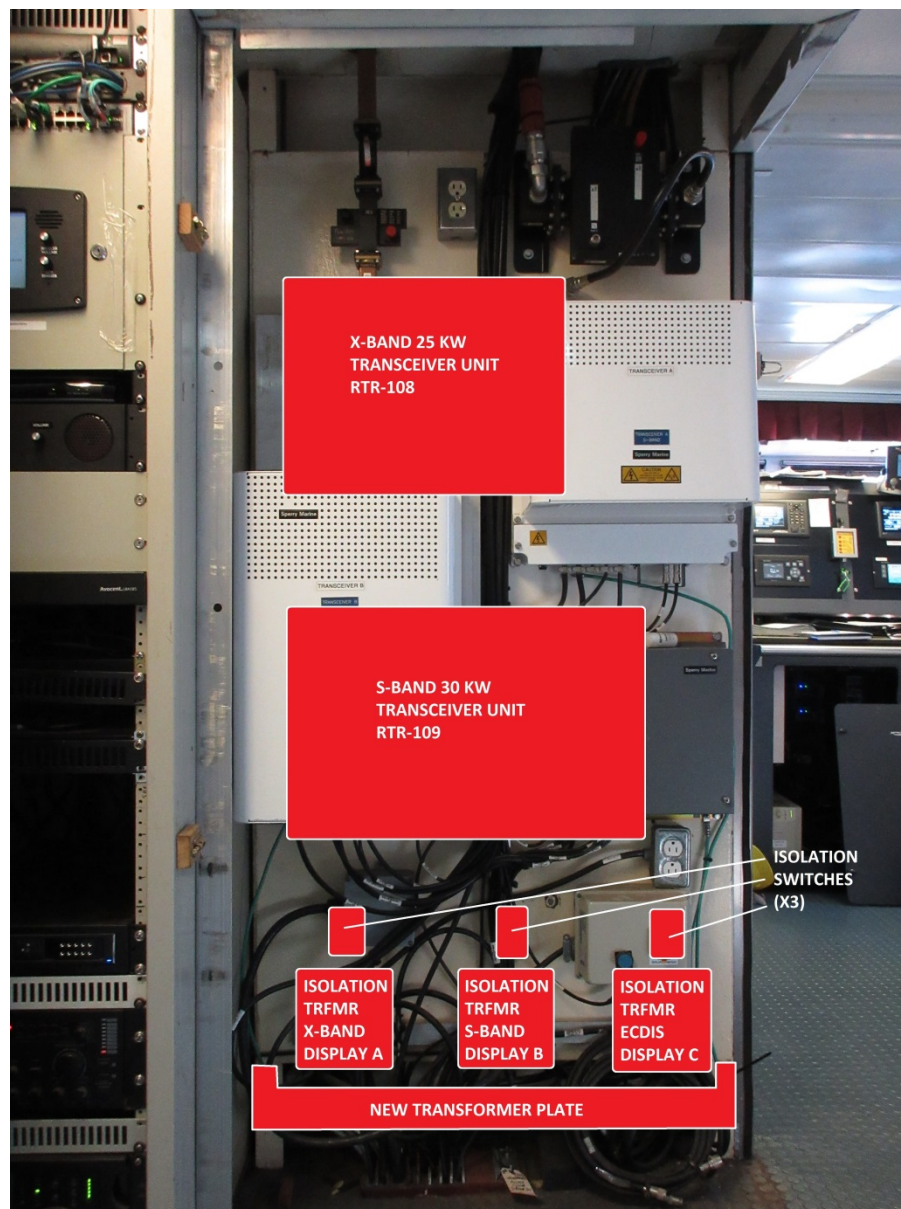
Picture: Location of Transceiver, Transformers, and Switches
