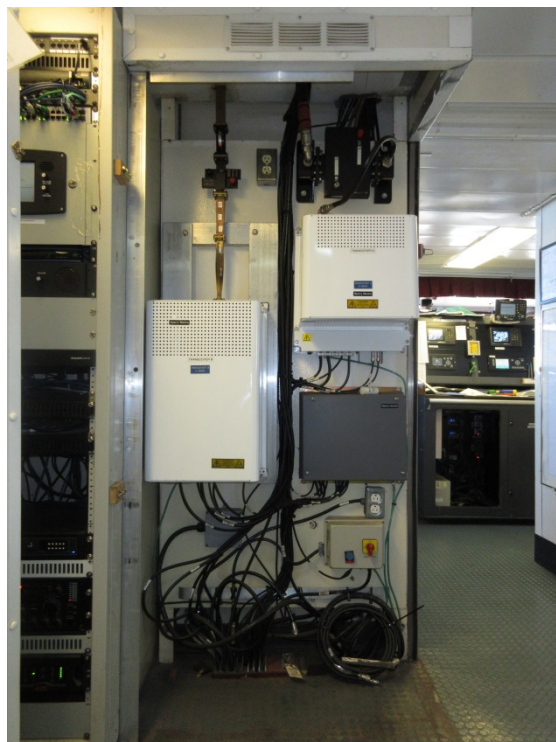
Picture: Radar Transceivers, Interswitch, and Scanner Control Unit
