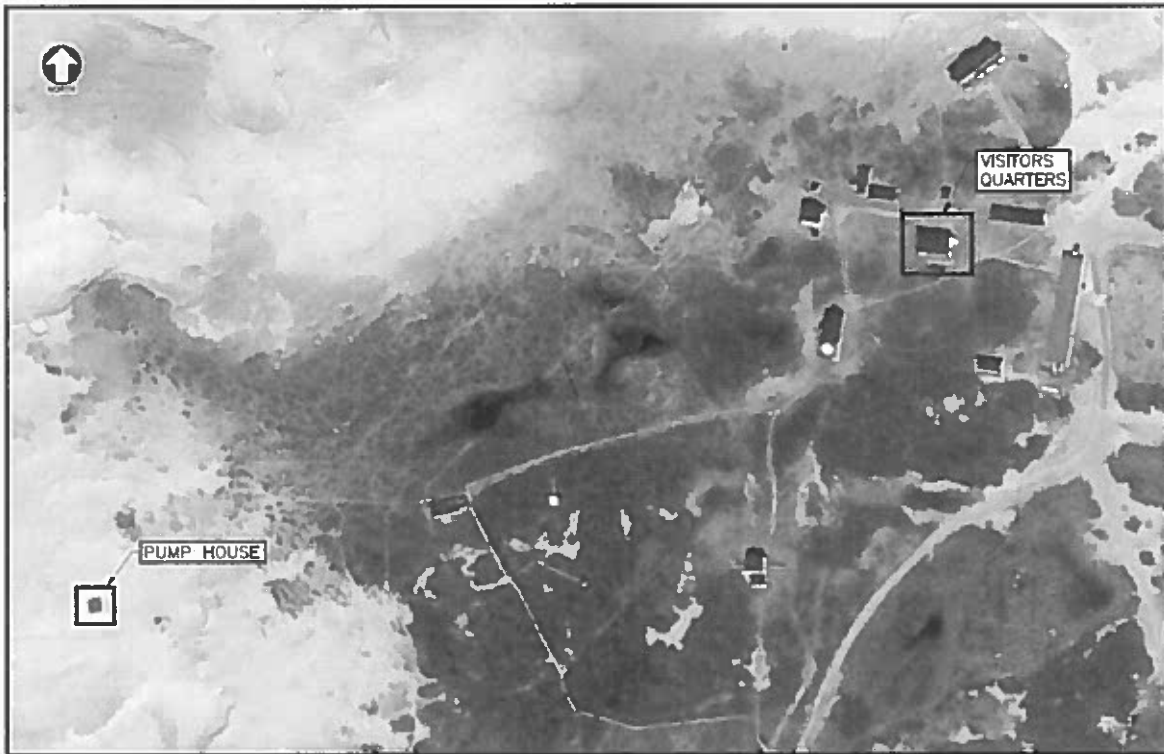
Figure 1: Location of the pump house relative to main station infrastructure.
