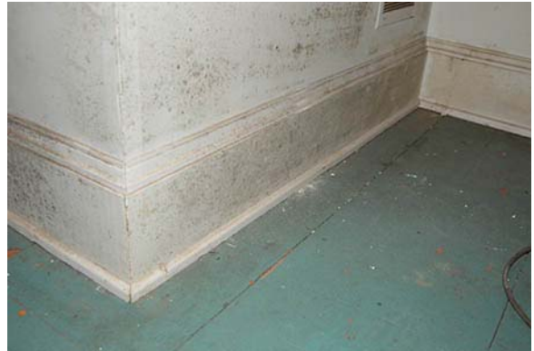
4. Baseboards & Trim Of Note: material, detailing
