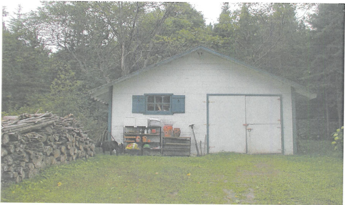
Photo 2: Former Barn, current garage (storage) looking south from laneway.
