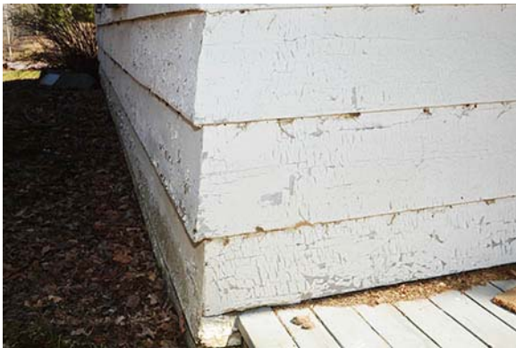
5. Exterior Wall Material Of Note: material, colour palette
