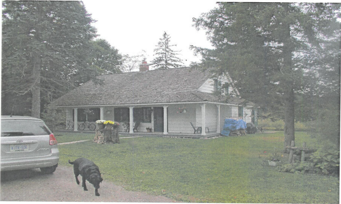
Photo 1: Home on subject site looking northwest.
