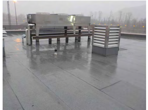
Photograph 6: General roof layout from roof hatch.
