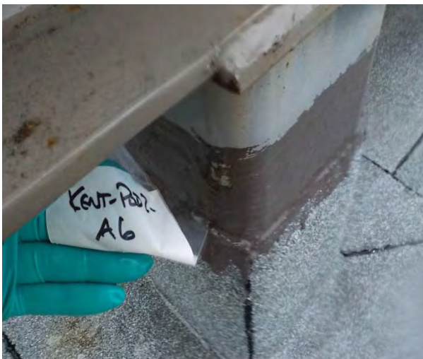
Photograph 7: Non-asbestos roof mastic (Samples A4, A5, and A6).
