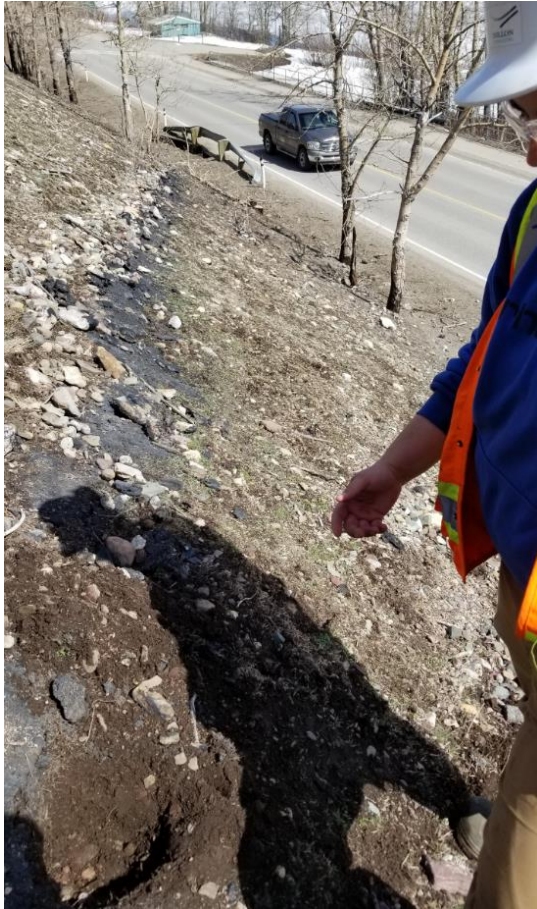
Photo 10b: Picture taken along the burnt salamander barriers. A trace of black burnt debris is visible where the barrier was previously.
