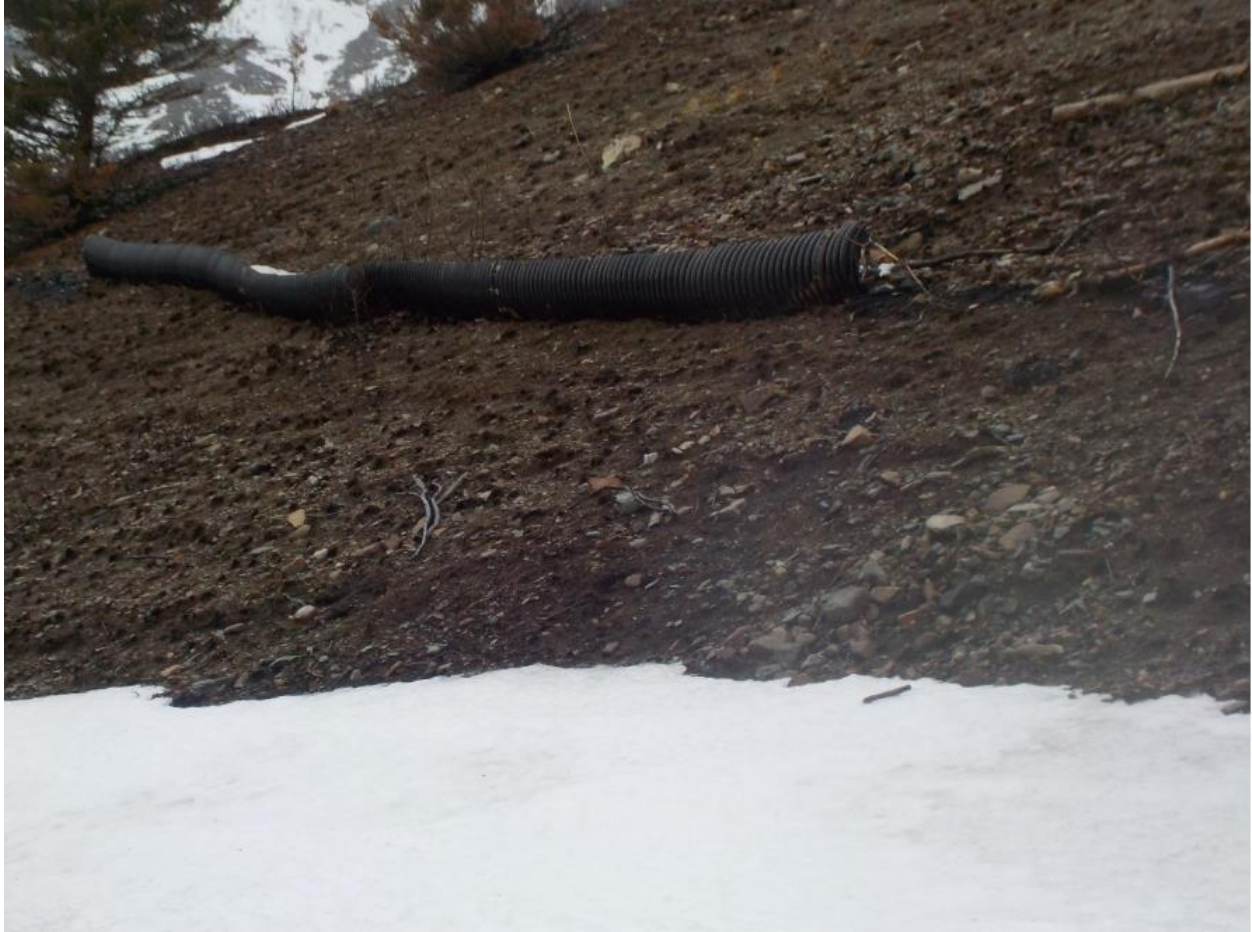
Photo 10a: Partially burnt Salamander Barrier. Image taken from COR#1 dated Jan 19, 2018.
