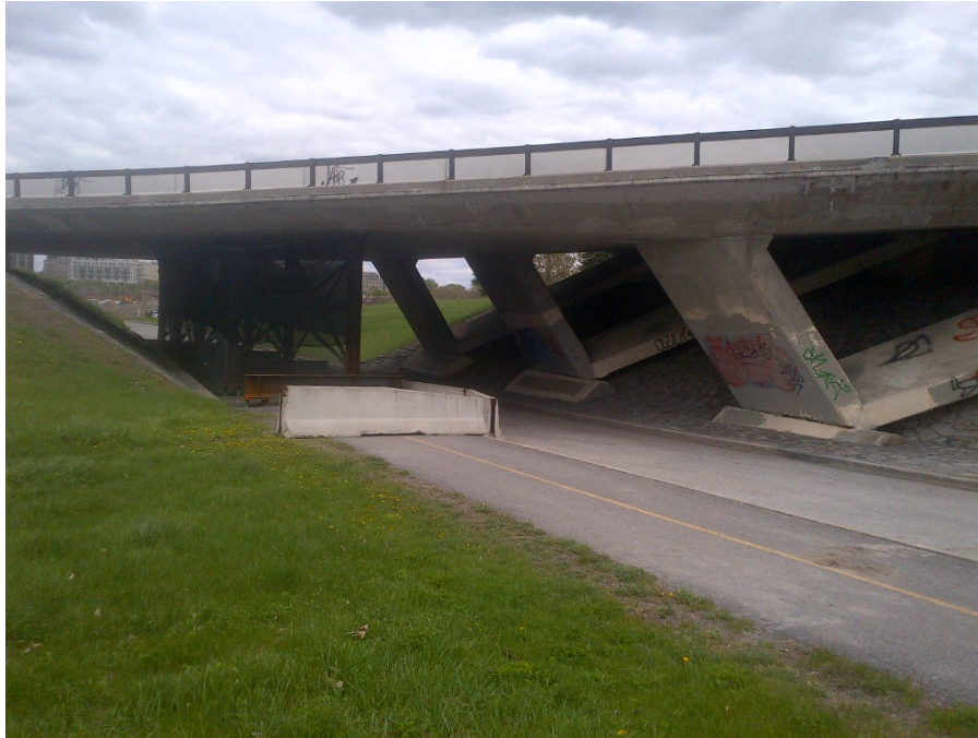
Figure 2 - LeBreton Flats exit (Ramp E) bridge, west elevation
