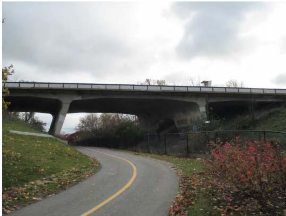
Figure 4 – CPR overhead bridge, north elevation
