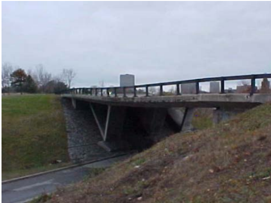
Figure 3 - LeBreton Flats exit (Ramp E) bridge, east elevation
