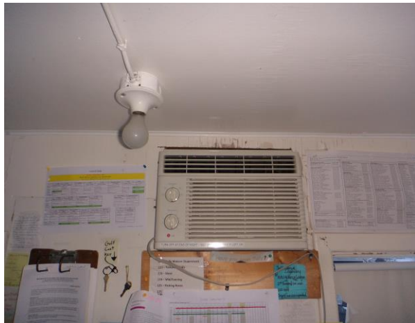
Photograph 21: Air Conditioner with Ozone-Depleting Substances in the Kiosk.
