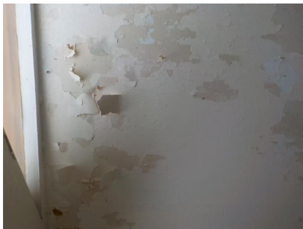
Photograph 02: Sample L-2, L-3, and L-4 – Lead Containing White (with Beige and Grey Underneath) Painted Interior Wood Walls and Ceiling in Pit Privy #1.
