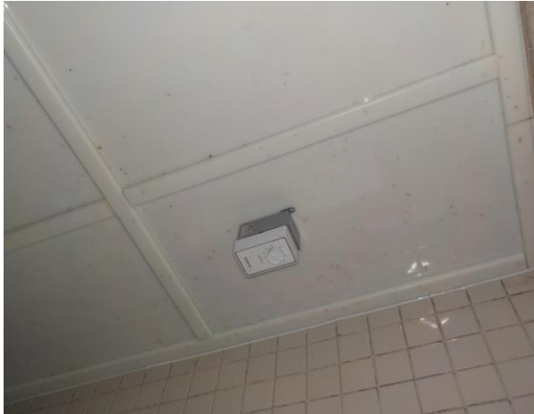
Photograph 19: Timer Potentially Containing Mercury Dust in the Shower Building
