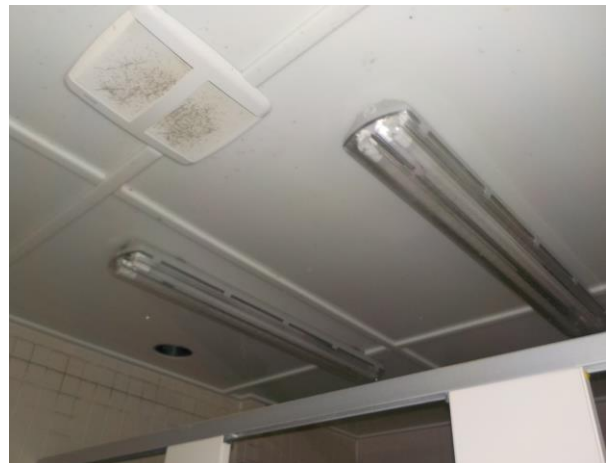
Photograph 16: Fluorescent Light Ballasts Potentially Containing PCB's and Fluorescent Light Tubes Potentially Containing Mercury Dust in the Shower Building.
