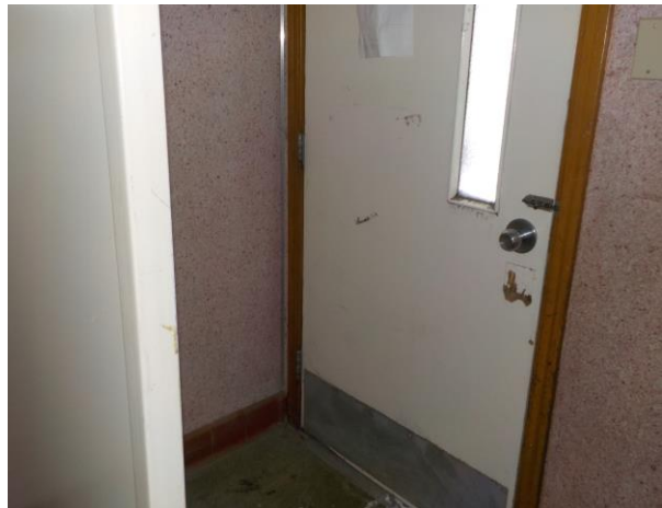
Photograph 02: Sample A-5 – Asbestos Containing Speckled Transite Wall Panel in the Men's and Women's Sections of the Shower Building.
