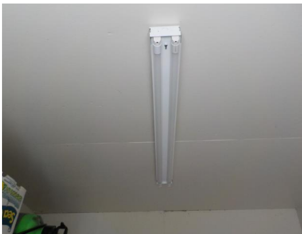
Photograph 17: Fluorescent Light Ballasts Potentially Containing PCB's and Fluorescent Light Tubes Potentially Containing Mercury Dust in the Storage Building.
