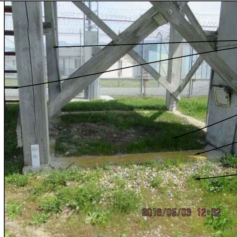
2 PHOTO OF EXISTING CONDITION
