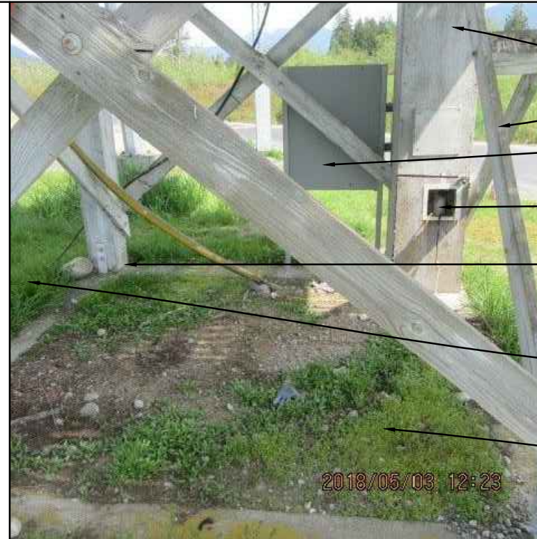
10 PHOTO OF EXISTING CONDITION
