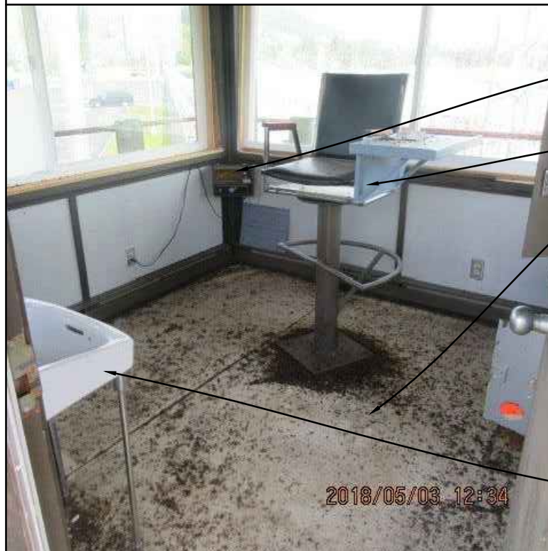
3 PHOTO OF EXISTING CONDITION
