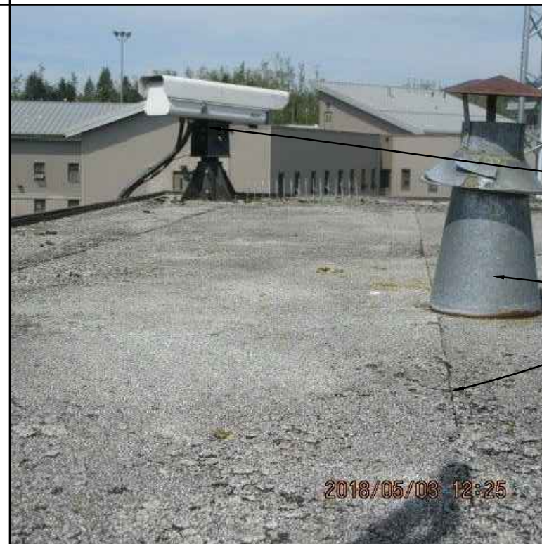
12 PHOTO OF EXISTING CONDITION
