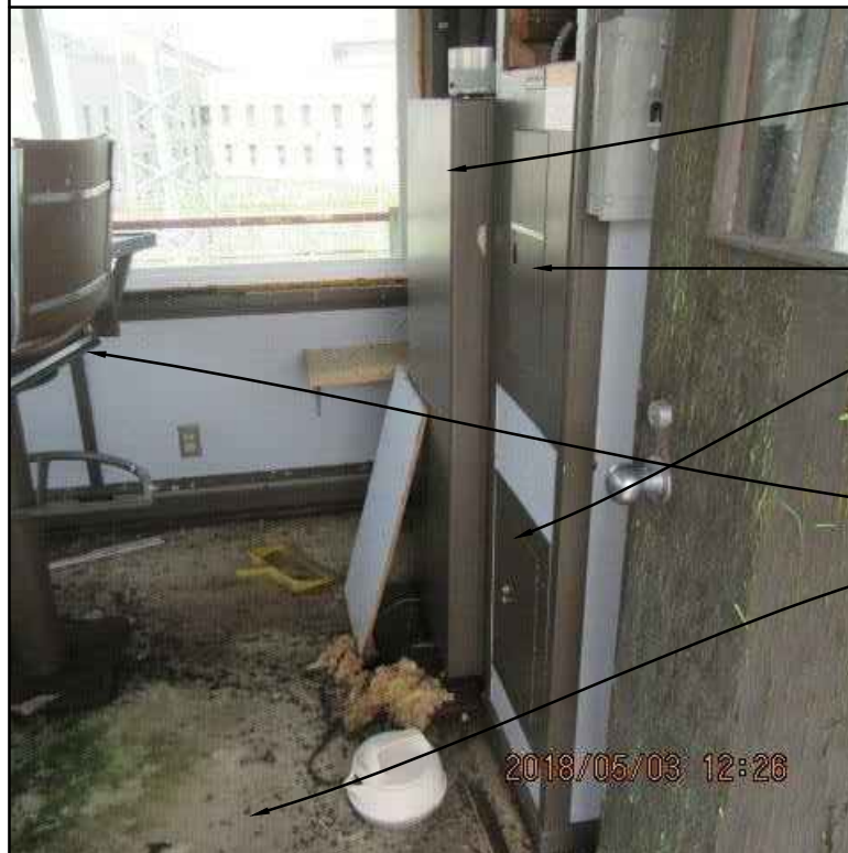
11 PHOTO OF EXISTING CONDITION
