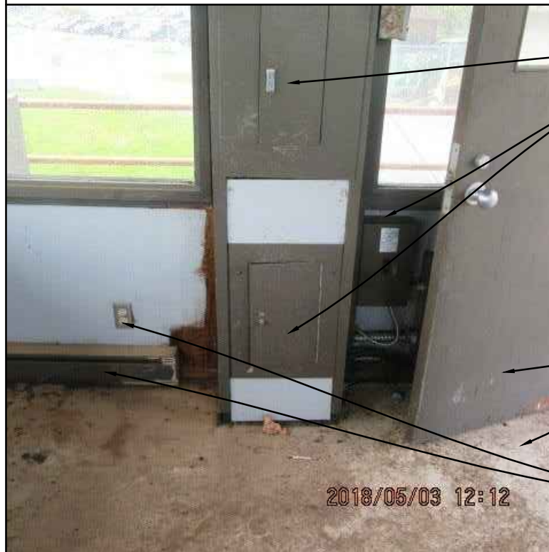
7 PHOTO OF EXISTING CONDITION
