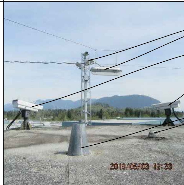
4 PHOTO OF EXISTING CONDITION
