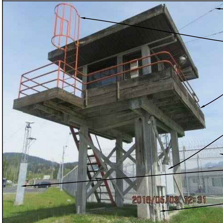
1 PHOTO OF EXISTING CONDITION
