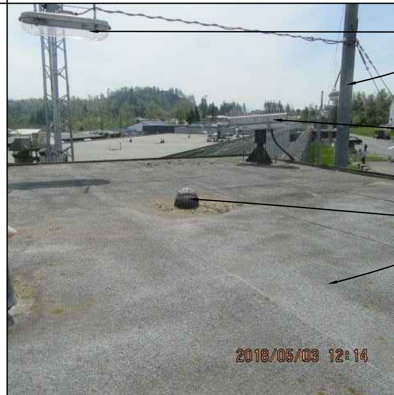
8 PHOTO OF EXISTING CONDITION
