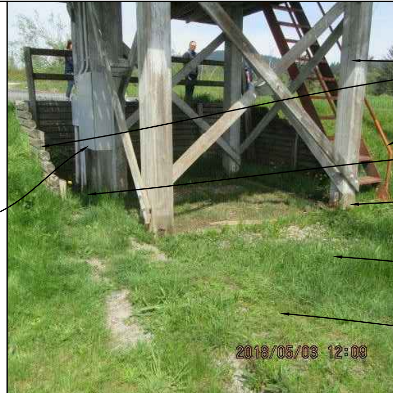
6 PHOTO OF EXISTING CONDITION
