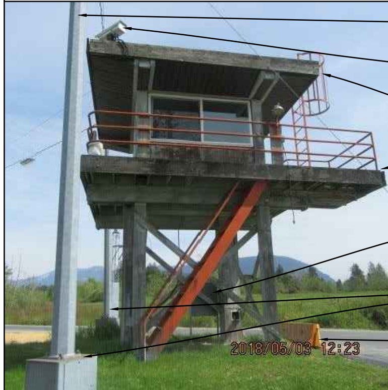
9 PHOTO OF EXISTING CONDITION
