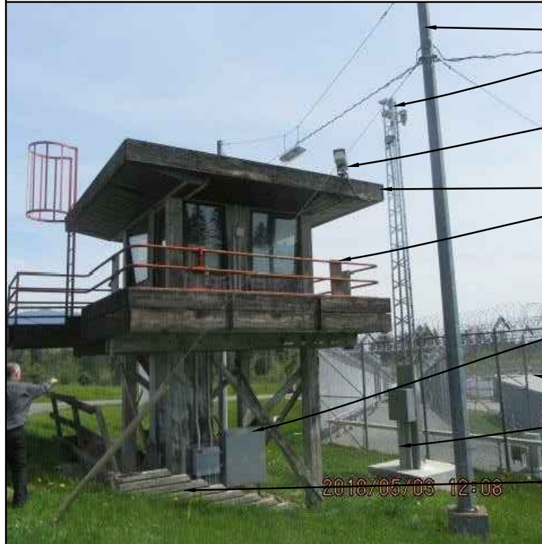
5 PHOTO OF EXISTING CONDITION
